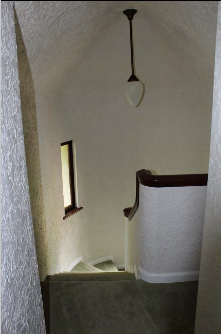
16 of 36. Stairs to second story. Camera facing north.
