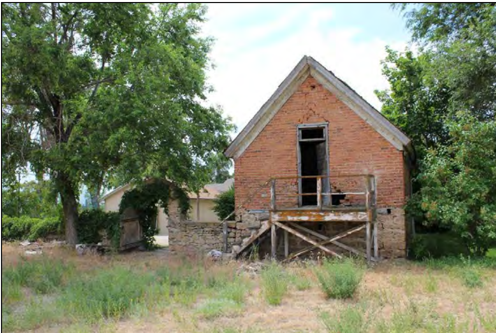
20 of 36. Outbuilding 1 (creamery/granary). Camera facing south.
