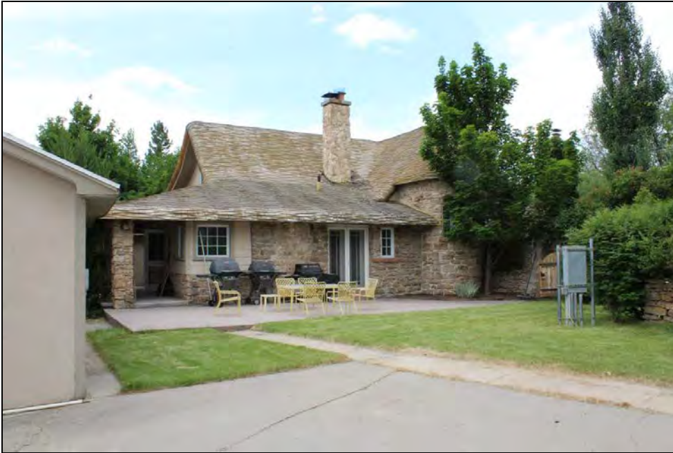
7 of 36. North and east elevation. Camera facing southwest.
