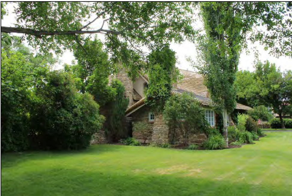
8 of 36. North and west elevations. Camera facing southeast.
