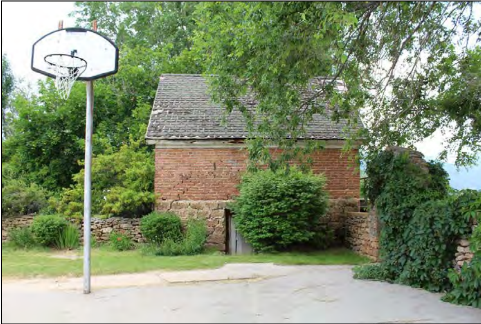
23 of 36. Outbuilding 1 (creamery/granary). Camera facing west.
