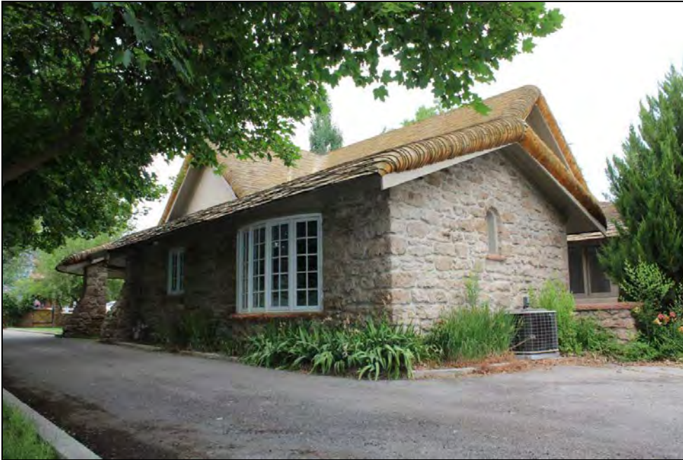
5 of 36. South and east elevations. Camera facing northwest.
