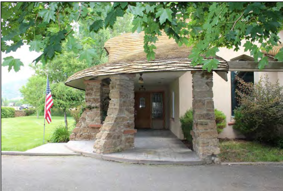
4 of 36. South elevation. Camera facing north.
