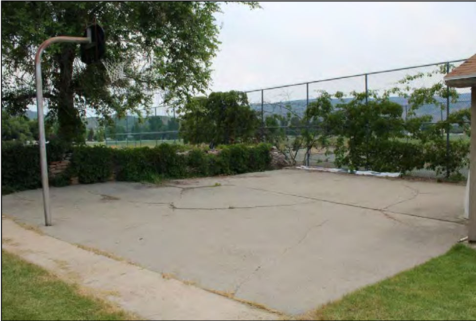
35 of 36. Structure 2 (basketball court). Camera facing northeast.
