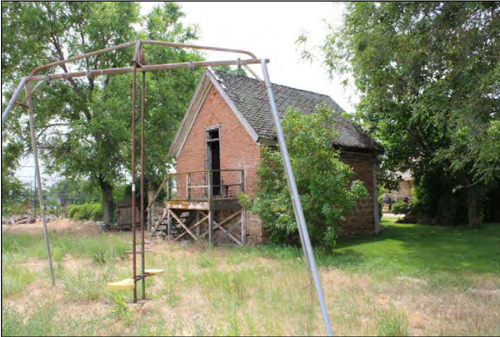
21 of 36. Outbuilding 1 (creamery/granary). Camera facing southeast.
