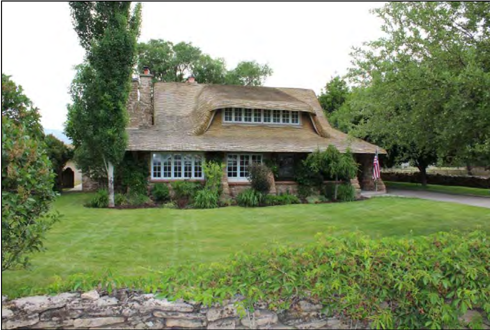
1 of 36. West elevation. Camera facing east.
