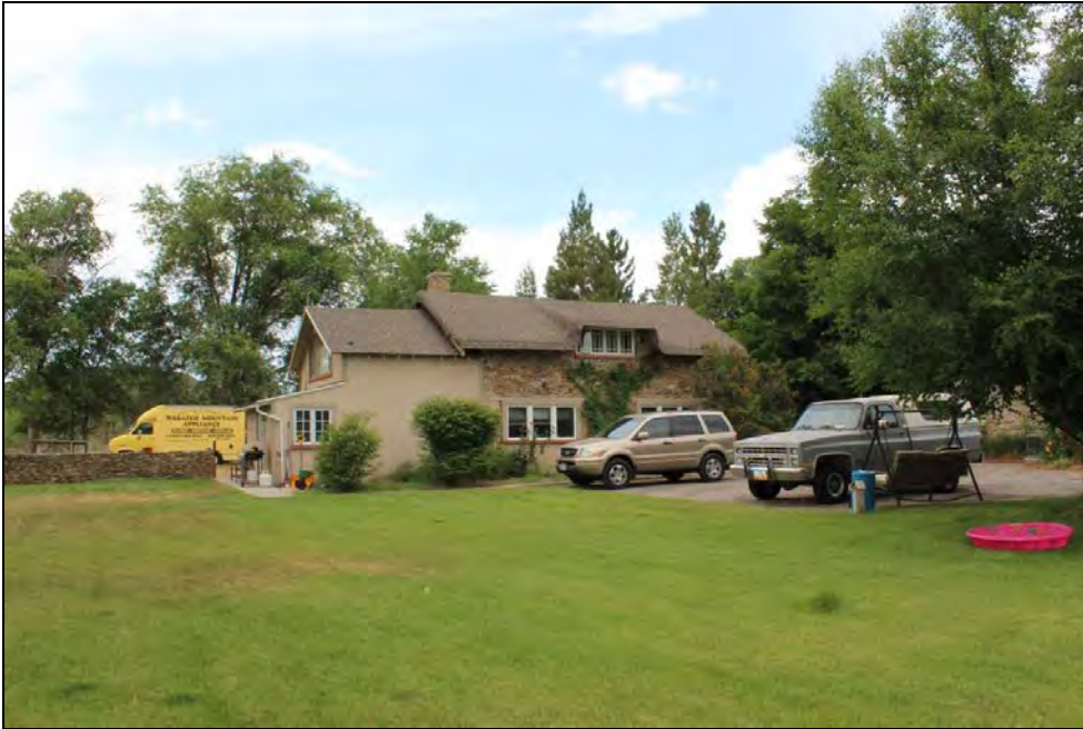
27 of 36. Outbuilding 3 (original garage). Camera facing south.
