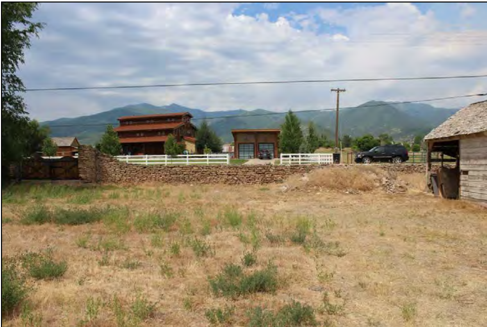
26 of 36. Outbuilding 2 (horse barn and shed). Camera facing west. Note missing section of building to the south of the remaining building
