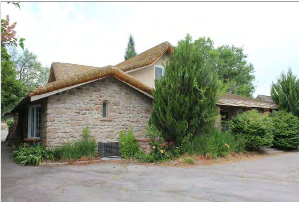
6 of 36. East and south elevations. Camera facing west.
