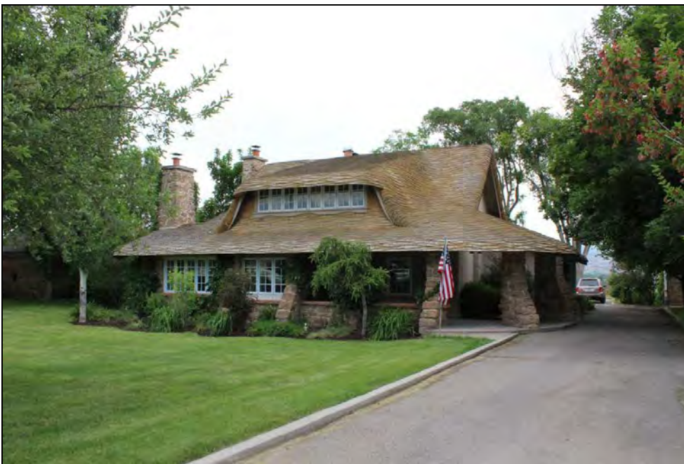
2 of 36. West and south elevations. Camera facing east.
