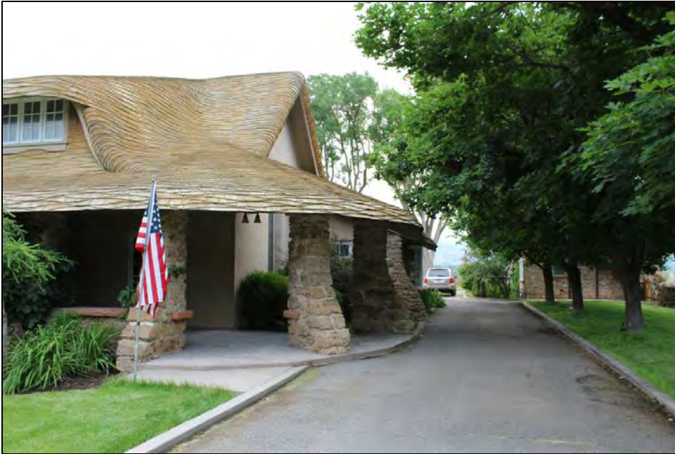
3 of 36. West and south elevations. Camera facing east.
