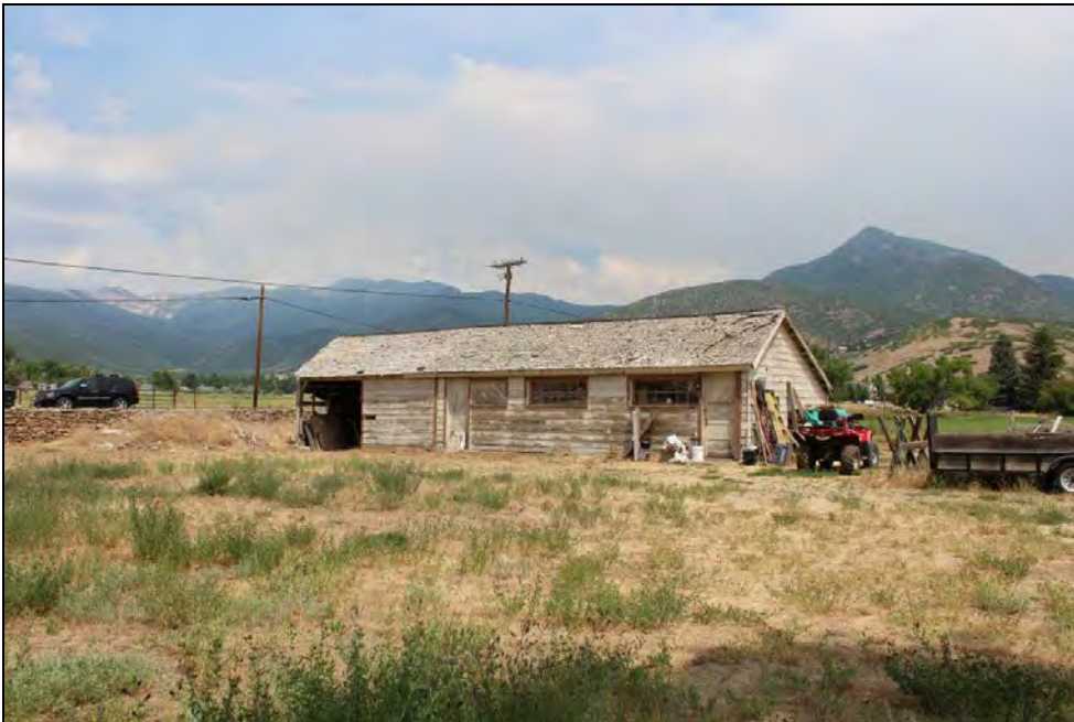
24 of 36. Outbuilding 2 (horse barn and shed). Camera facing north.
