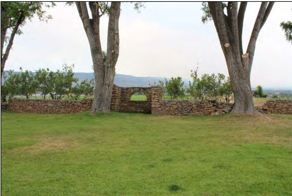
30 of 36. Structure 1 (stone wall). Camera facing east.
