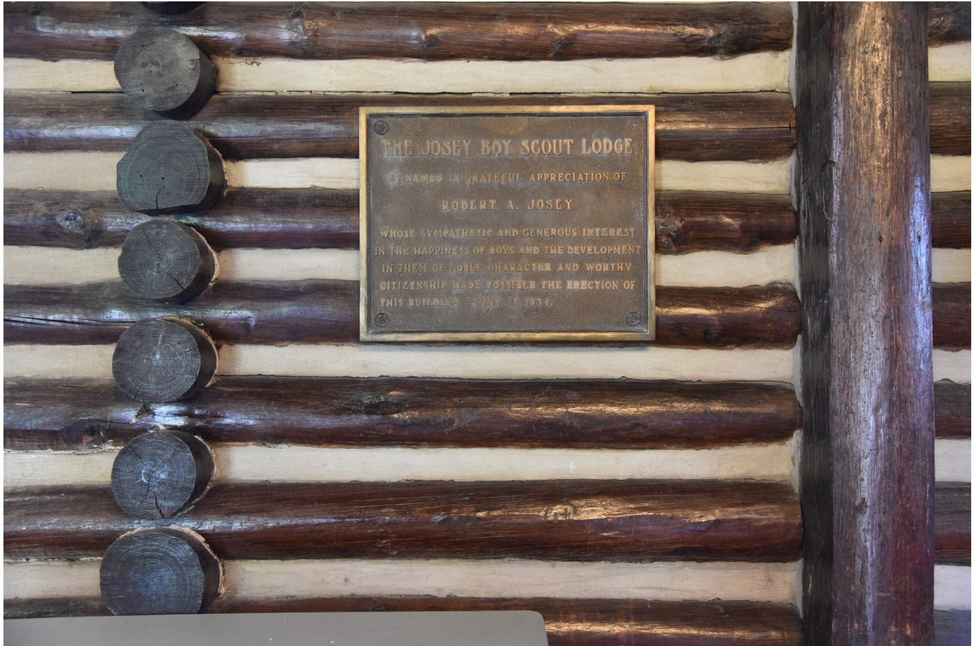
Photo 9: Dedication plaque and detail view of structural log construction and daubing, camera faces west— June 6, 2017.
