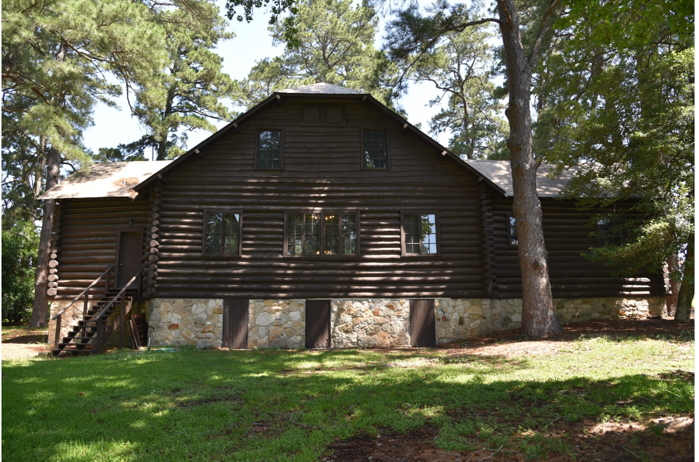
Photo 6: South elevation, camera faces north—June 6, 2017.
