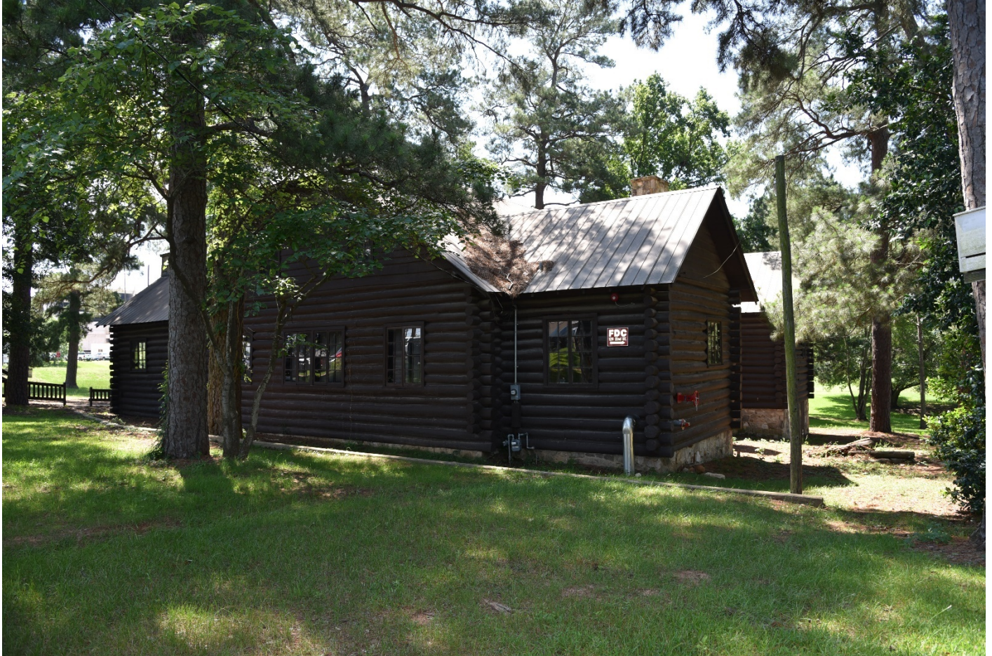
Photo 4: North and partial west (rear) elevation, camera faces southeast—June 6, 2017.
