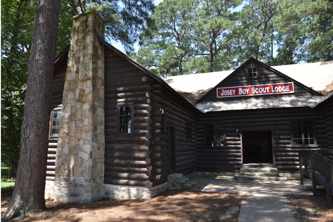
Photo 2: South wing and entrance at front (east) elevation, camera faces west—June 6, 2017. Interlocking half-round notches connect the log corners.
