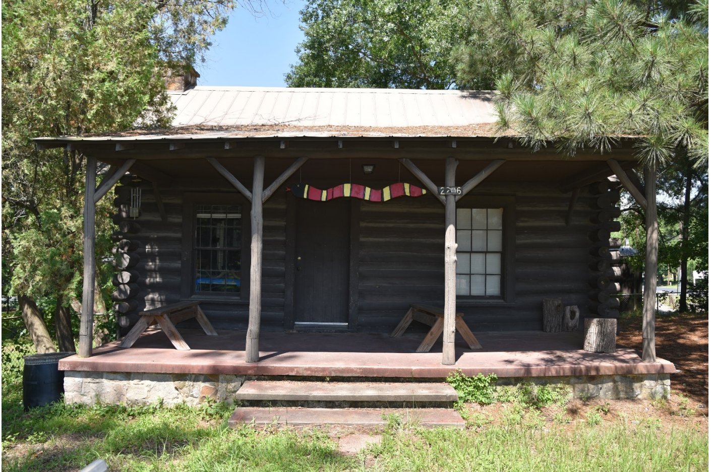
Photo 17: 1935 Keeper's Cabin front (east) elevation, camera faces west—June 6, 2017.
