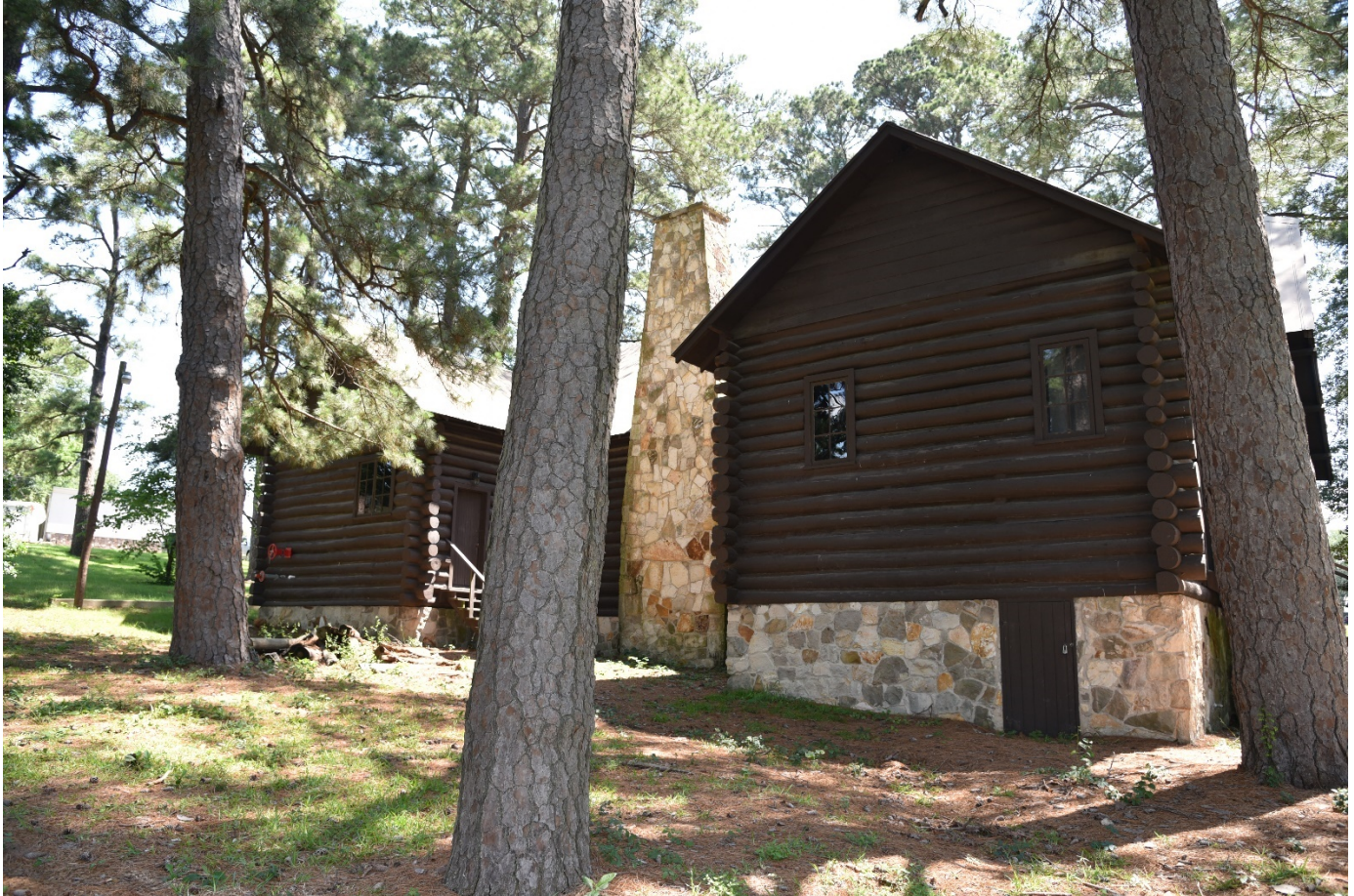
Photo 5: Southwest oblique of rear (west) elevation, camera faces northeast—June 6, 2017.
