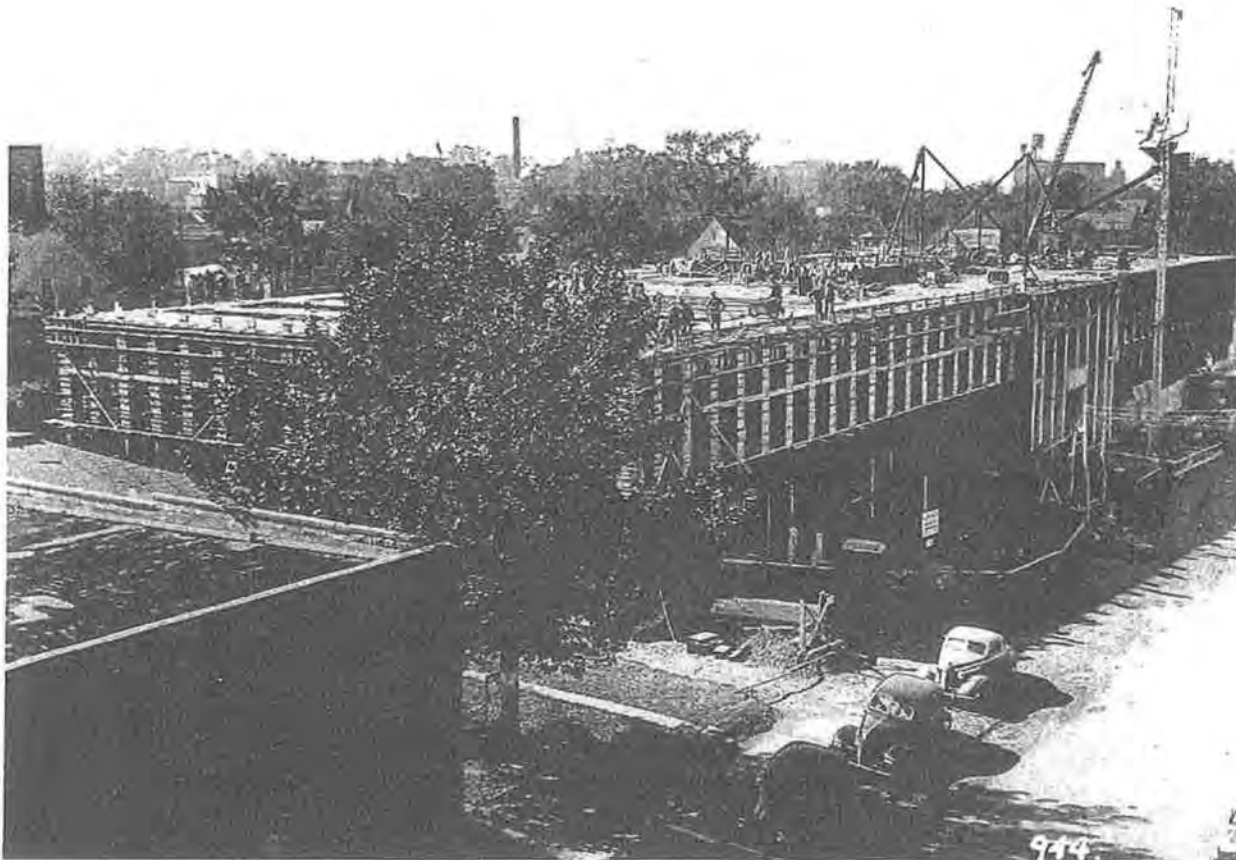
Figure 7. The 3M Administration Building under construction in 1939. (MHS photograph collection)
