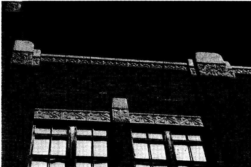
Photo 14. Office/Library/Classroom Block, South Elevation. Parapet Treatment.
