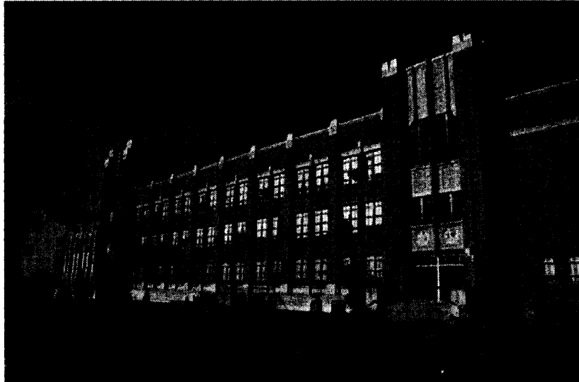
Photo 12. Office/Library/Classroom Block, South Elevation.
