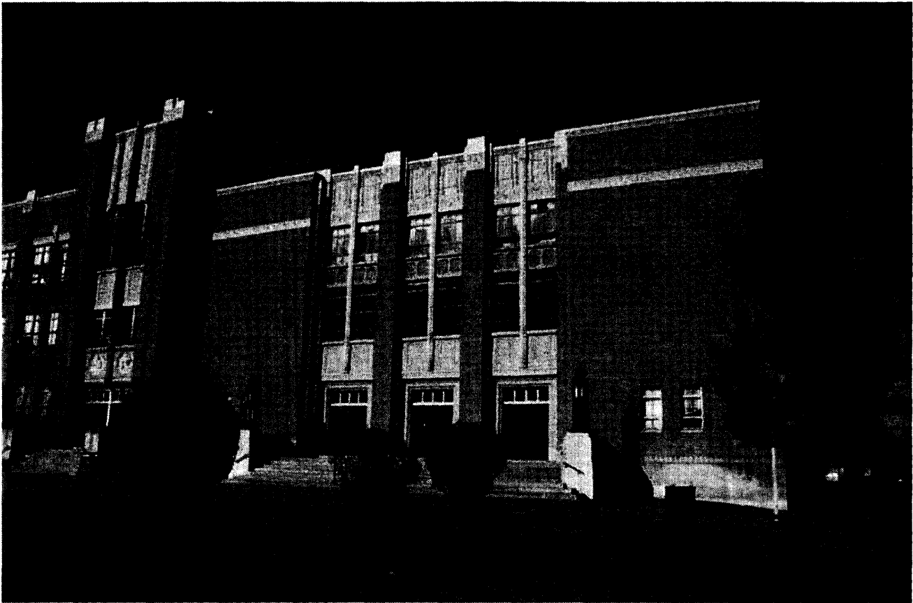
Photo 2. Auditorium Block, South Elevation.
