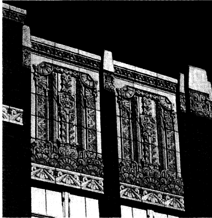
Photo 22. Gym Block, South Elevation. Panel and Parapet Detail.
