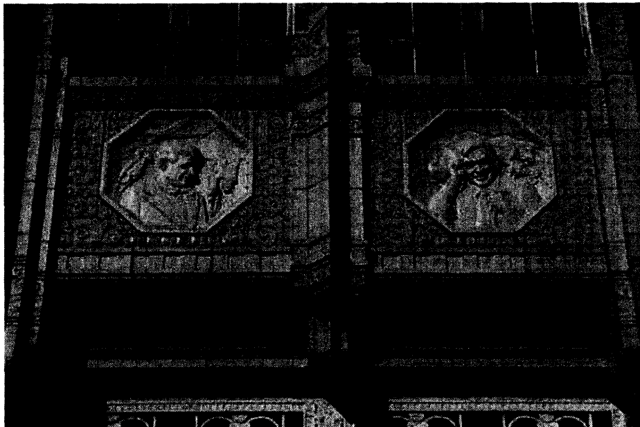
Photo 18. Main Entry Tower, South Elevation. Will Rogers Panels.
