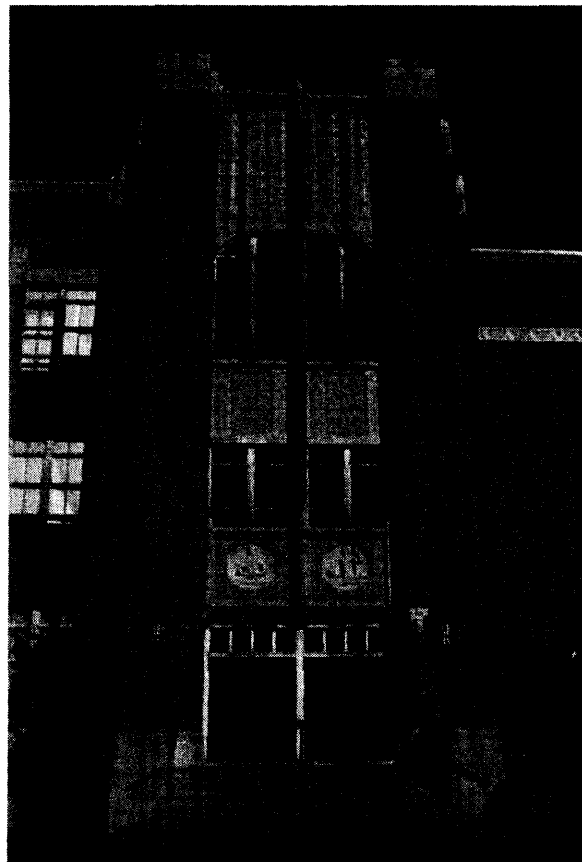
Photo 8. Secondary Tower Projection, South Elevation.
