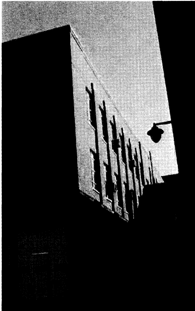
Photo 32. 1949 Classroom Wing, West Elevation.
