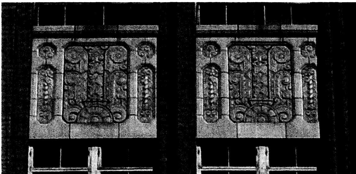
Photo 19. Main Entry Tower, South Elevation. Crop Main Entrance Bas Relief Spandrels.
