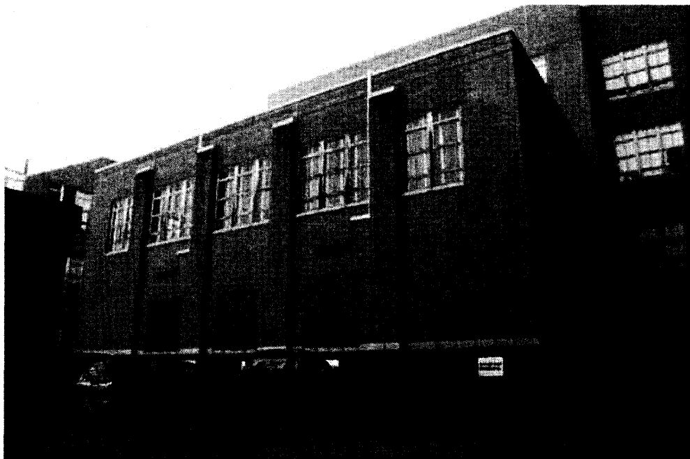
Photo 40. Library/Swimming Pool, North and East Elevation.
