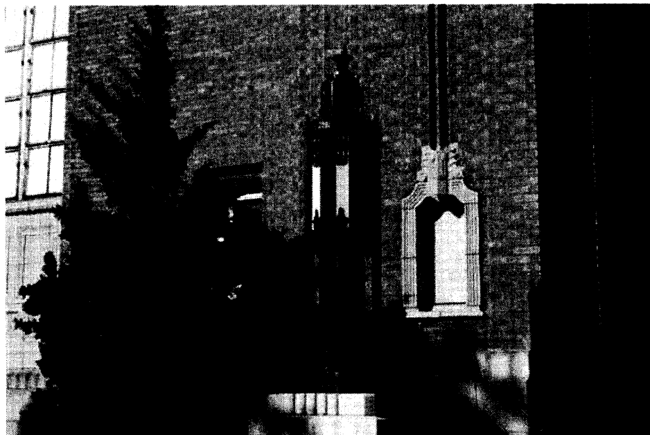
Photo 16. Main Entry Tower, South Elevation. Detail of Window, and Trim and Lanterns.
