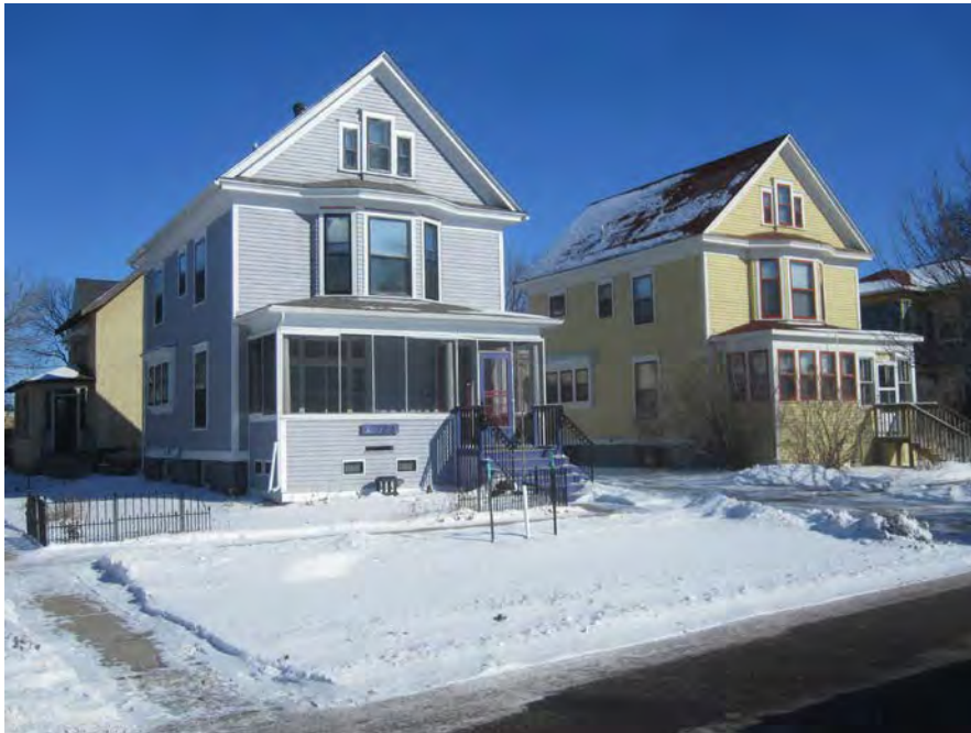
Fig. 10: Twin residences at 719 (right) and 723 (left) Third Avenue North, Fargo, ND. M. E. Beebe, architect; 1903. View from the southwest. [Photo taken by the author February 2015]
