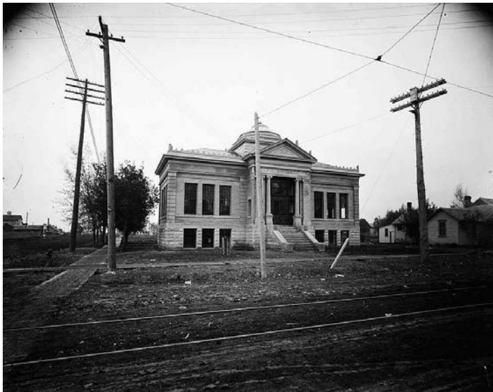
Fig. 25: Carnegie Library, Moorhead, MN. M. E. Beebe, architect; 1906. [Photo from: http://larl.org/about/history/ ]
