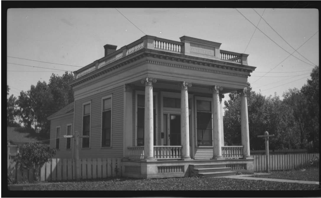
Fig. 6: M. E. Beebe Architectural Office, 717 Third Avenue North, Fargo, ND. M. E. Beebe, architect; 1906. View from the southwest. The wing extending behind the office may have been a small residence that once faced onto North Eighth Street; to make room for his own house of 1905, he seems to have relocated and rotated it 180° and incorporated it with the new construction of 1906. [Photo from: the Institute for Regional Studies, NDSU (ref. #007879)]
