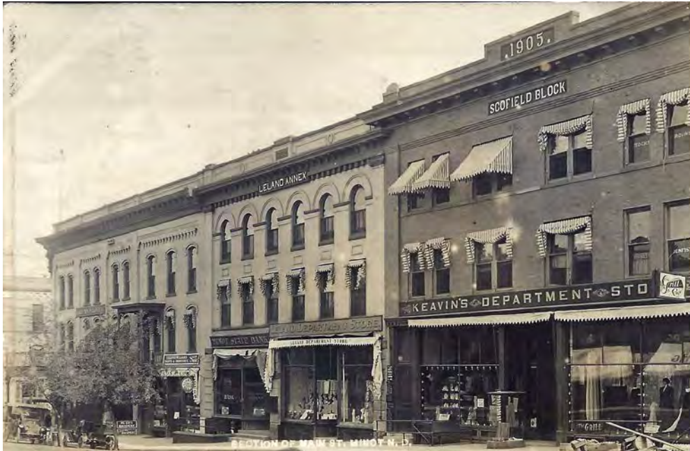
Fig. 23: Leland Hotel Annex, Minot, ND. M. E. Beebe, architect; 1902. [Photo from a postcard in the author's collection]
