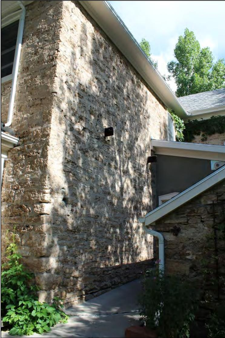
3 of 16. East elevation. Camera facing northwest. Note beams extending from wall, which may have provided a place for a porch to be attached.
