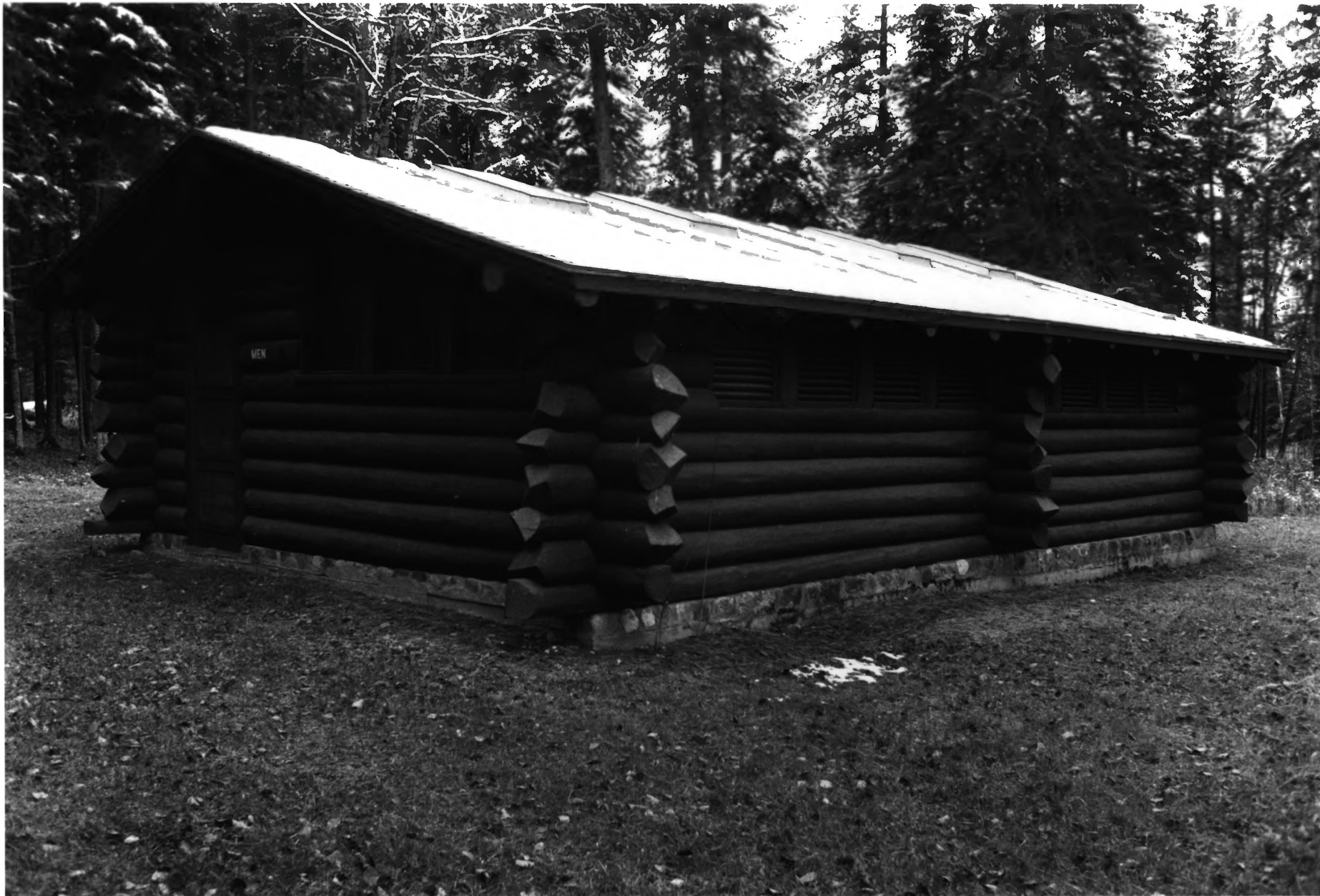
SCENIC STATE PARK - CCC / RUSTIC STYLE HISTORIC DISTRICT ITASCA CO., MN PHOTO I.D. # 09120 # 21 BLDG # 3
