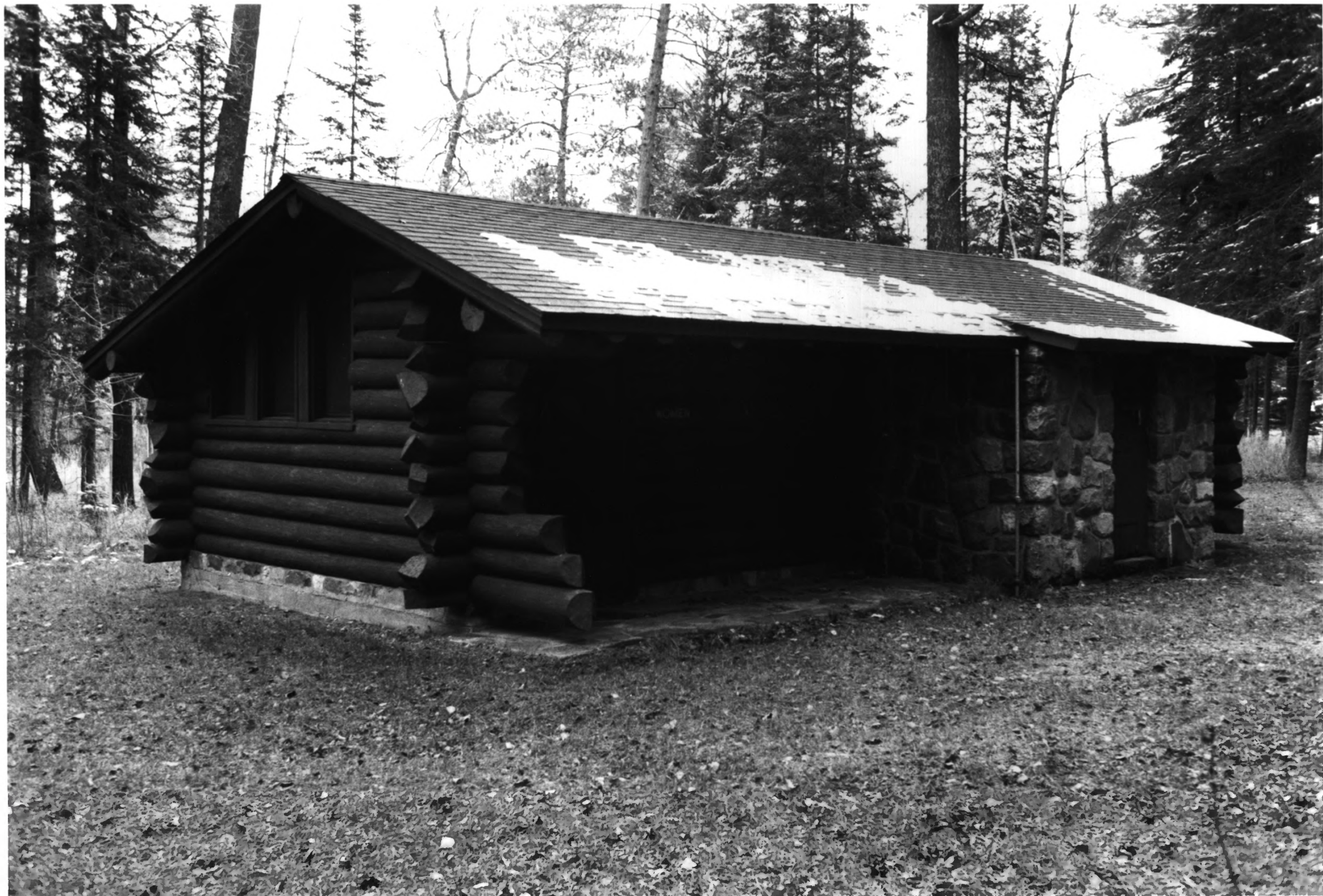
SCENIC STATE PARK-CCC/RUSTIC STYLE HISTORIC DISTRICT ITASCA CO., MN PHOTO I.D. # 09120 # 20 BLDG # 3
