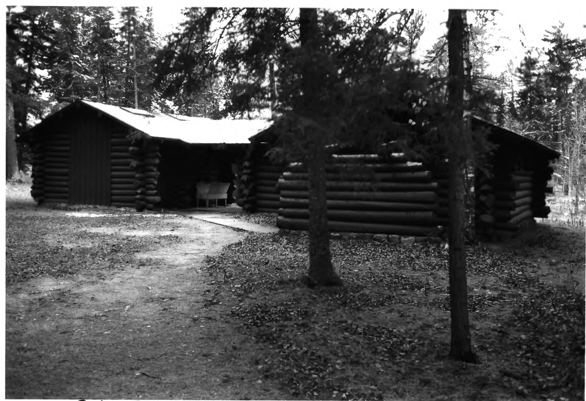
SCENIC STATE PARK - CCC/RUSTIC STYLE HISTORIC DISTRICT ITASCA CO. MN BLDG # 4 PHOTO I.D. 09399 #3
