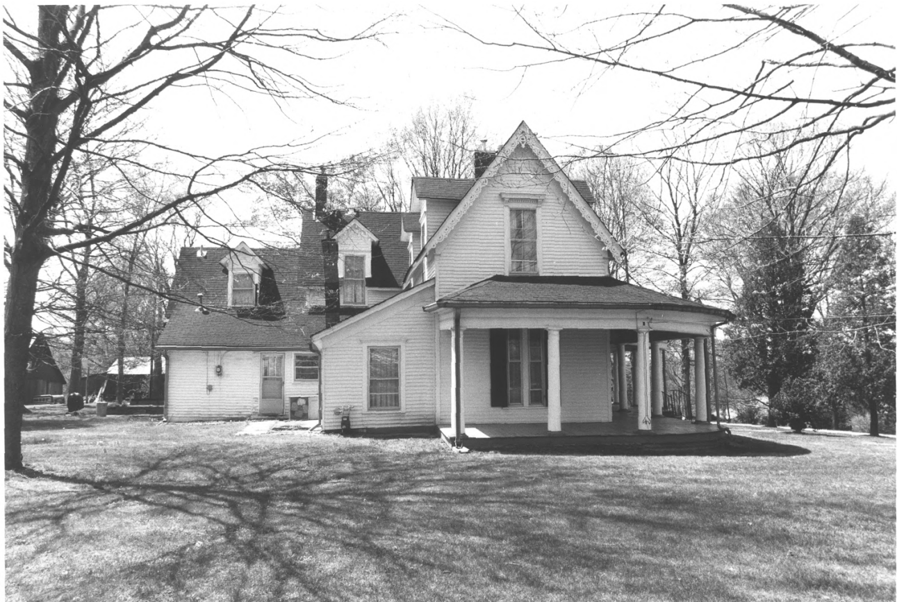
Edward S. Ferrill House, LU-49 Larue County, MRA
