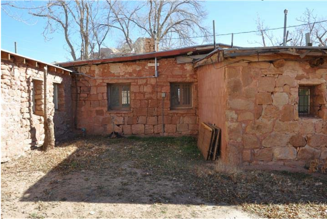
25 of 50. West elevation of mission house center section. Camera facing east.
