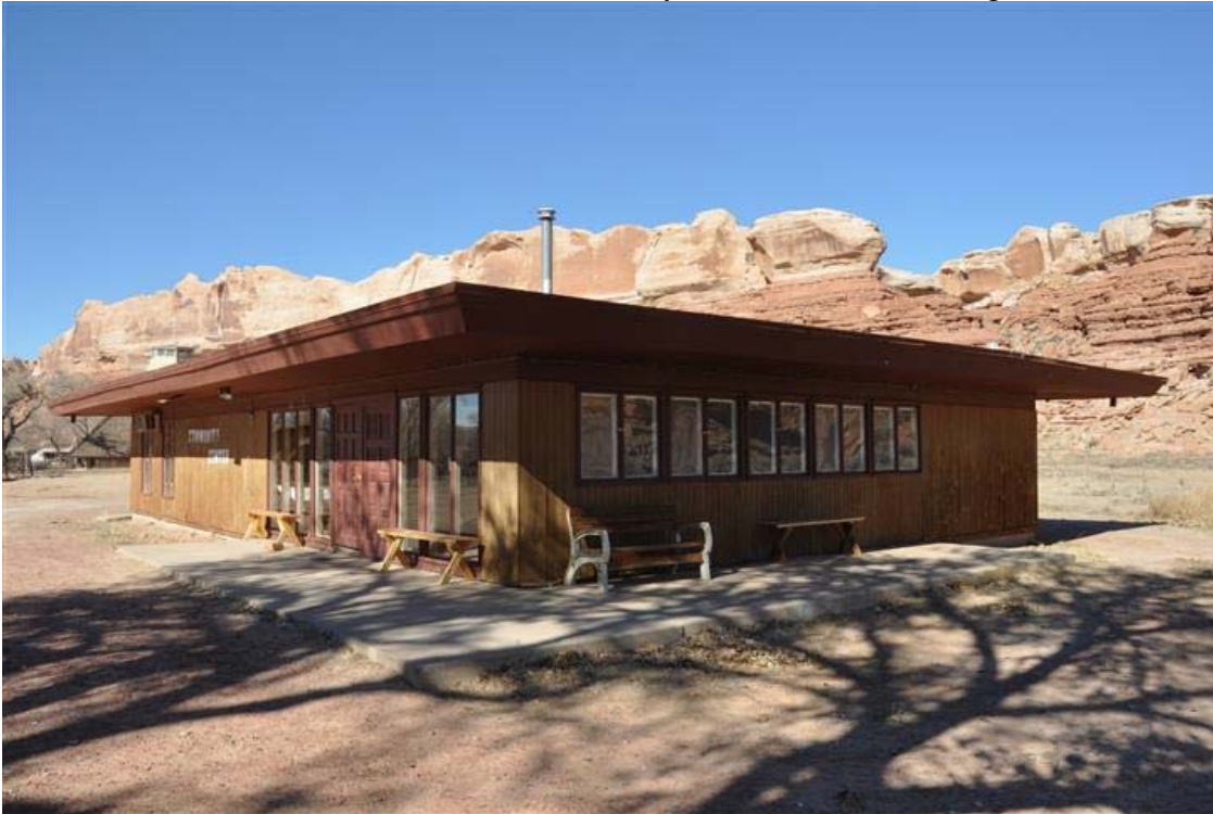
40 of 50. South and east elevations of community center. Camera facing northwest.
