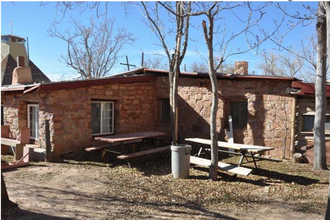
30 of 50. North & east elevations of mission house mid-section. Camera facing southwest.
