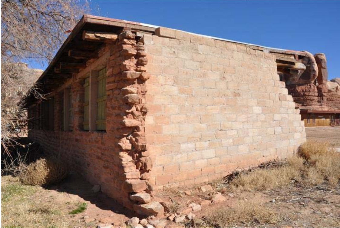
37 of 50. South and west elevations staff housing. Camera facing northwest .
