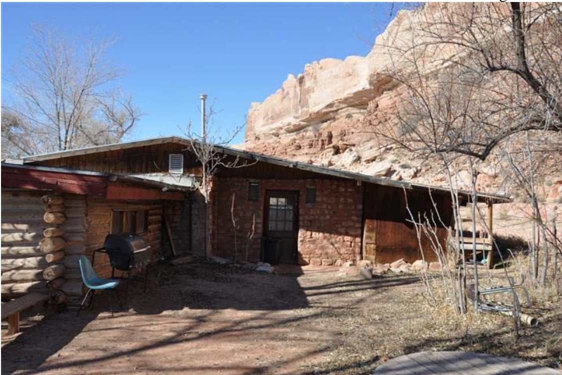
28 of 50. East and north elevations of mission house rear section. Camera facing west.
