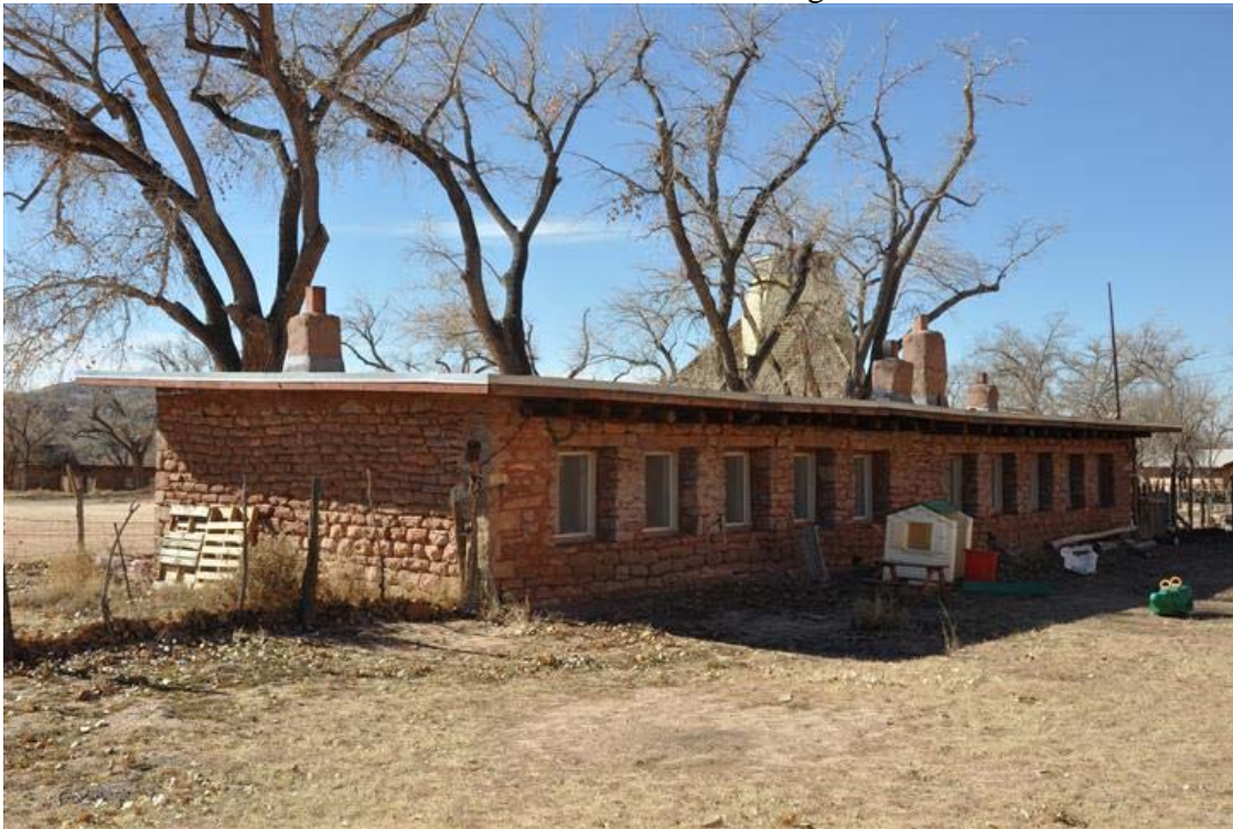
35 of 50. North and east elevation of school. Camera facing southwest.
