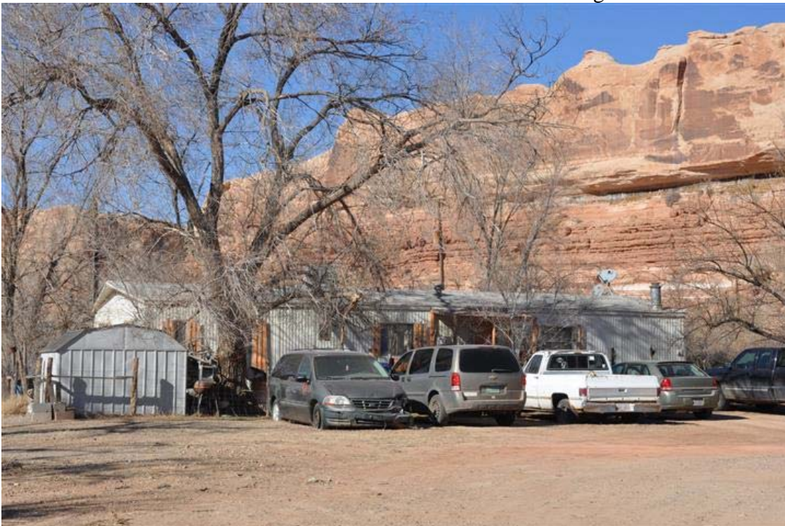
41 of 50. South and east elevations of mobile home. Camera facing northwest.
