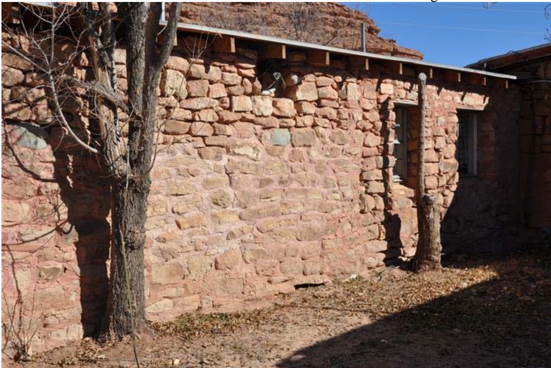
24 of 50. South elevation of mission house rear section. Camera facing northeast.
