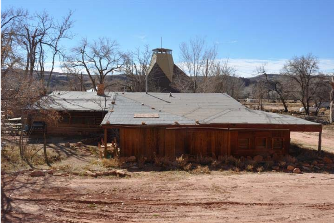
27 of 50. North elevation of main mission house. Camera facing south.
