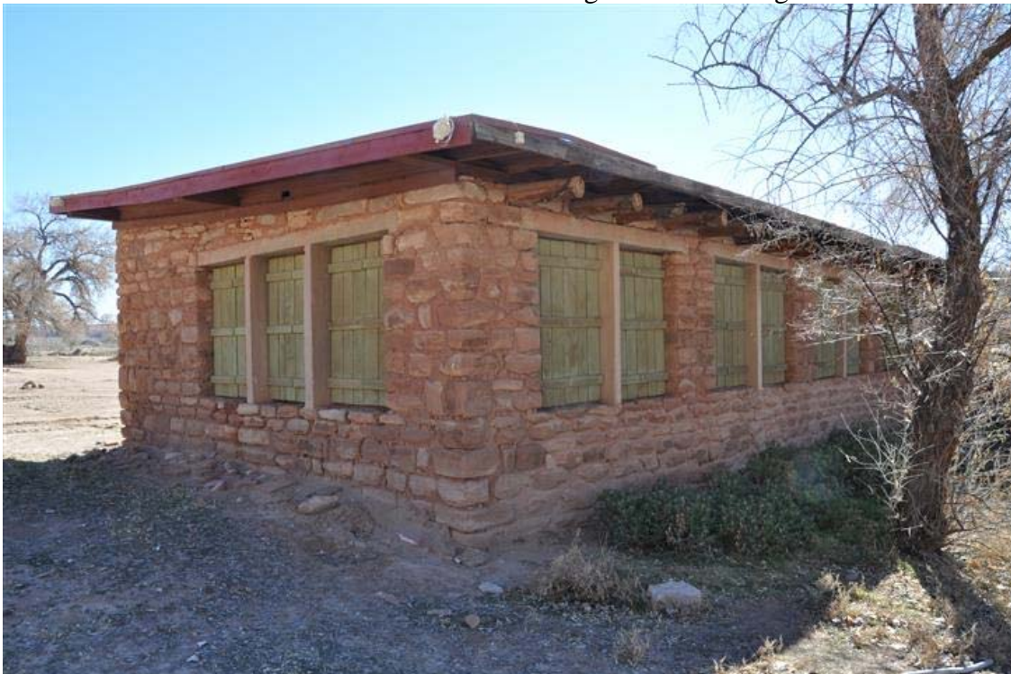
38 of 50. North and west elevations of staff housing. Camera facing southeast.
