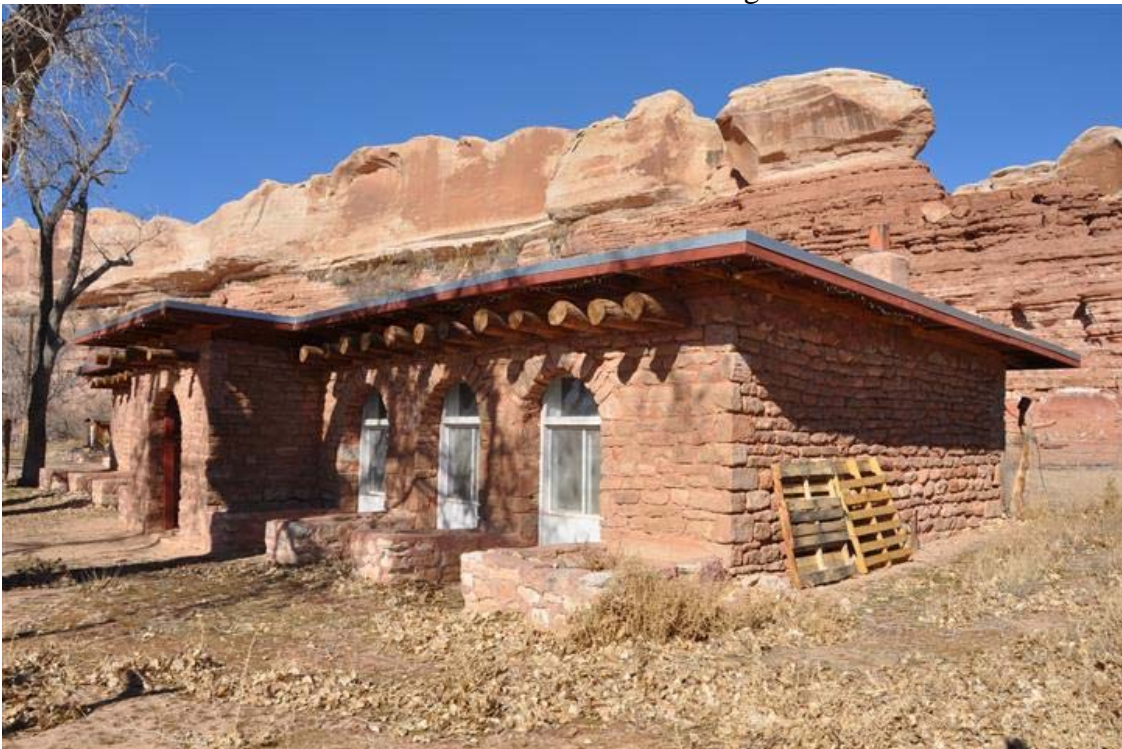
34 of 50. South and east elevations of school. Camera facing northwest.
