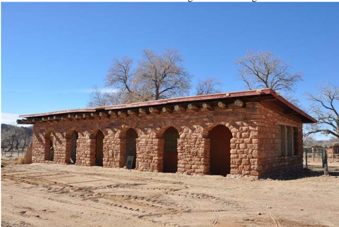
36 of 50. North and east elevation of staff housing. Camera facing southwest.
