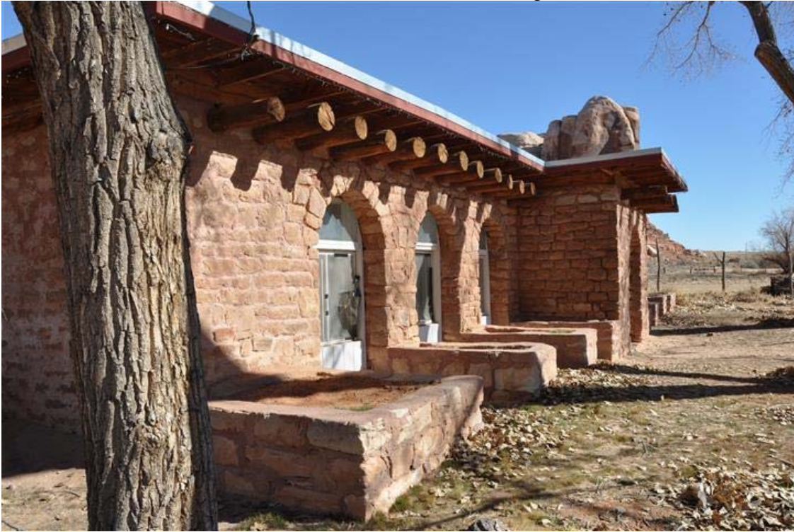
33 of 50. South and west elevations of school. Camera facing northeast.
