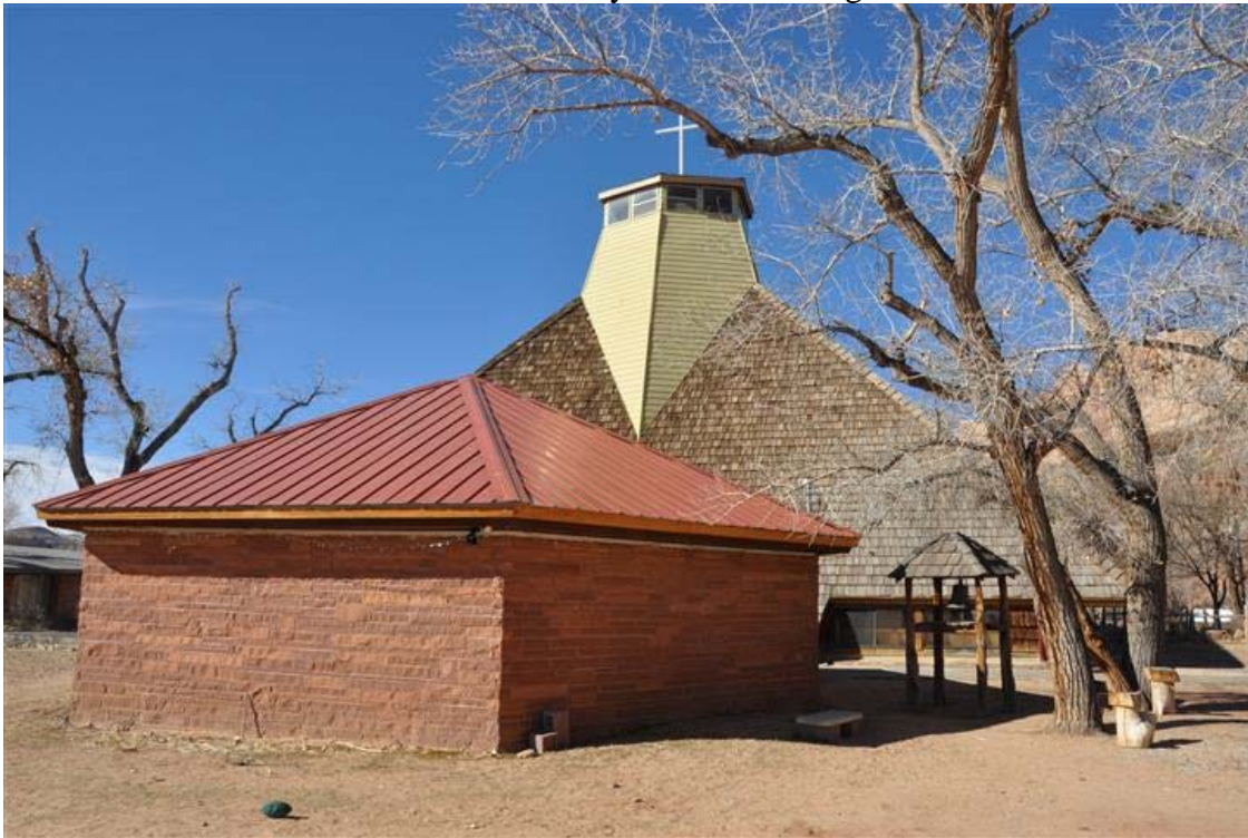
16 of 50. North and east elevations of sacristy. Camera facing southwest.
