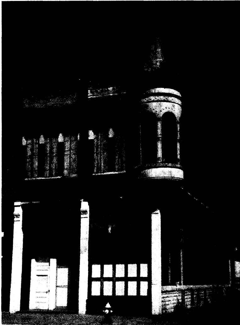
Figure 1: Insurance Building (c. 2005) west façade, south elevation
