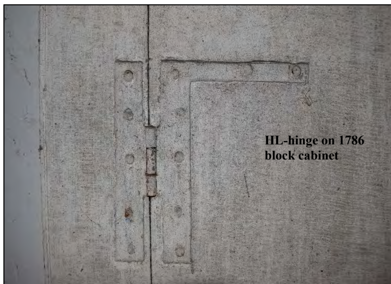
Figure 2: HL-Hinge, 1786 Block Cabinet
