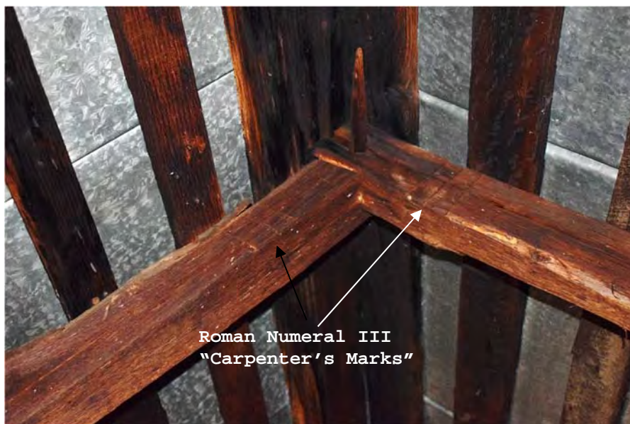
Figure 3: Attic Carpenter's Marks
