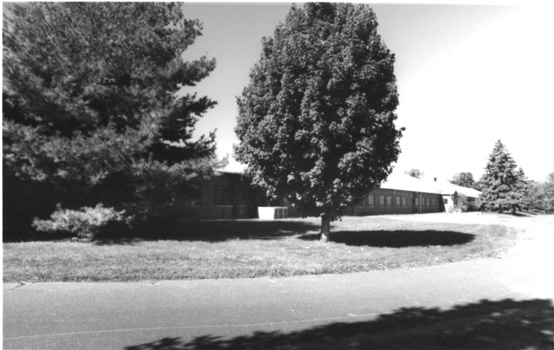
Front of 9010 looking east / Camp Evans Historic District / Monmouth Co., NJ / photo 11 of 20
