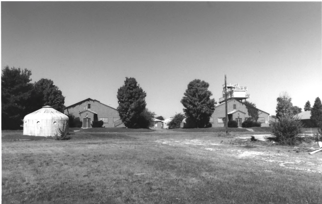
East view of 9076-9037 / Camp Evans Historic District / Monmouth Co., NJ / photo 12 of 20
