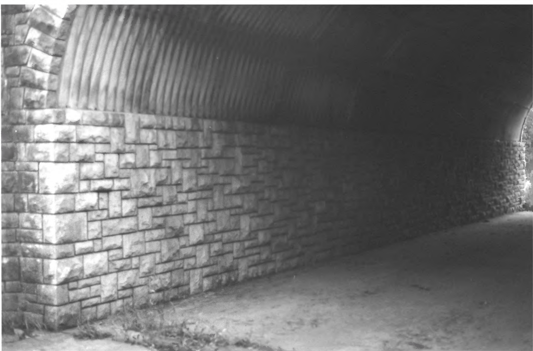
Bridge no. 5827 Mn Highway 60, Zumbro Falls Wabasha Co., Mn 013098-5A16
