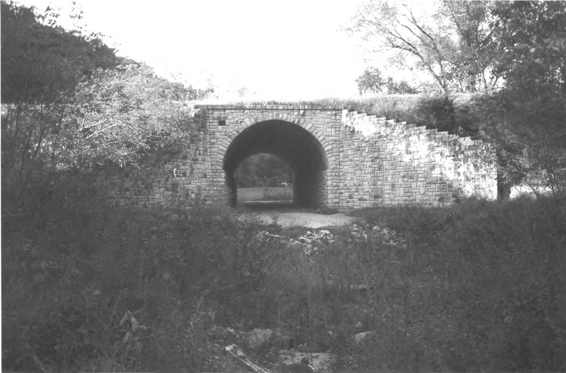
Bridge no. 5827 Mn Highway 60, Zumbro Falls Wabasha Co., Mn O 13098-6A17
