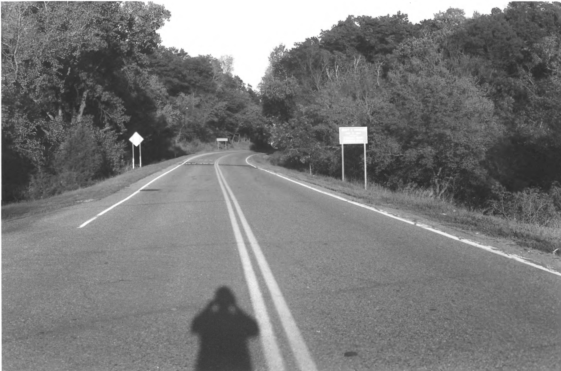
Bridge no. 5827 Mn Highway 60, Zumbro Falls Wabasha Co., Mn 013098-4A15
