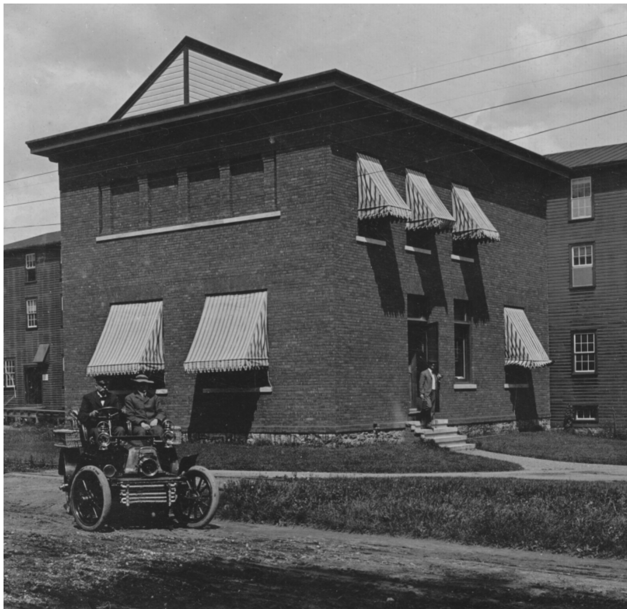
Figure 2. NR #3, Office Building, c. 1907 View toward Northeast from Water Street (Collection of the Bennington Museum, Bennington, Vermont.)
