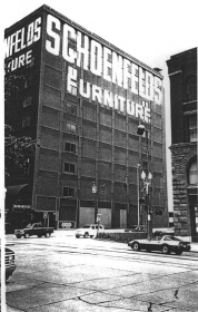
Sandberg Schoenfeld Building 1411-1423 Pacific Avenue, Tacoma August, 1998 South Elevation Angle Looking North =>
