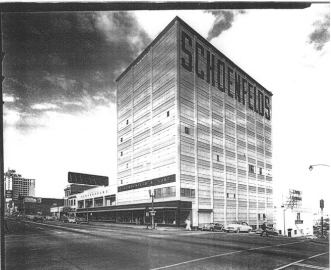
SANDERSON-GRIFFIN/PHILIP BULLFINCH, 444-443 Pacific Avenue, Toronto, O.A. Nomination to the National Register of Historic Places Historic Photograph, 119, S.W. Iron, Southwest Angle, ca. 1955
