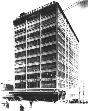
SANDBERG-SCHOENFELD BUILDING, 1411-1423 Pacific Avenue, Tacoma, WA. Nomination to the National Register of Historic Places Historic Photograph, TPL NW Room, Southwest Angle, ca. 1925
