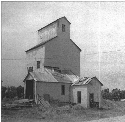
Photo 14 of 30. Grain Elevator, facing northwest.
