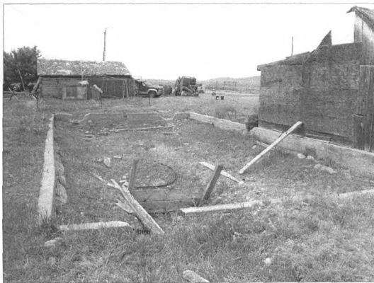
Photo 20 of 30. Non-contributing element 2 (NC2): Foundation remains, view to south.
