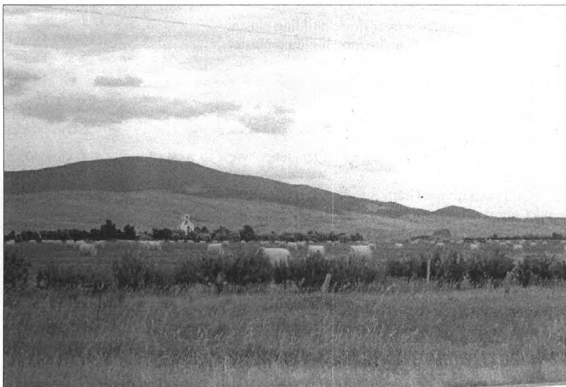
Photo 2 of 30. Overview of the historic building cluster, Naylor Brothers Ranch. Facing east from State Highway 191.
