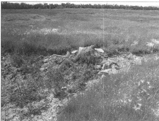
Photo 6 of 30. Dam remains, facing south.
