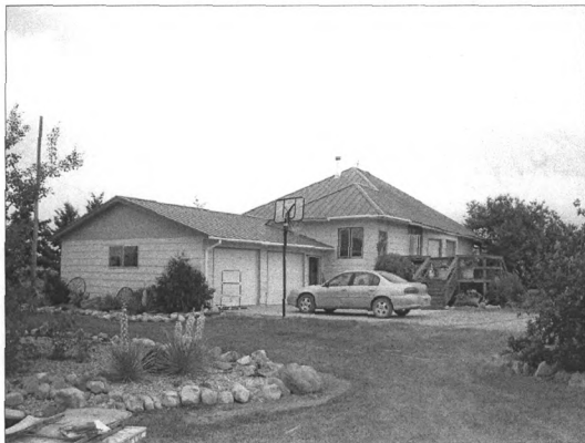
Photo 19 of 30. Non-contributing element 1 (NC1): The Main Residence, view to northeast.
