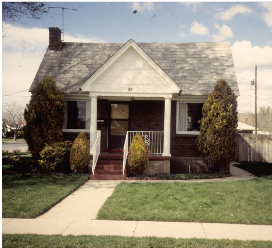
Fig. 20 of 47. South Elevation / Façade of 34 Boulevard Gardens c. 1985.
