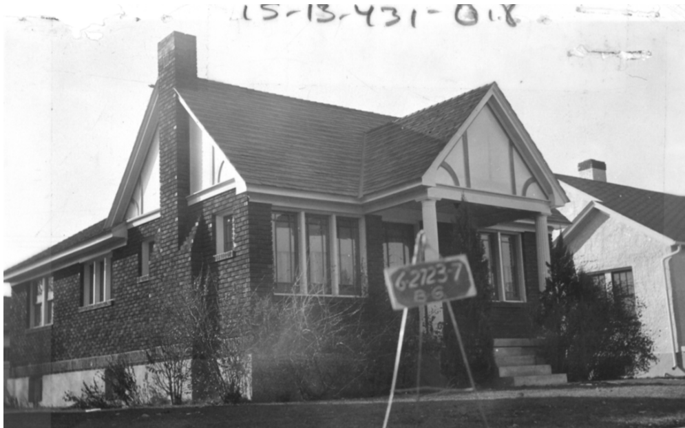
Fig. 19 of 47. South Elevation / Façade of 34 Boulevard Gardens c. 1935.
