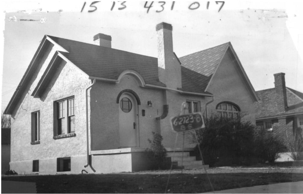
Fig. 39 of 47. East and North Elevations / Side and Façade of 57 Boulevard Gardens c. 1935.
