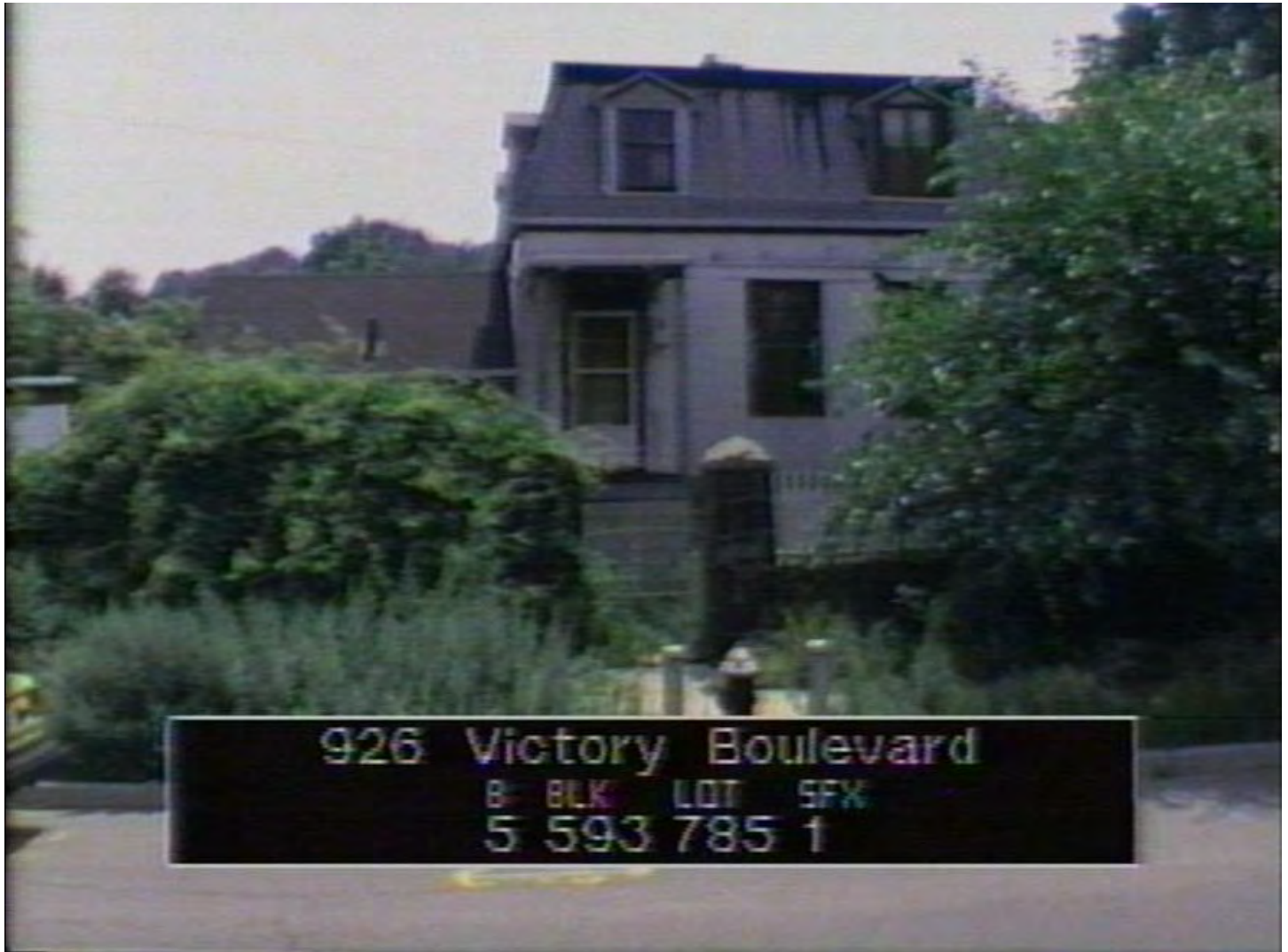
Figure 3 New York City tax photo of 926 Victory Boulevard, ca. 1983-1988, showing the former caretaker's cottage at the northwest corner of Silver Lake Cemetery. The stone wall surrounding the cemetery can be seen in the foreground.
