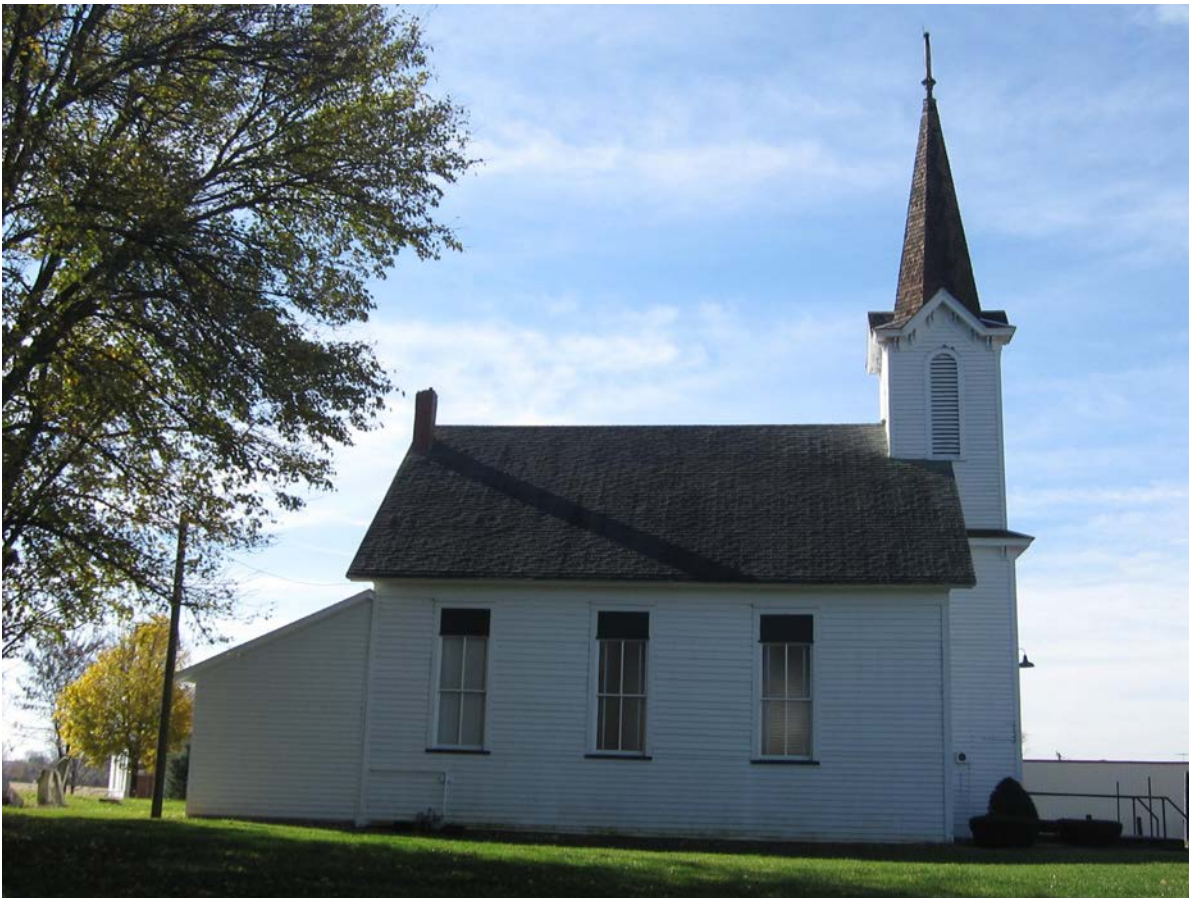
Above: Hauge Lutheran Church and the Annex read as two separate buildings.
