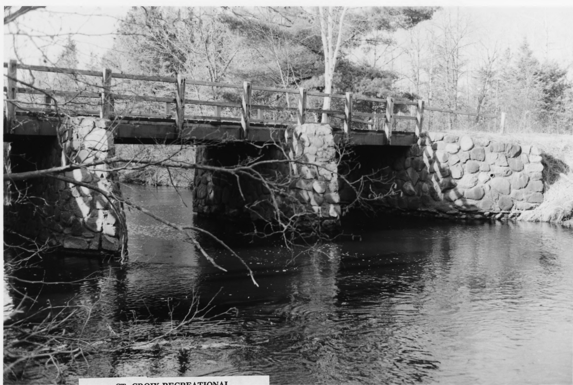
ST. CROIX RECREATIONAL DEMONSTRATION AREA Hinchley, Pine County, MN Bridge over Sand Creek Photo: Rolf Anderson, 1988
