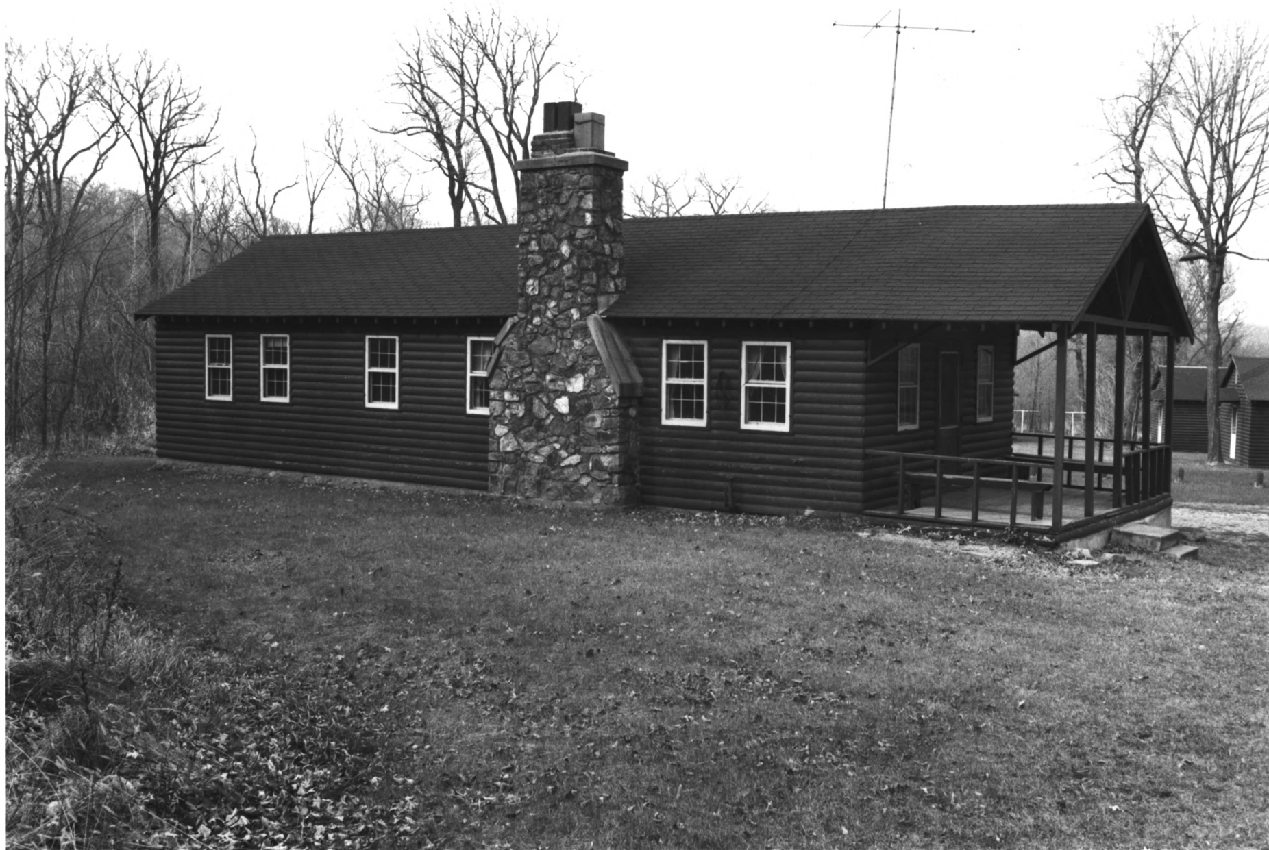
FLANDRAU STATE PARK - OFFICE / WPA CAMP BROWN CO., MN BLDG # 17 PHOTO I.D. 09118 # 14
