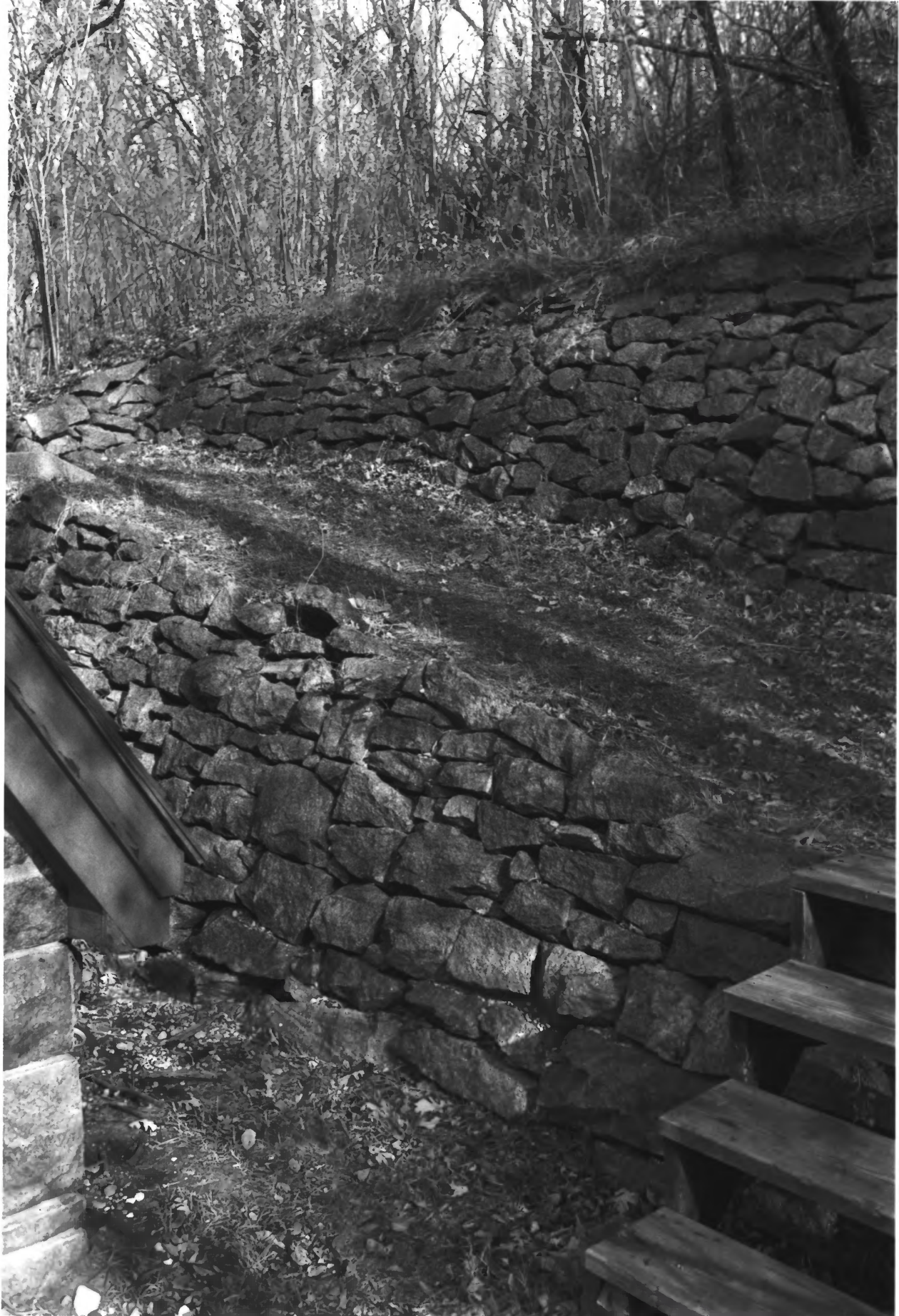
FLANDRAU STATE PARK - RETAINING WALL BROWN CO., MN STRUCTURE #11 PHOTO I.D. 09399 #14
