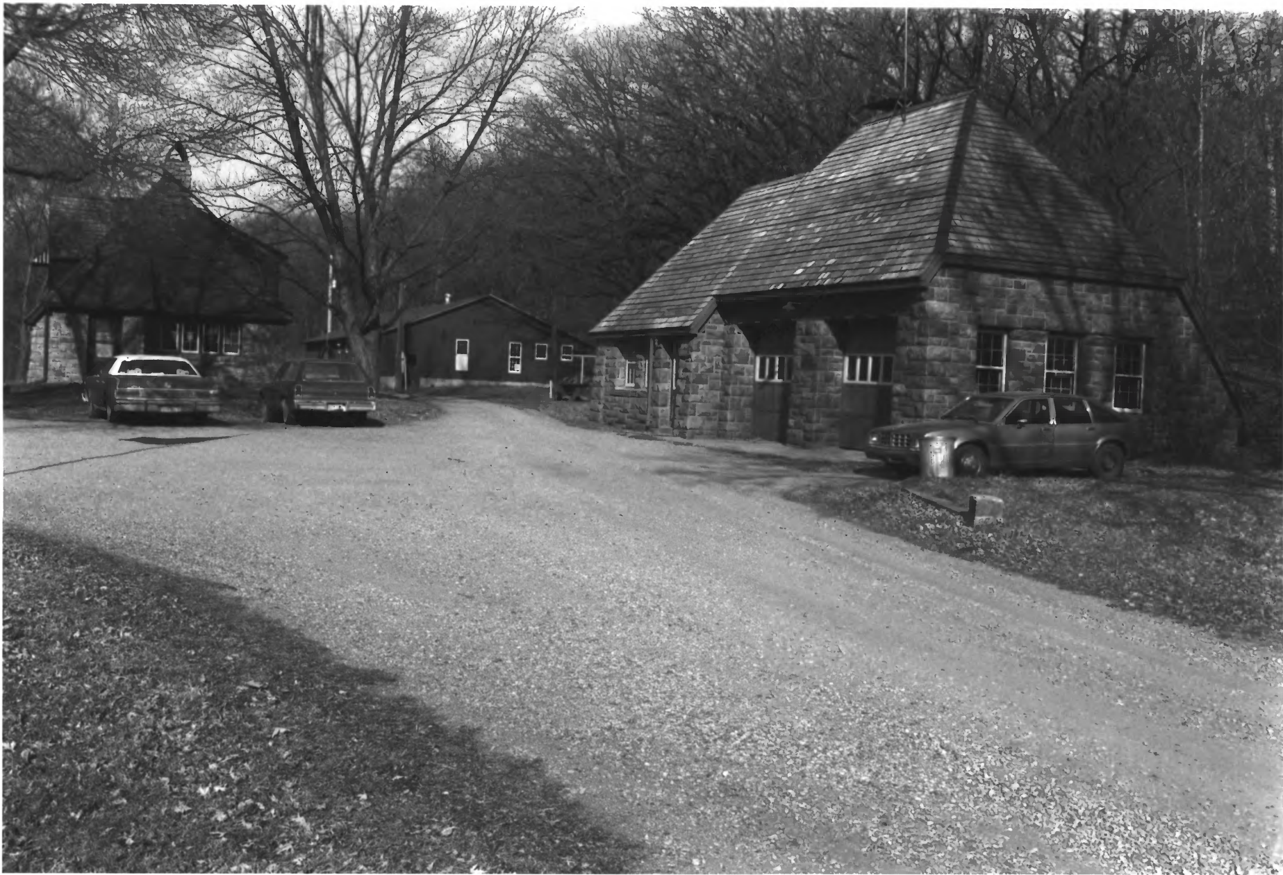
FLANDRAU STATE PARK - RESIDENCE, SHOP, GARAGE (L to R) BROWN CO. MN BLDGs # 9, 12 + 10 PHOTO I.D. 09399#19
