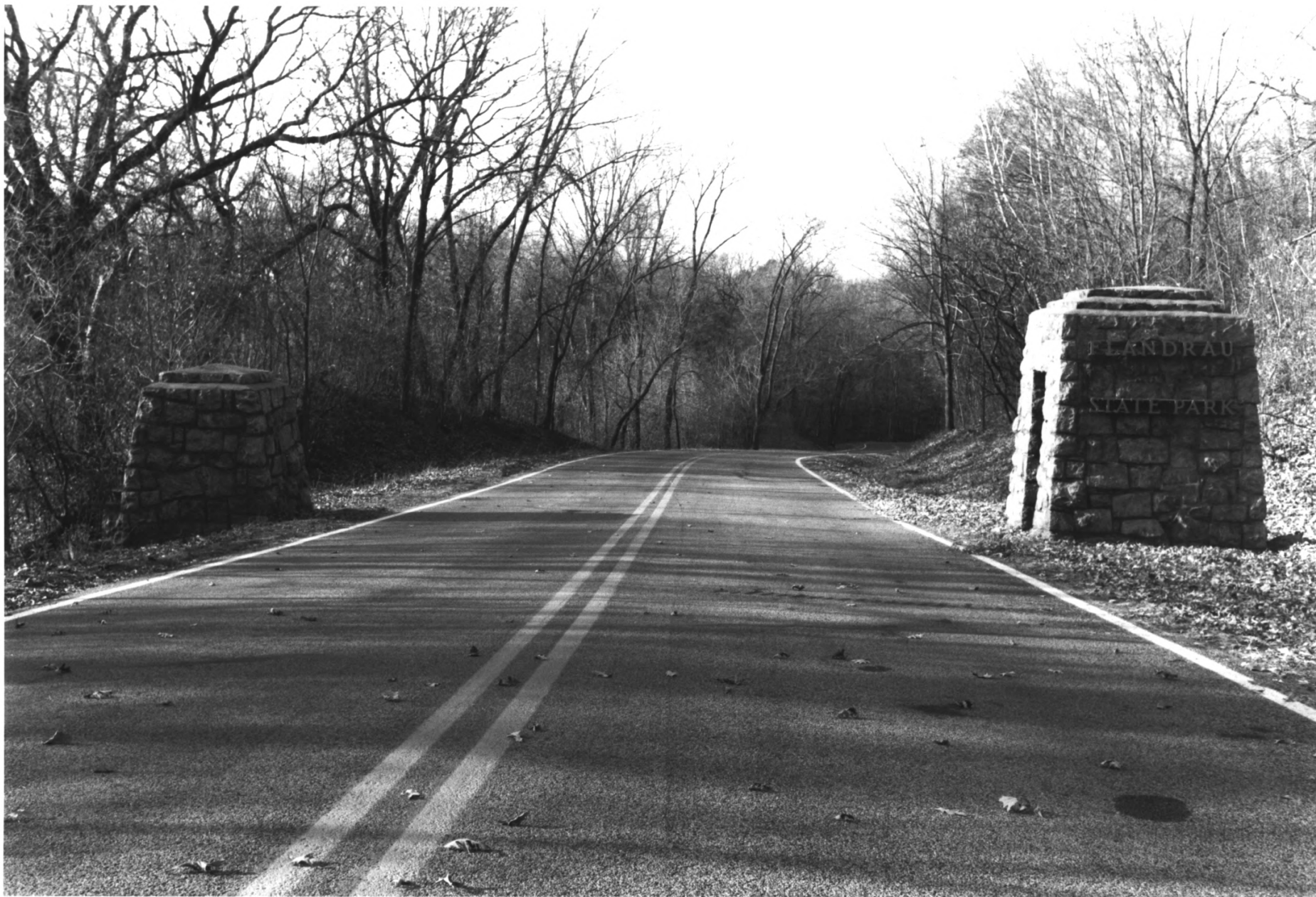
FLANDRAU STATE PARK - ENTRANCE PORTALS BROWN CO., MN OBJECT #1 PHOTO I. D. 09399#11
