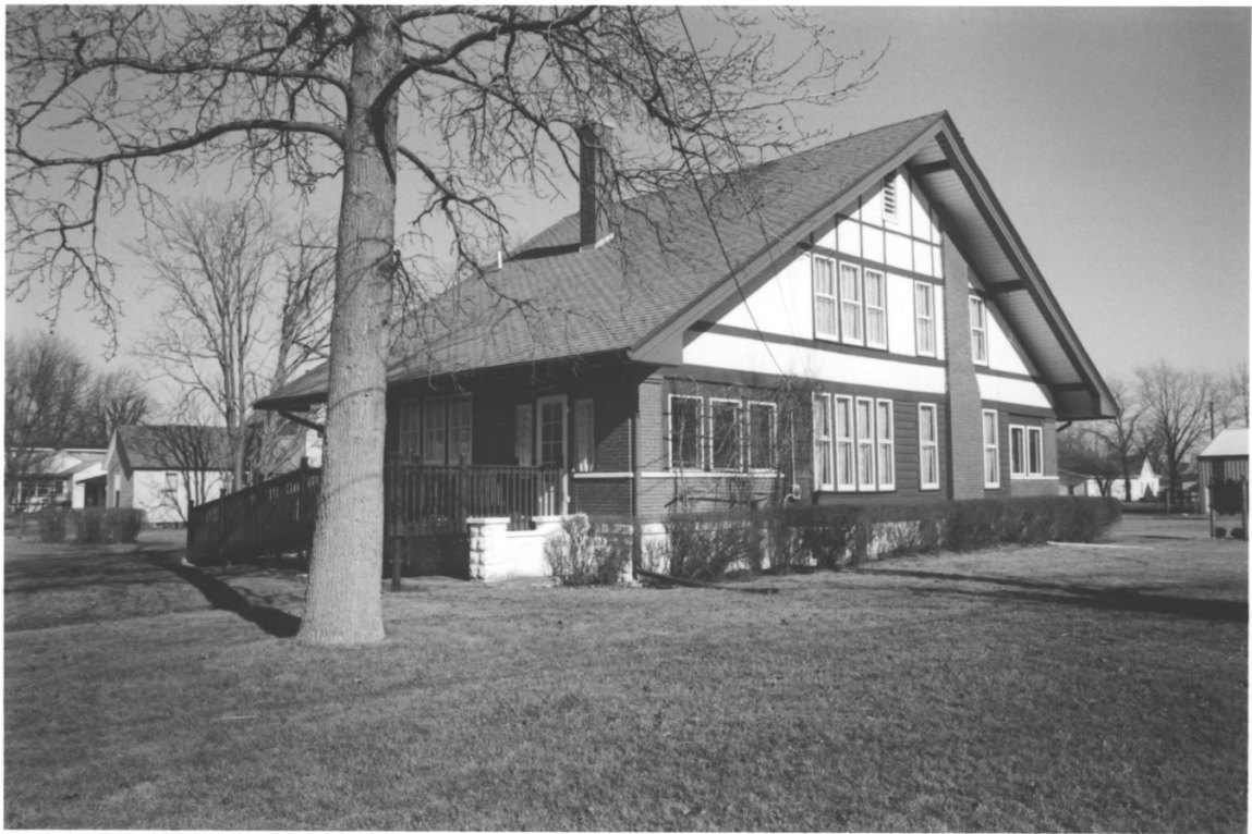
Scott Lucas House Newton County 114
