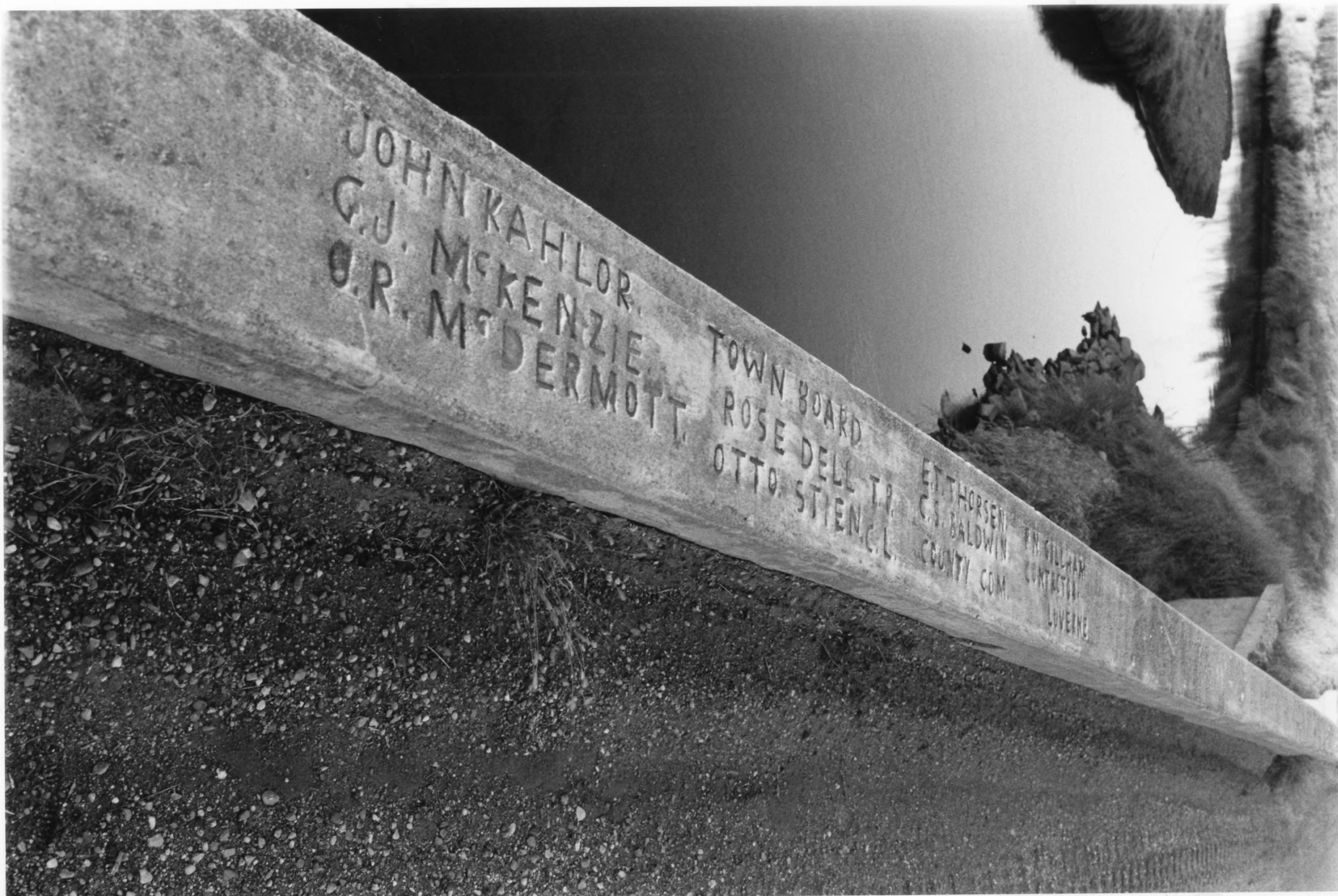
BRIDGE NO. L-2162 ROCK CO., MN ROSE DELL TOWNSHIP PHOTO I.D. 09168#9
