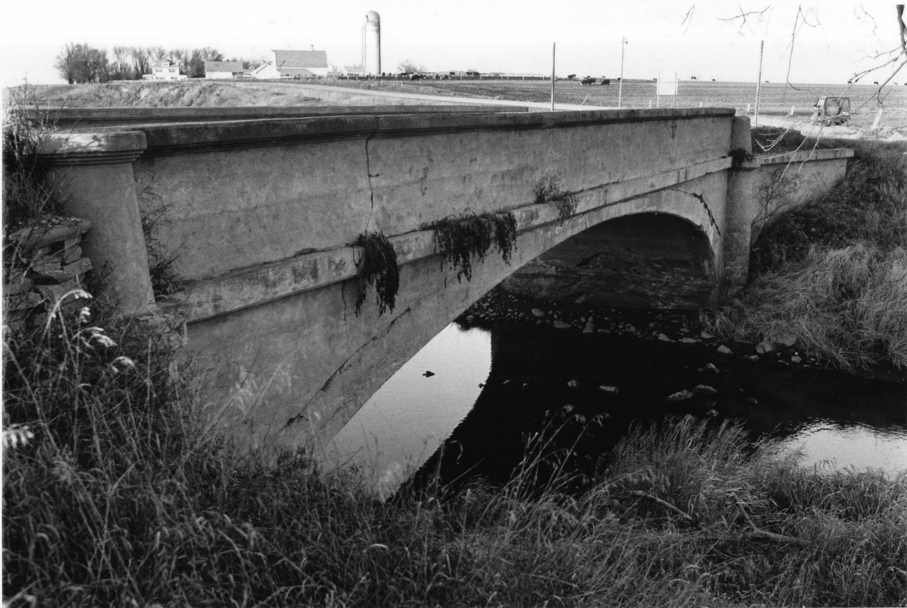
BRIDGE NO. L-2162 ROCK CO., MN ROSE DELL TOWNSHIP PHOTO I.D. 09168#4
