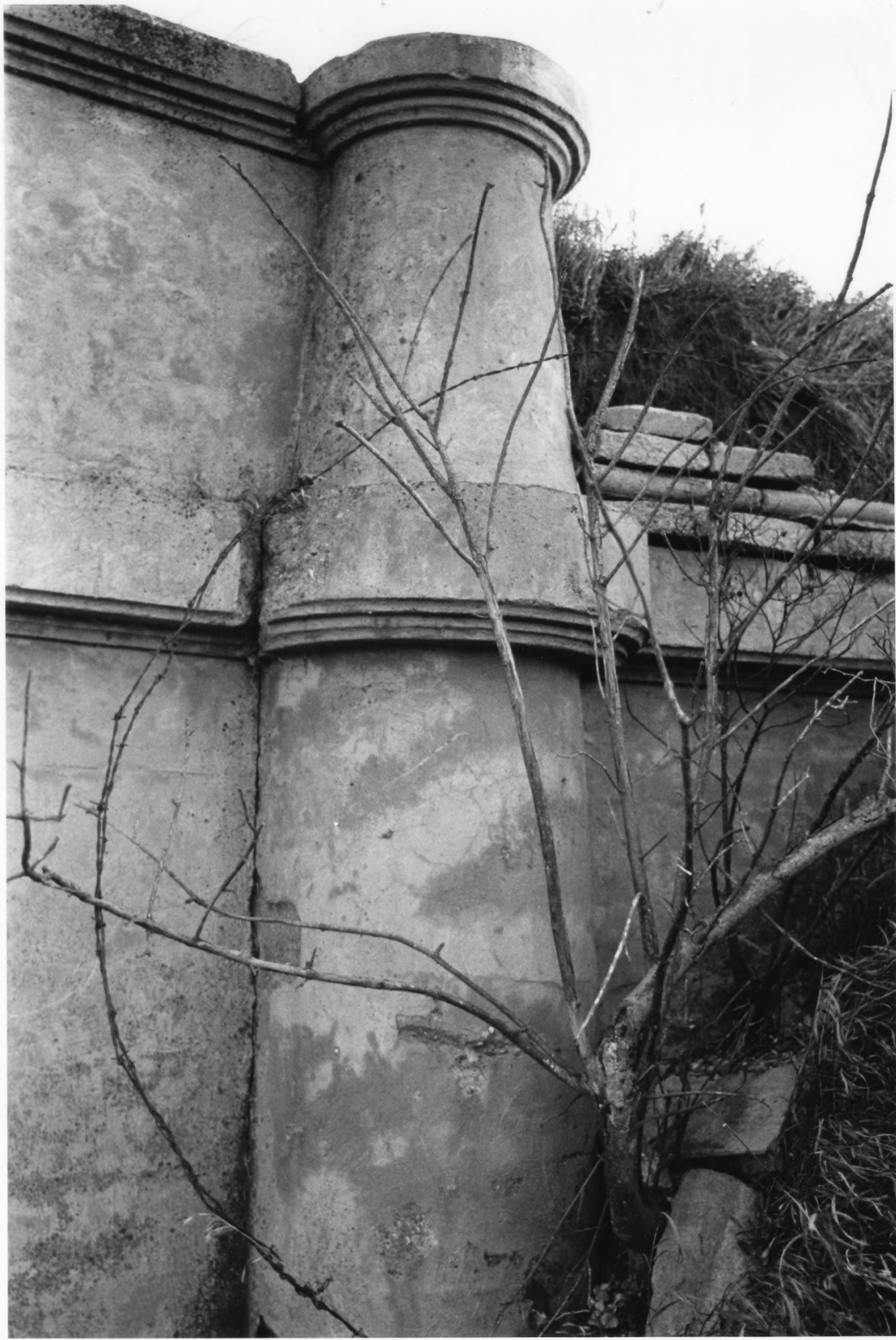
BRIDGE NO. L-2162 ROCK CO., MN ROSE DELL TOWNSHIP PHOTO I.D. 09168 #8
