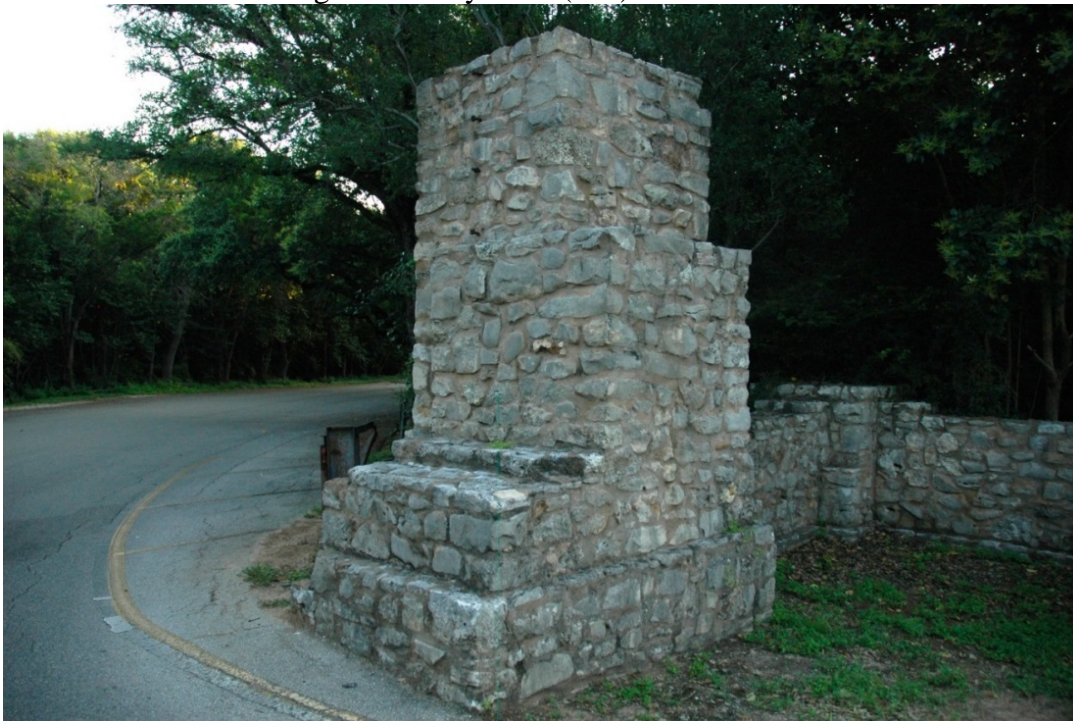
Photo 34: Camera facing SW. Entry Piers (#25).
