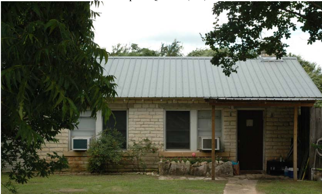
Photo 28: Camera facing S. Keeper's Quarters (#20) north elevation.
