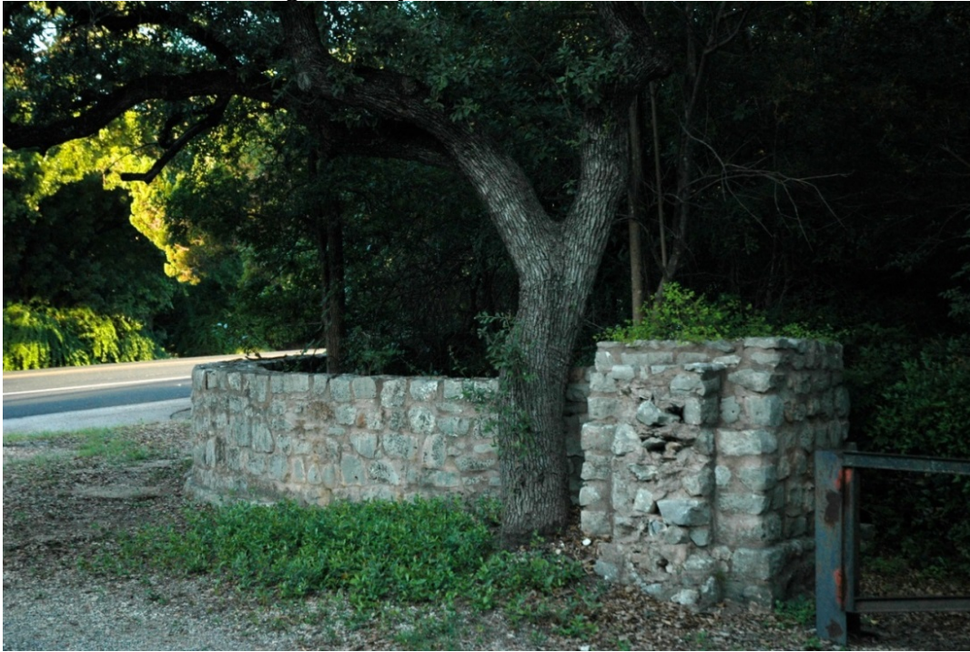
Photo 33: Camera facing E. Entry Piers (#25).
