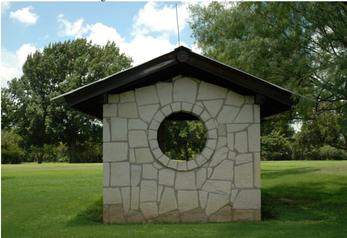
Photo 30: Camera Facing N. Limestone storm shelter (#22) between 3 rd tees and 8 th tees. South elevation.
