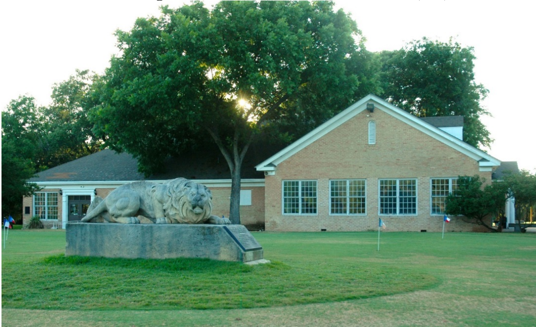
Photo 25: Camera facing W. 1930 Colonial Revival Clubhouse (#19) with Lion Statue (#26)
