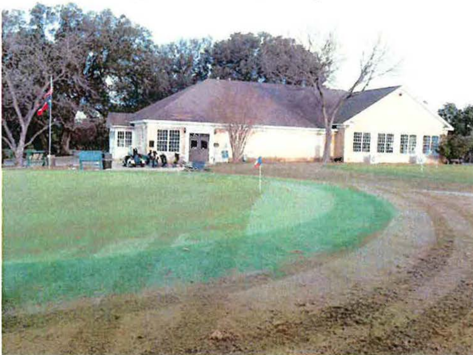
Figure 26. Clubhouse, Looking Northwest
