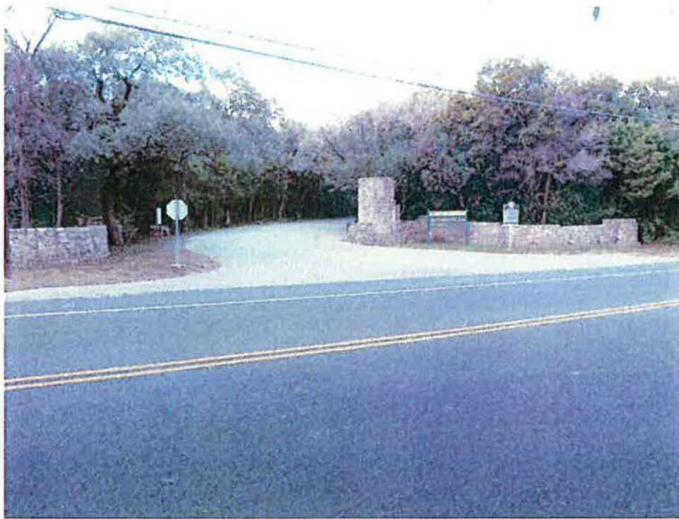
Figure 39. Entry Gate Piers, Looking Southwest
