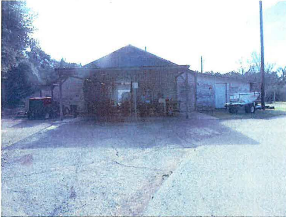
Figure 37. Maintenance Building, Looking South-Southeast
