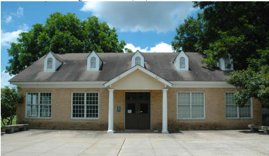
Photo 26: Camera facing S. Clubhouse (#19) north elevation.
