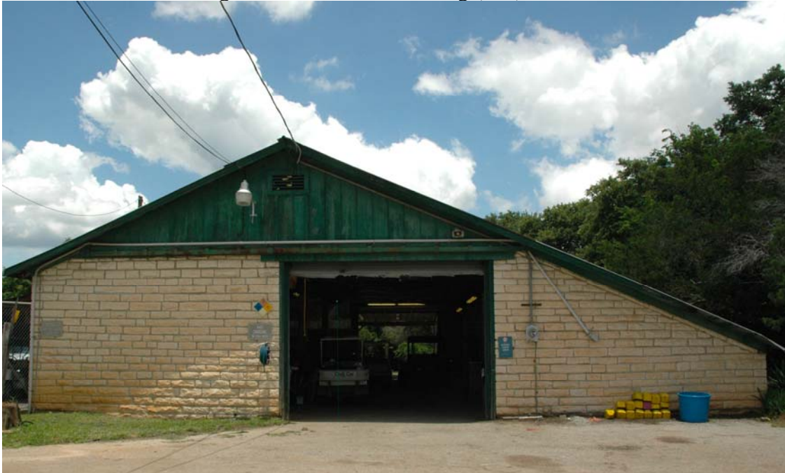
Photo 29: Camera facing N. Maintenance Building (#21) south elevation.
