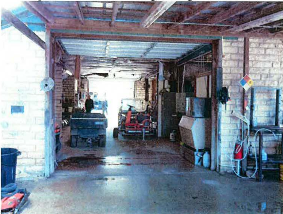
Figure 38. Maintenance Building, Looking South-Southeast
