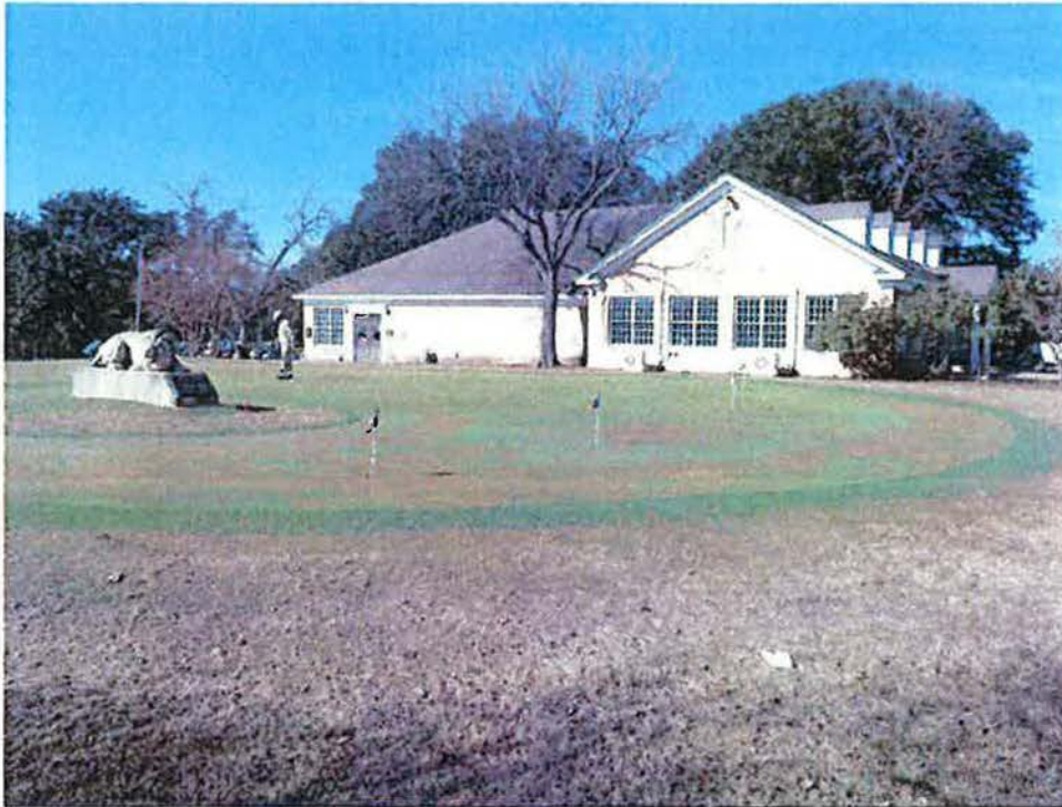
Figure 25. Clubhouse, Looking West
