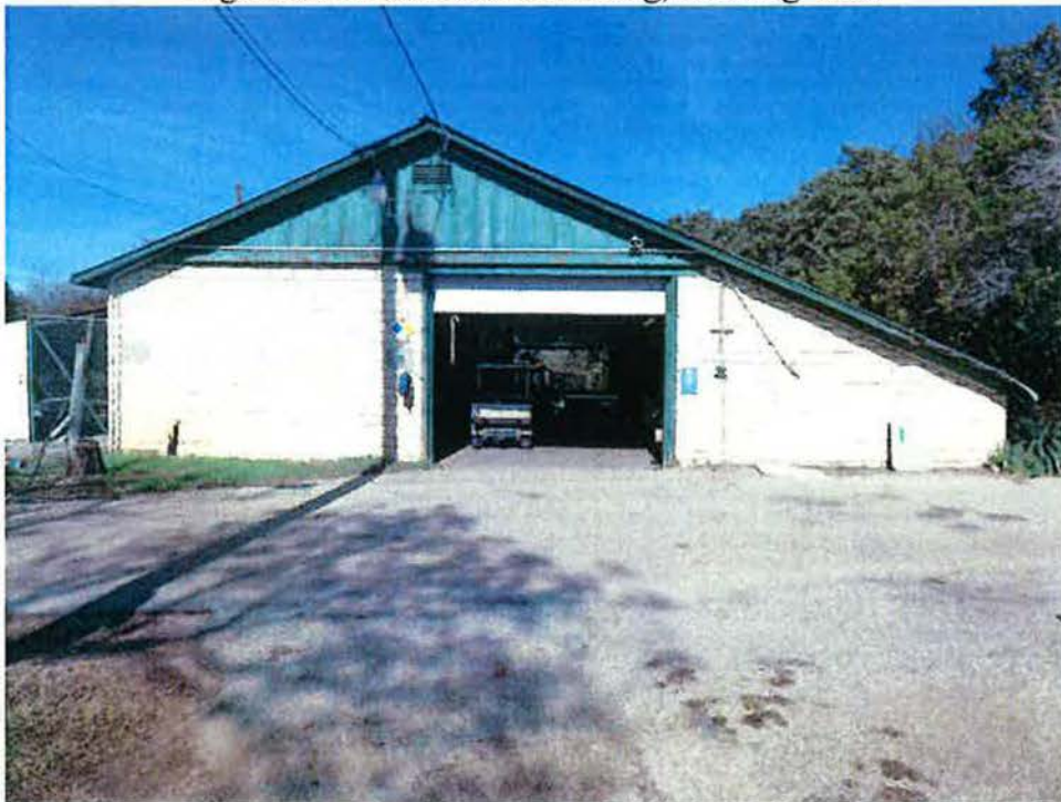
Figure 34. Maintenance Building, Looking Northwest
