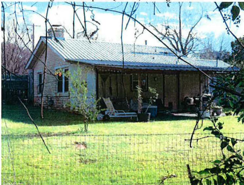
Figure 32. Keeper's Quarters, Looking East
