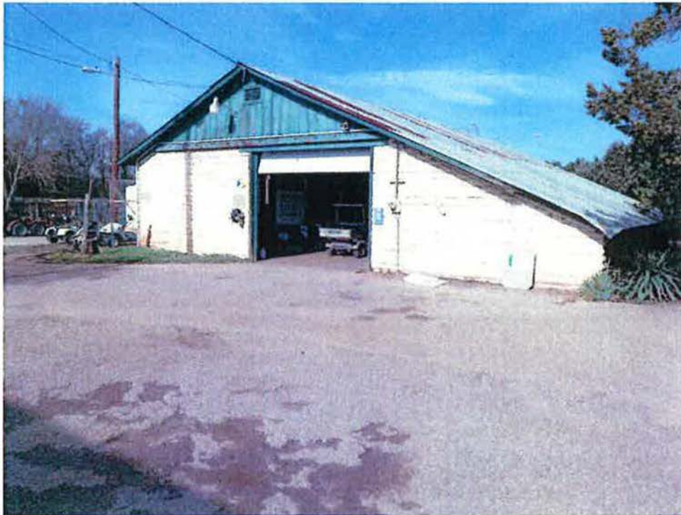
Figure 33. Maintenance Building, Looking West
