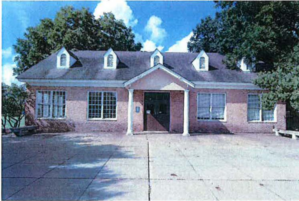
Figure 23. Clubhouse, Looking West
