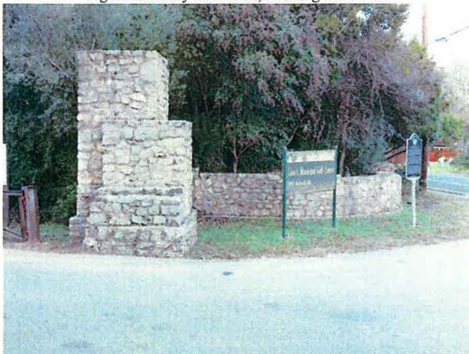
Figure 40. Western Entry Gate Pier, Looking West
