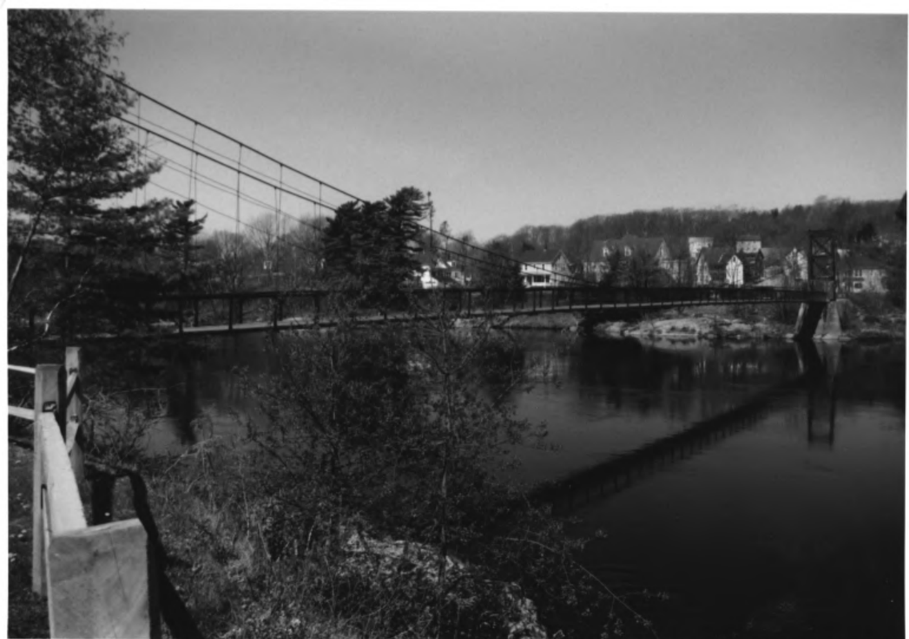
ANDROSCOGGIN SWINGING BRIDGE; CUMBERLAND AND SAGadahoc COUNTIES, MAINE
