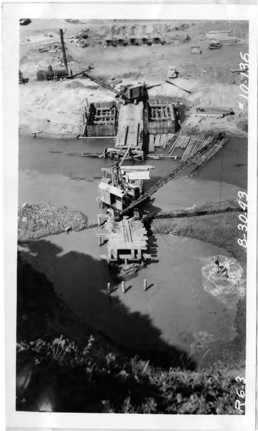
Figure 1: Albion River Bridge under construction, August 1943. California Department of Transportation archive.
