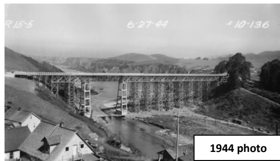
Figure 1. The Albion River Bridge
