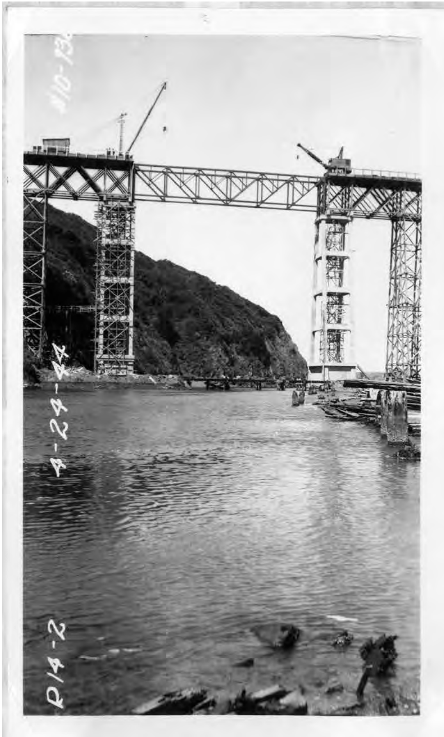
Figure 4: Albion River Bridge under construction, April 1944. California Department of Transportation archive.
