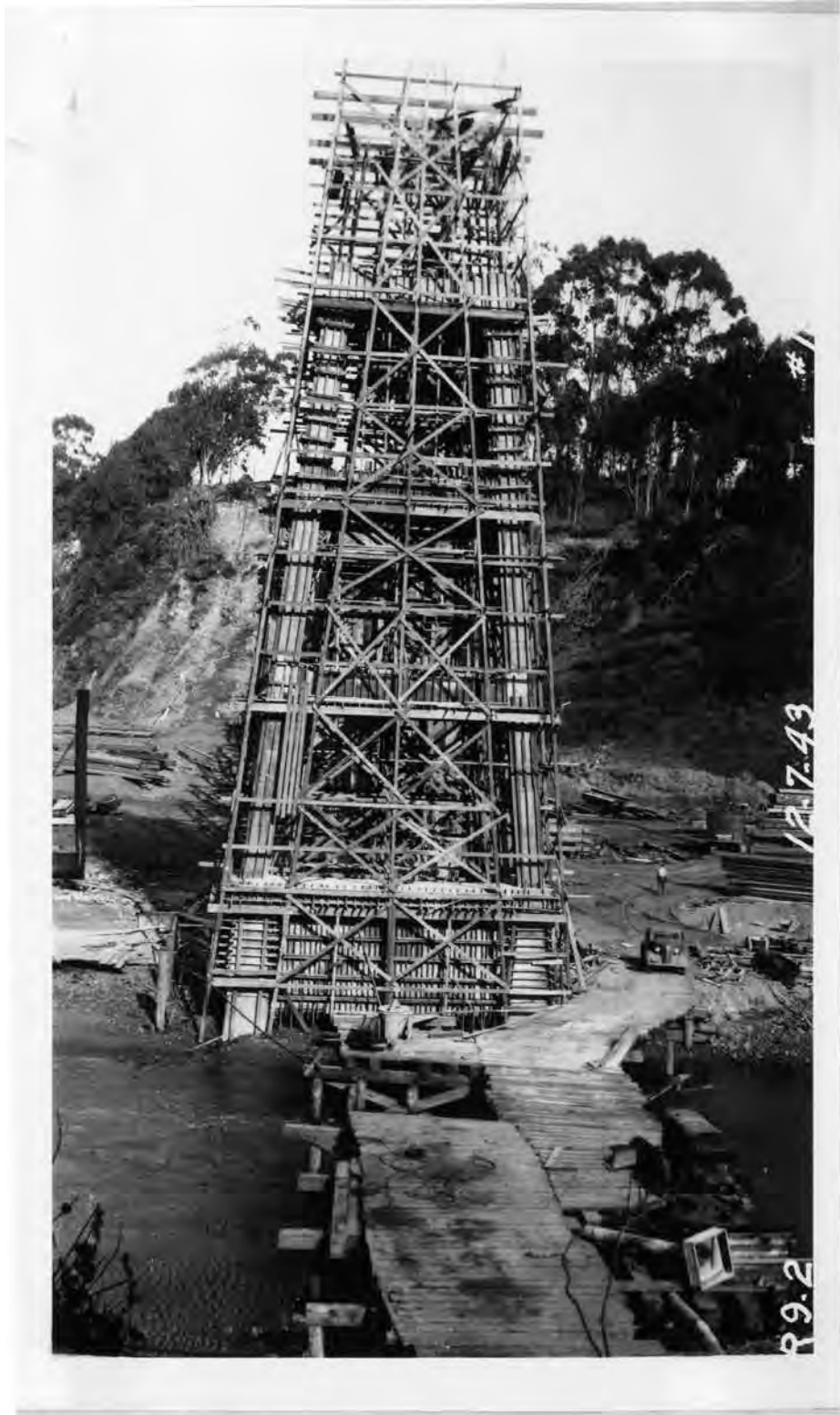
Figure 2: Albion River Bridge under construction, December 1943. California Department of Transportation archive.
