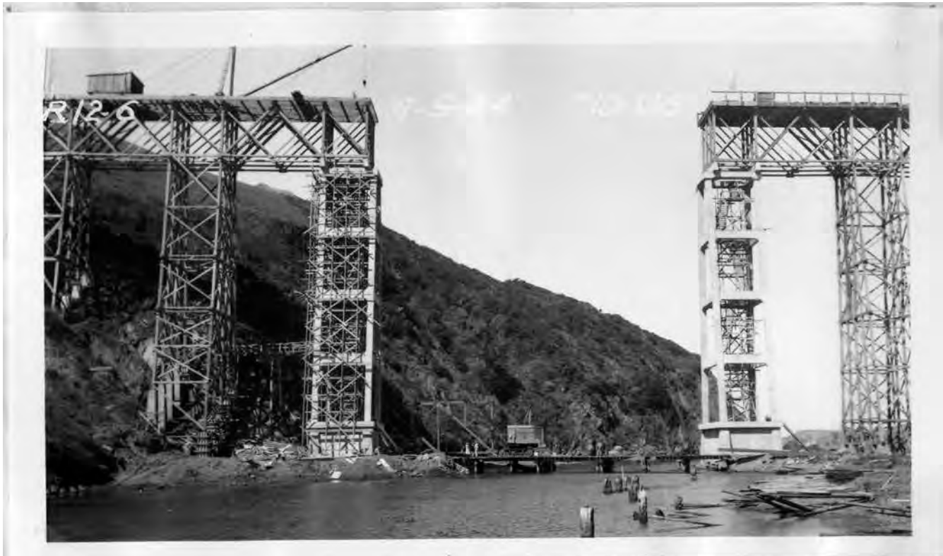
Figure 3: Albion River Bridge under construction, April 1944. California Department of Transportation archive.
