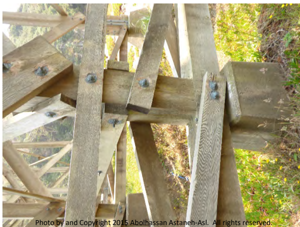
The bolts connecting the timber members are in good condition in these 2015 photos
