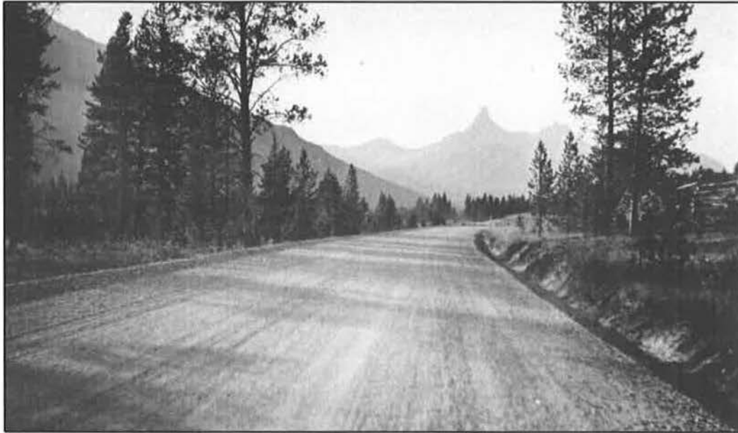
“Looking toward Cooke from Stuart's Ranch on Section Portion of D at Station 2780 after surfacing was laid.” Final Construction Report (1934-1935) on Red Lodge-Cooke City Approach Road to Yellowstone National Park, on Section B and Portion of D Surfacing. H. E. Mitchell, 1935. Photo No. 29145 from page 1.
