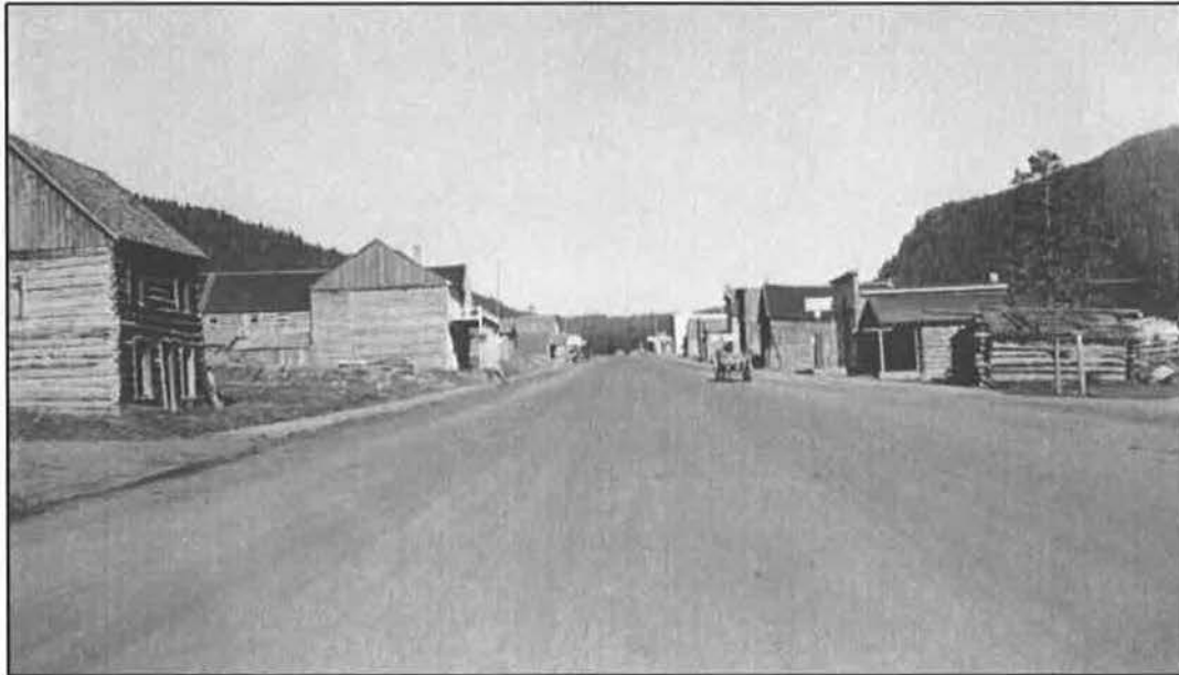
“Looking east thru Cooke City at Sta. 3430+00.” Final Construction Report (1935-1936) on Red Lodge-Cooke City Approach Road to Yellowstone National Park, on Section D (Portion), Surfacing, Bituminous Base Treatment and Bituminous Road Mix. L. A. Deklotz, 1936. Photo No. 29846 from page 15.
