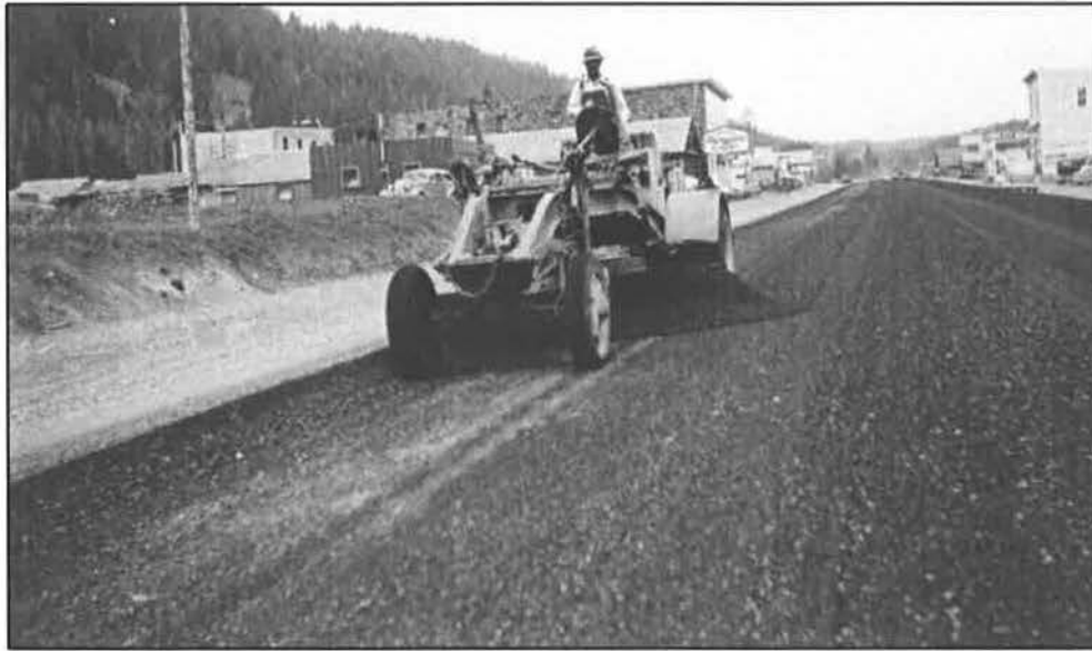
“Processing road mix in Cooke City.” Final Construction Report (1935-1936) on Red Lodge-Cooke City Approach Road to Yellowstone National Park, Section D (Portion), Surfacing, Bituminous Base Treatment and Bituminous Road Mix. L. A. Deklotz, 1936. Photo No. 29131 from page 5.
