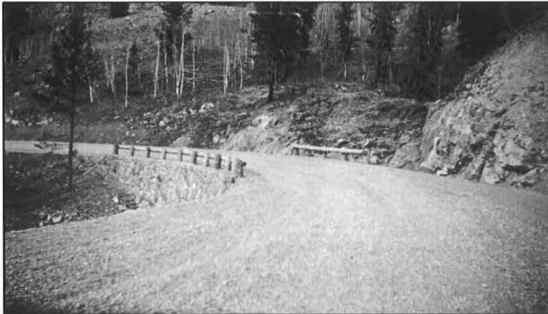
“Roadway view over Rock Creek culvert at Station 2730.” Final Construction Report (1932-1934) on Section D, Grading Red Lodge-Cooke City Approach Road to Yellowstone National Park, H. E. Mitchell, 1934. Photo No. 26054 from page 8.
