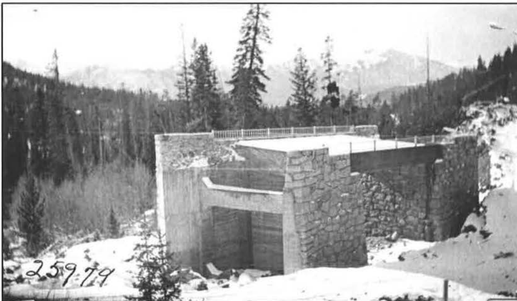
“Muddy Creek Bridge showing concrete abutments with stone facing.” Final Construction Report (1931-1933) on Section B, Grading Red Lodge-Cooke City Approach Road to Yellowstone National Park, H. E. Mitchell, 1934. Photo No. 25979 from page 25.
