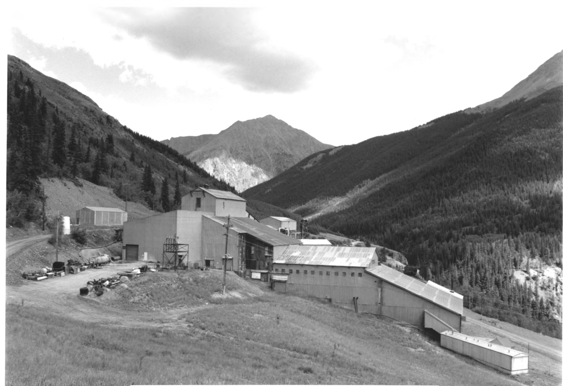
Photograph #3 Shenandoah-Dives Mill Silverton Vicinity, San Juan County, Colorado Mill, North from Tailings Pond #1 Frederick Athearn, San Juan County Historical Society, September 1995
