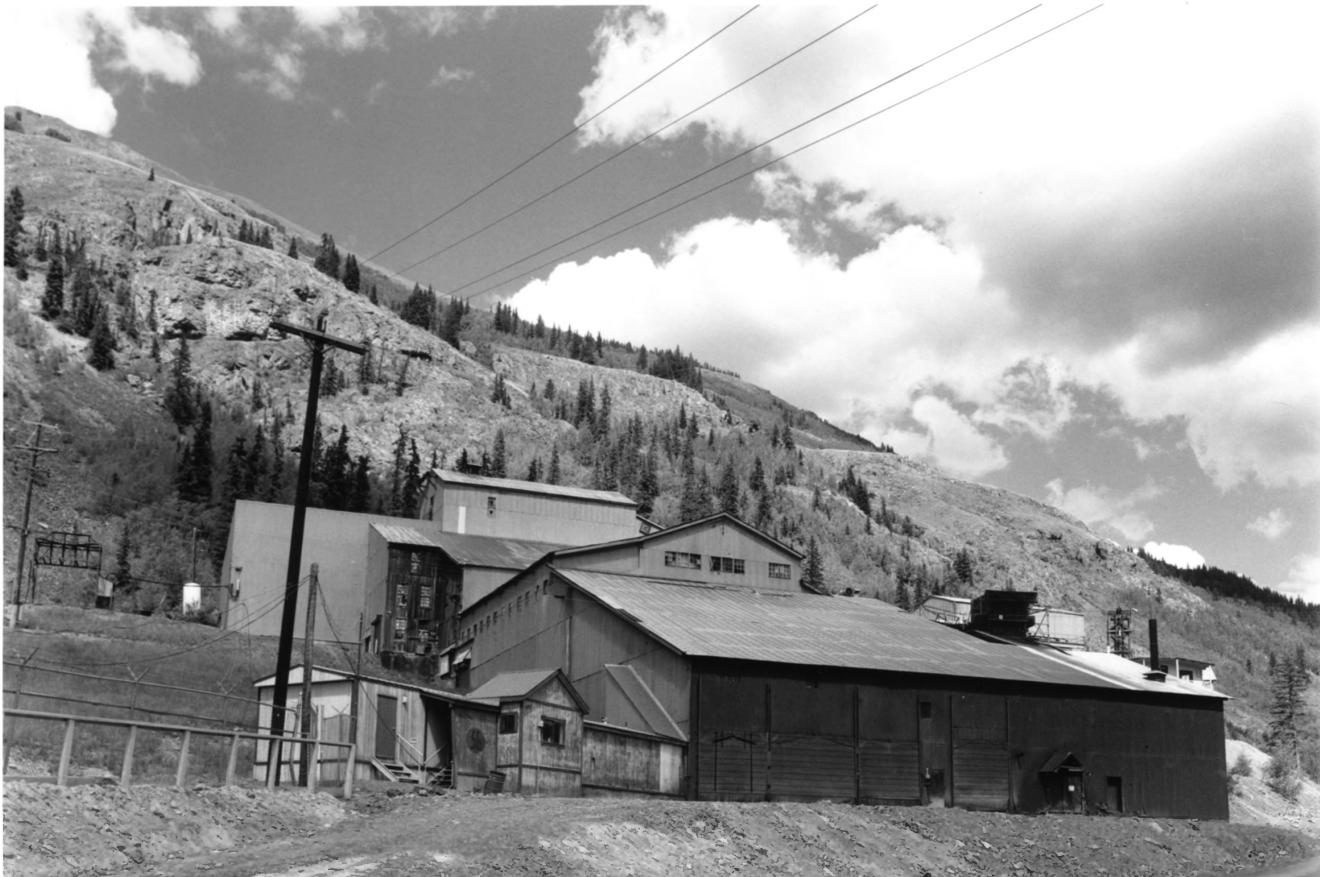
Photograph #4 Shenandoah-Dives Mill Silverton Vicinity, San Juan County, Colorado Mill, North Frederick Athearn, Historian, San Juan County Historical Society, September 1995
