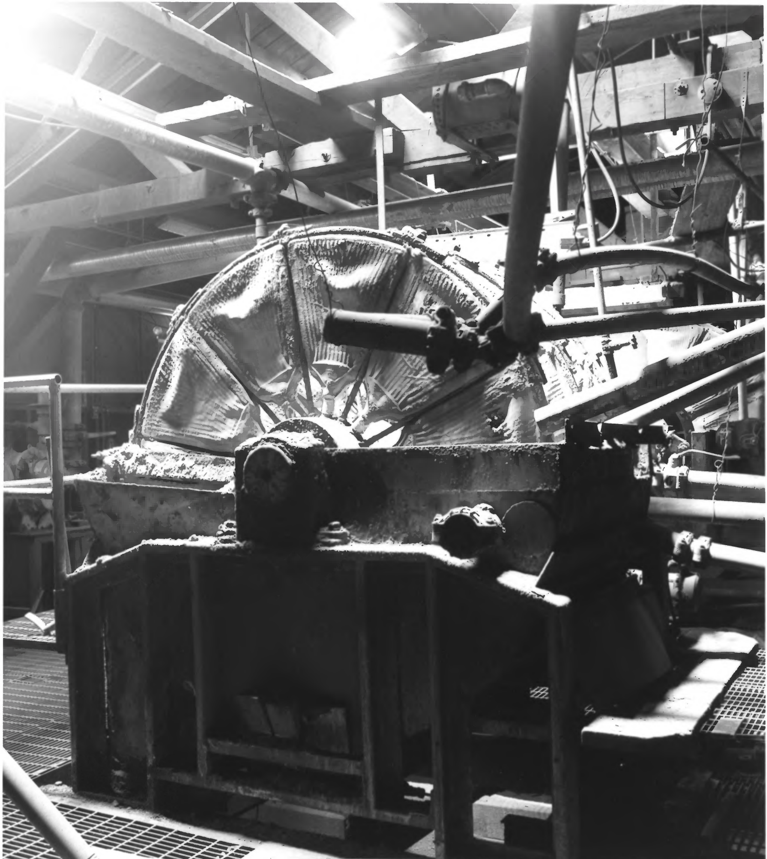
Photograph #31 Shenandoah-Dives Mill Silverton Vicinity, San Juan County, Colorado Canvas Wheel Filter (#32 & 33 on Flow Chart) Silver Rich Images (John Matsko), Olathe, Kansas, August 1998
