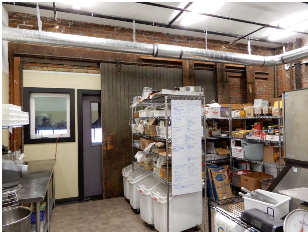
12 of 25 – Converted kitchen area. View towards north into one-story shed space.
