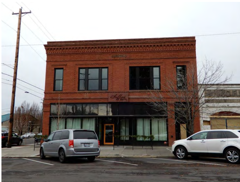
2 of 25 – Main façade of the Bachtold Building facing south.
