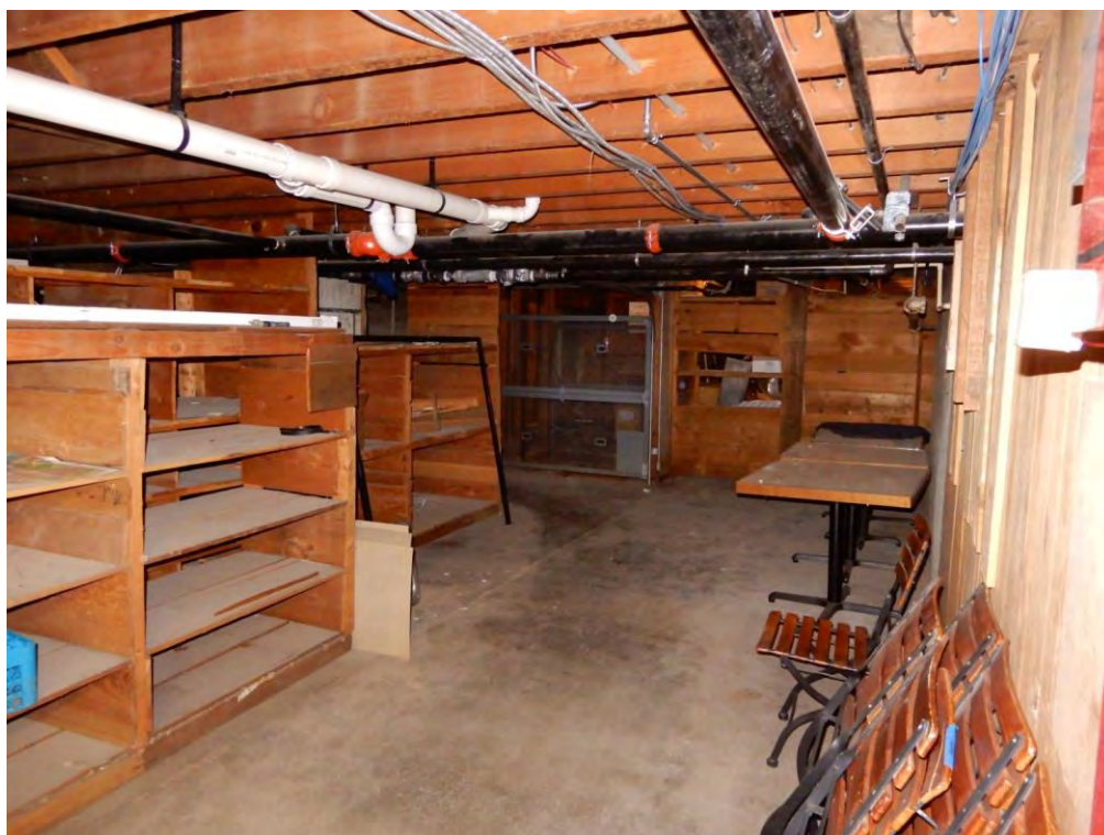
23 of 25 – Basement storage area.
