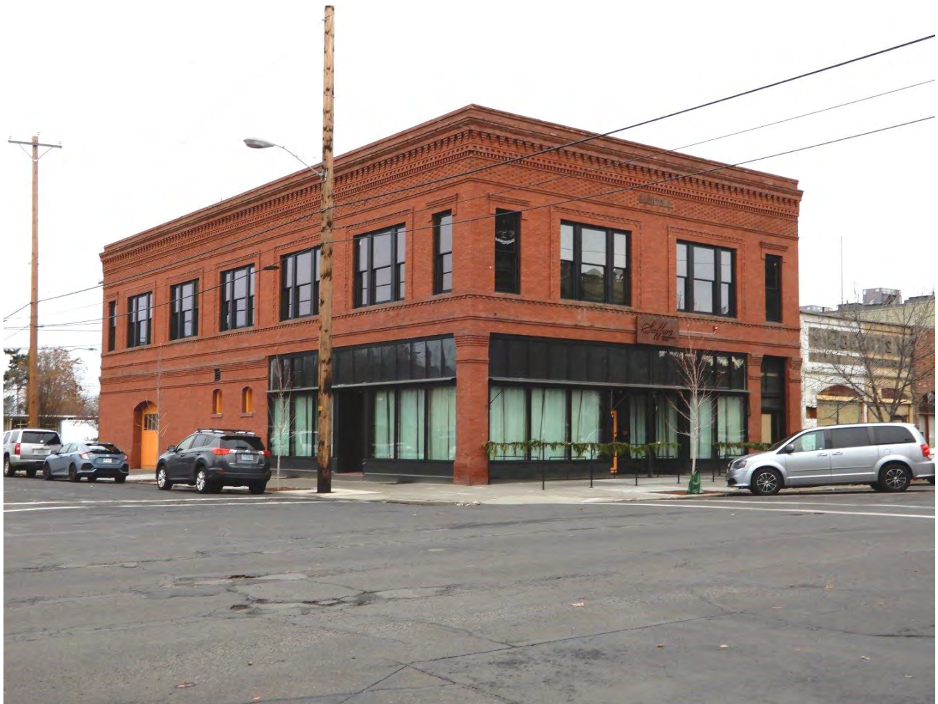
1 of 25 - Southwest corner, looking towards front of building.
