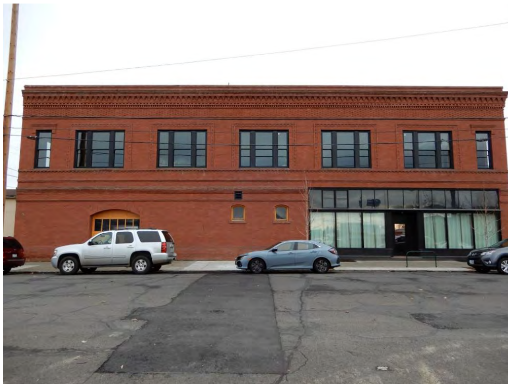
3 of 25 – West side of building showing main depot entry (right) and freight door (left)
