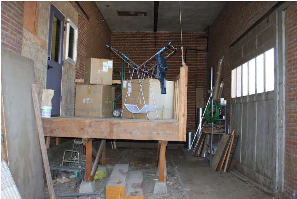
15 of 25 – Trolley car barn at northwest corner of building.
