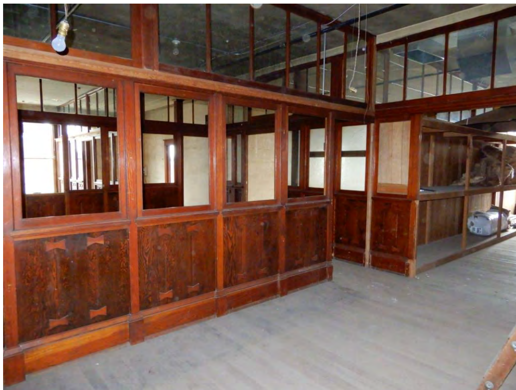
19 of 25 – Second floor office spaces.
