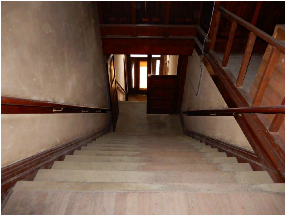
16 of 25 – Stairs leading from street to second floor office spaces.
