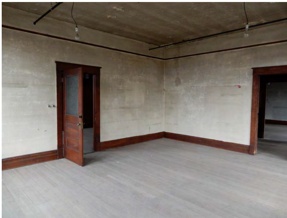
20 of 25 – Second floor office spaces.
