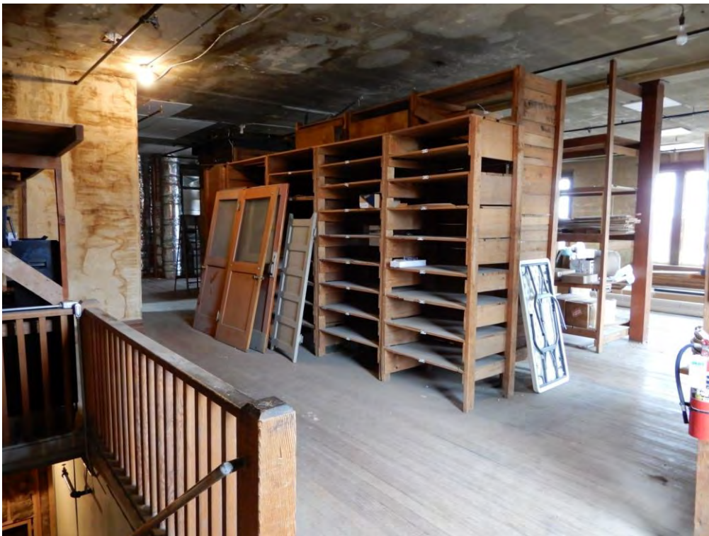
17 of 25 – Second floor office spaces rear stair area at northeast corner of building.
