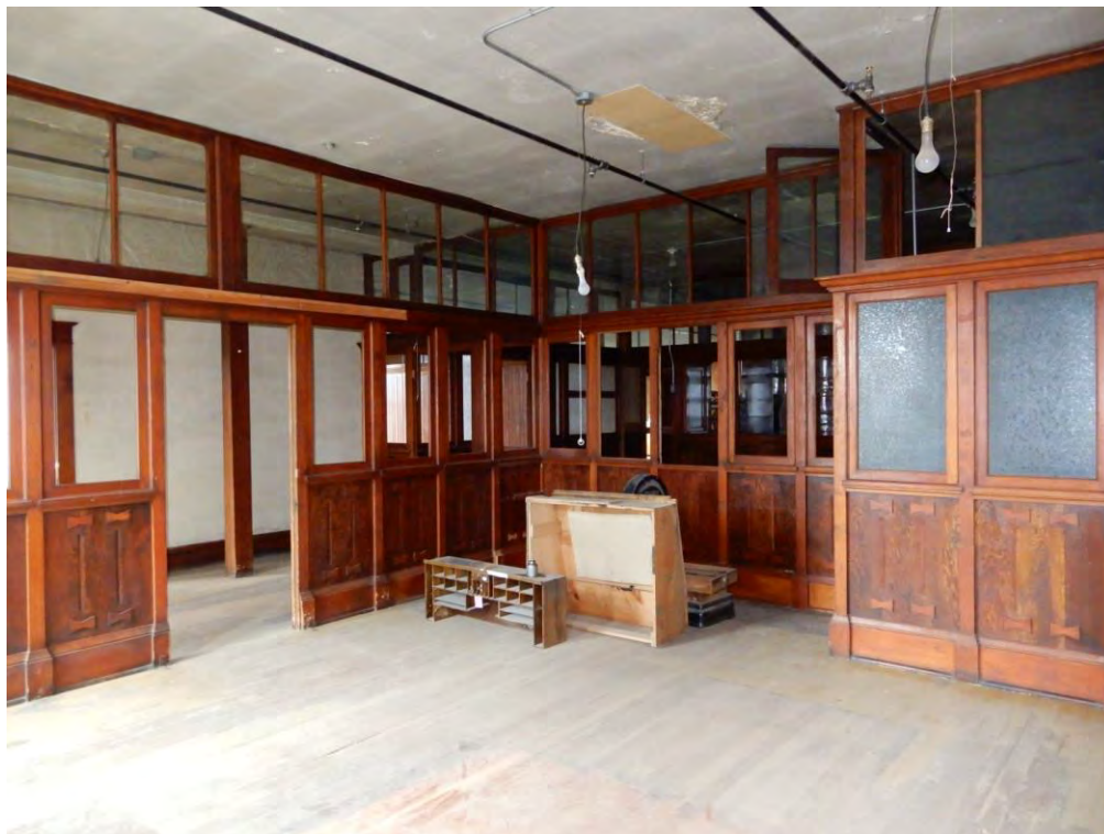
18 of 25 – Second floor office spaces.
