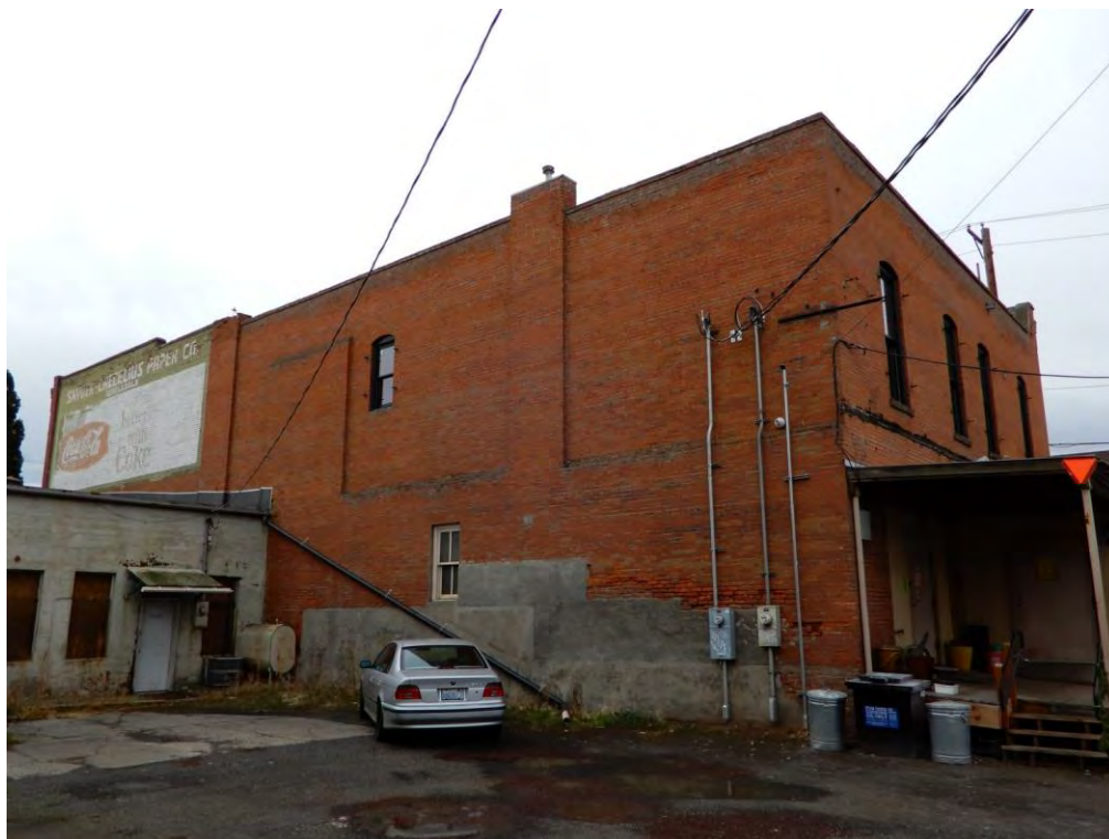
4 of 25 – East façade showing ghost sign.
