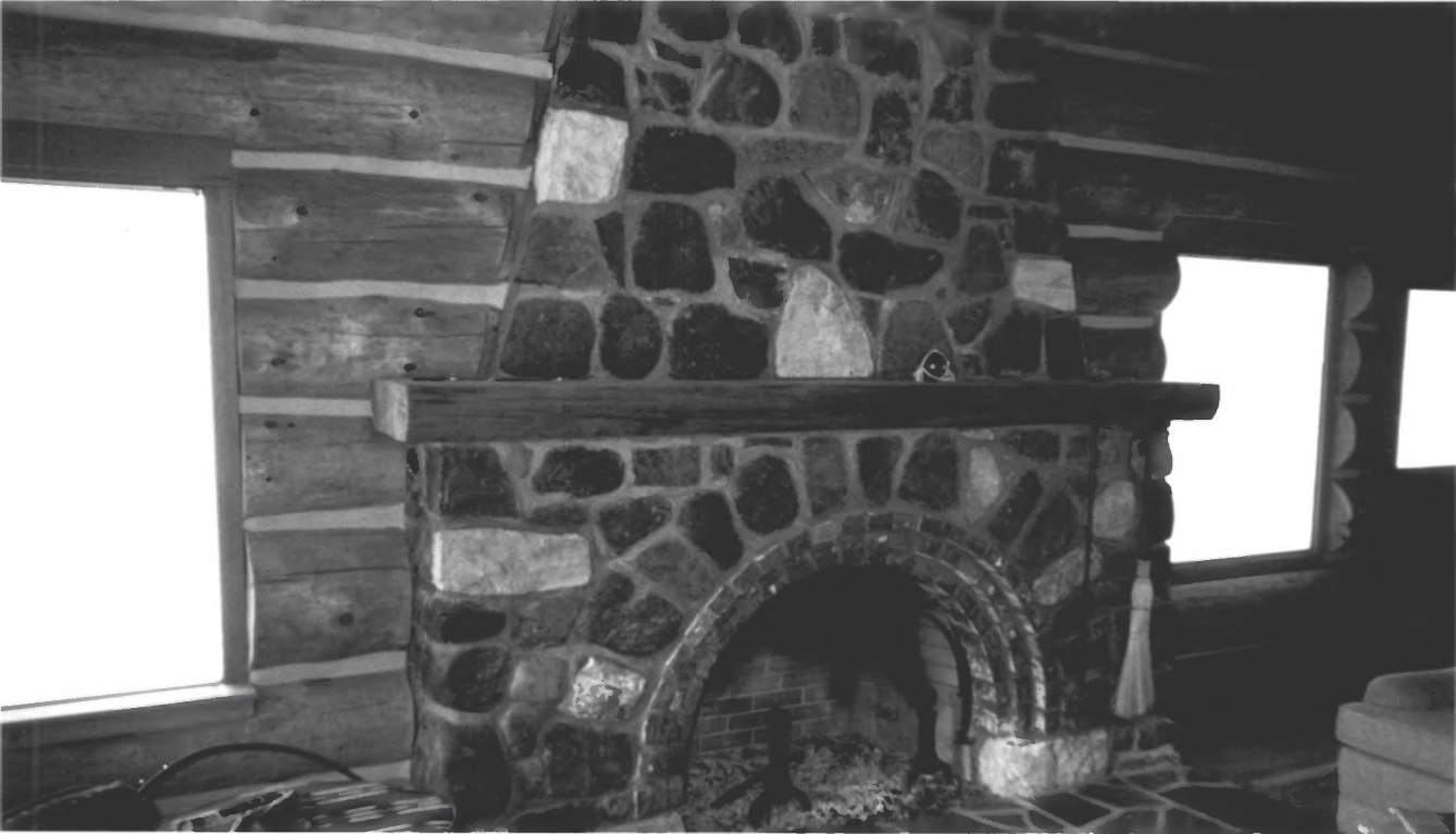
WEST - BOUVY LOG HOUSE, CLATSOP COUNTY, OR
