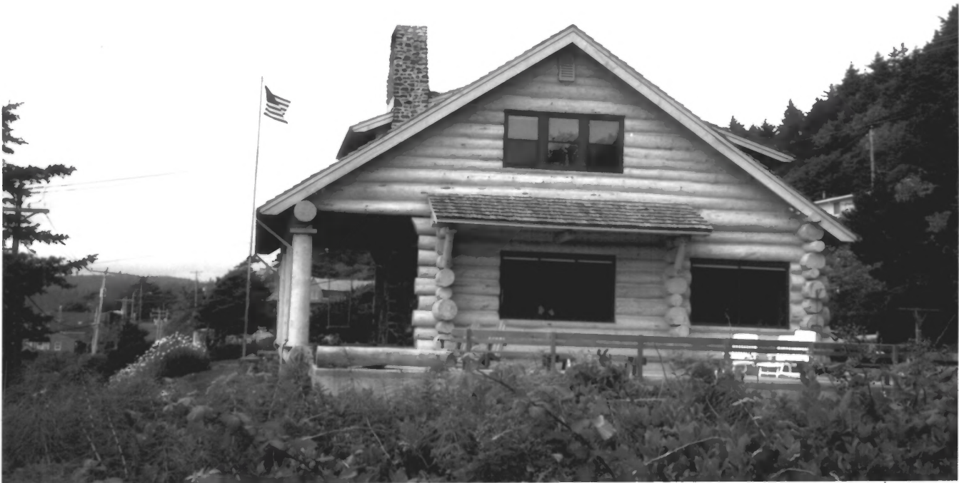
WEST -BOVY LOG HOUSE, CLATSOP COUNTY, OR
