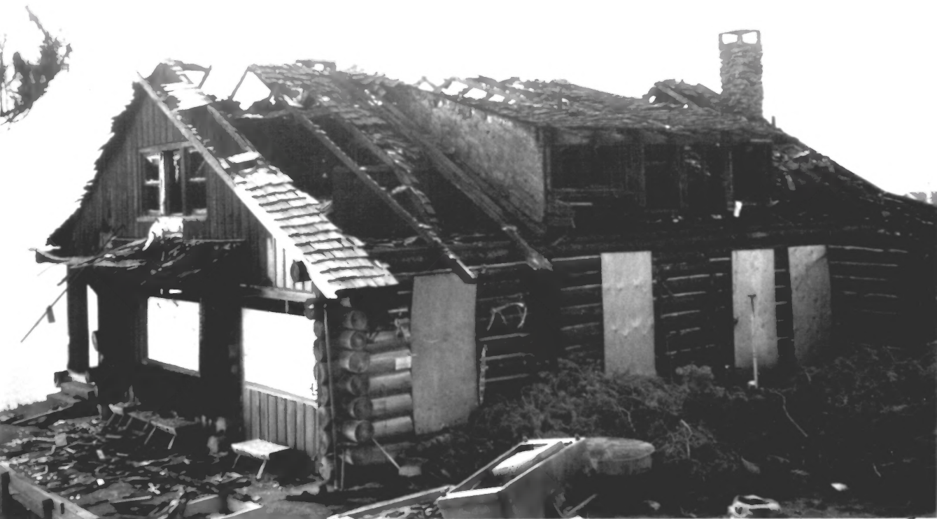
WEST-BOWNY LOG HOUSE, CLATSOP COUNTY, OR
