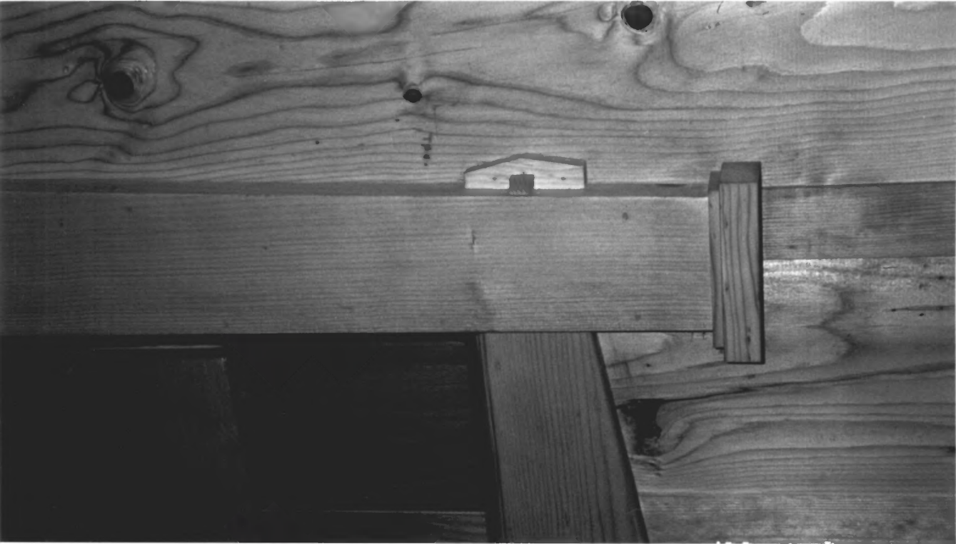
WEST-BOUVY LOG HOUSE, CLATSOP COUNTY, OR
