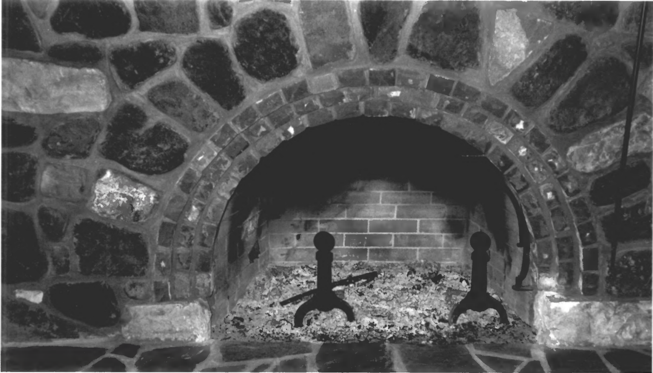
WEST BOUVY LOG HOUSE, CLATSOP COUNTY, OR
