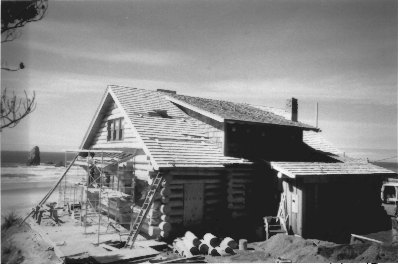
WEST-BOUVY LOG HOUSE, CLATSOP COUNTY, OR
