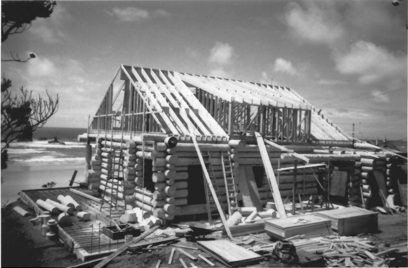
WEST-BOUVY LOG HOUSE, CLATSOP COUNTY, OR
