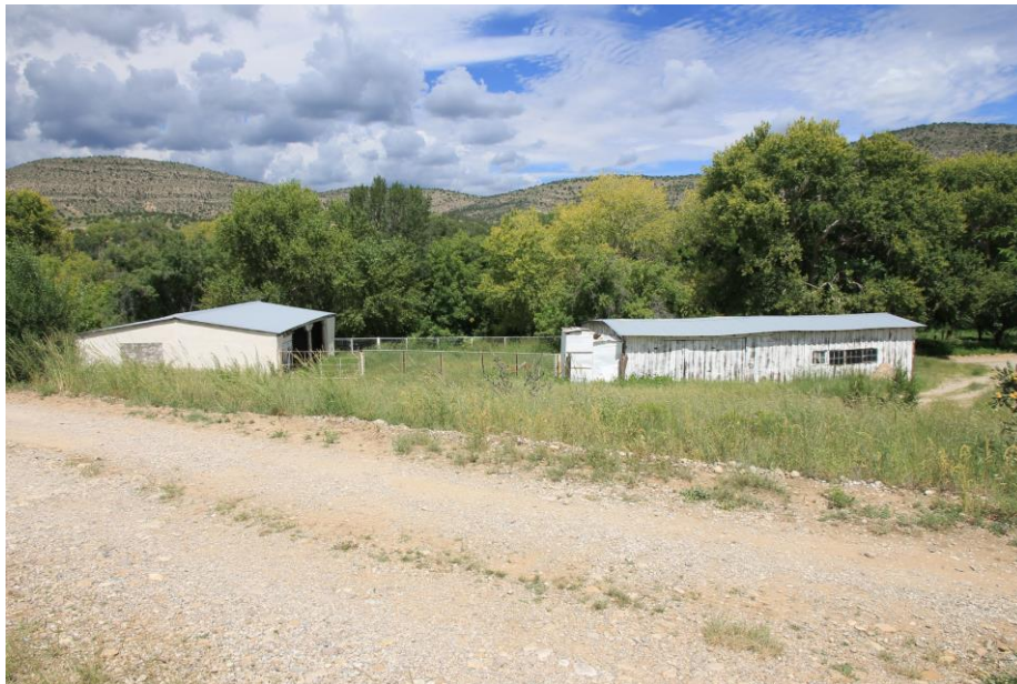
45 of 54. Stable (left) and long garage (right), photographer facing northeast.
