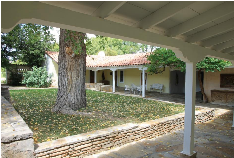
18 of 54. Main house, placita , interior courtyard, photographer facing north.
