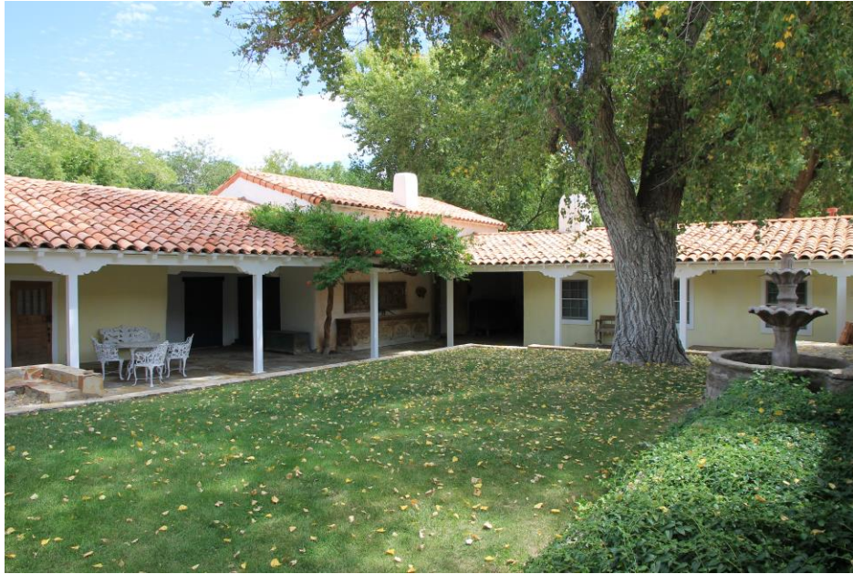
21 of 54. Main house, placita and Peter Hurd studio (center) and Wyeth Wing (right), photographer facing east.
