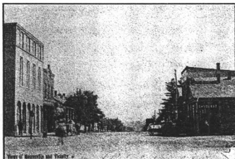
Fig. 26 “Views of Mooresville and Vicinity” showing East Main Street and the early Bass Drugstore at lower right. The IOOF building at left has lost its third floor. Photo by J. P. Calvert. Source: Mooresville Times , 8 August 1974.
