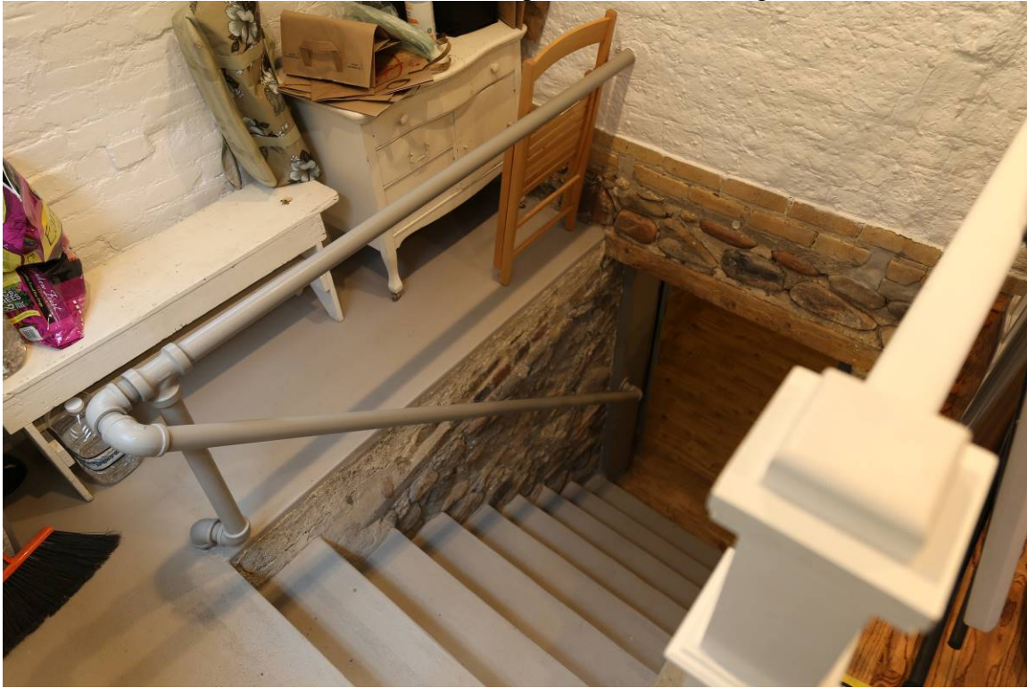
15 of 20. Basement entrance within enclosed porch. Camera facing southeast.
