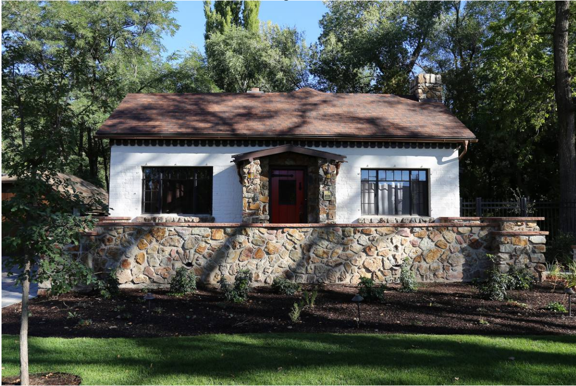
1 of 20. Front (south) façade. Camera facing north.
