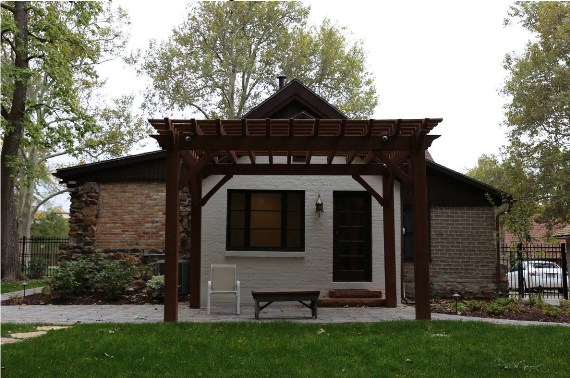
6 of 20. North façade. Camera facing south.
