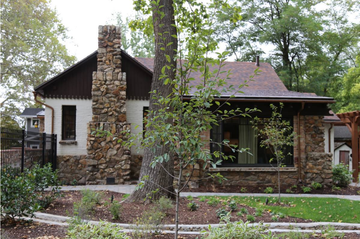
4 of 20. East façade. Camera facing west.
