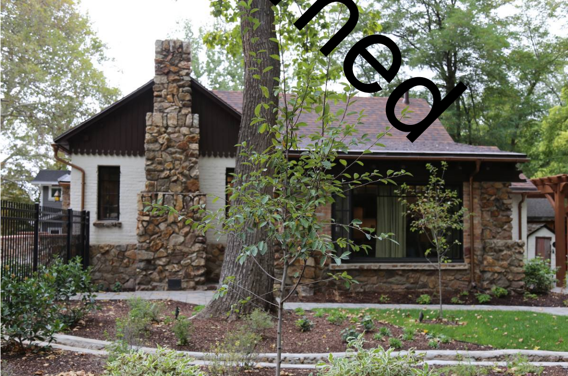
4 of 16. East façade. Camera facing west.
