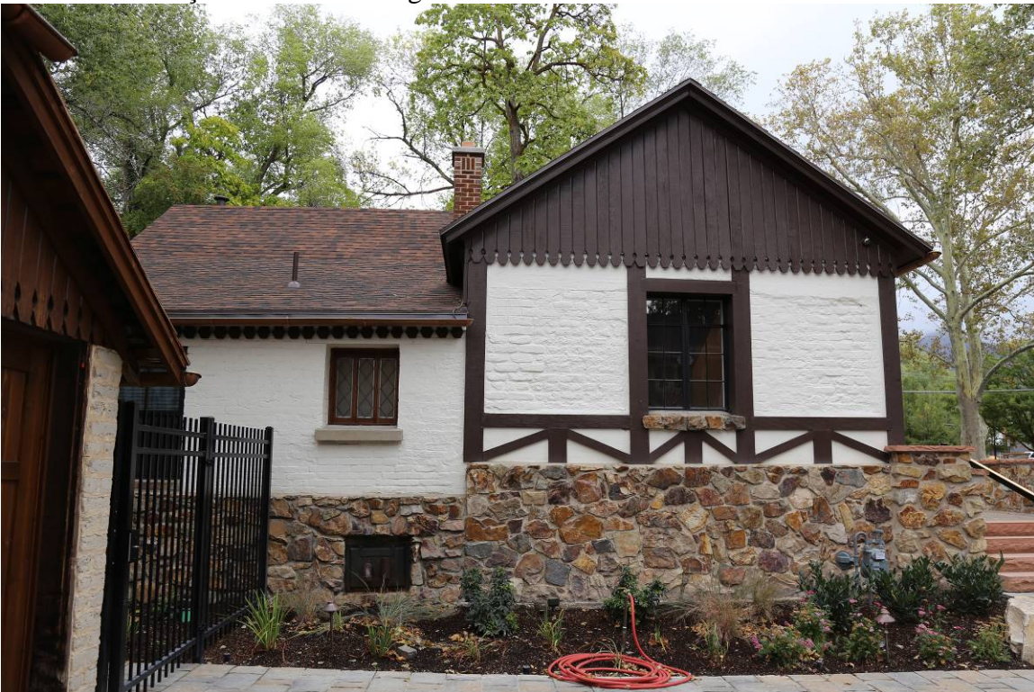
8 of 20. West façade. Camera facing east.
