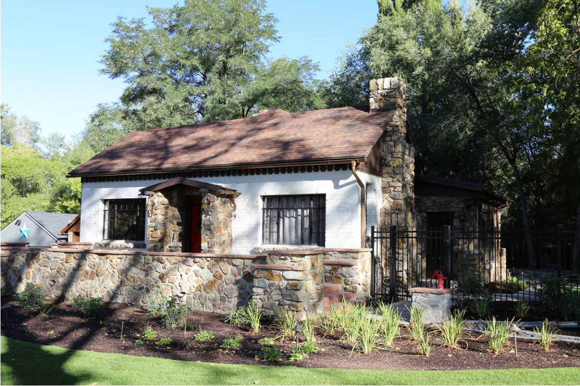
3 of 20. Southeast façade. Camera facing northwest.
