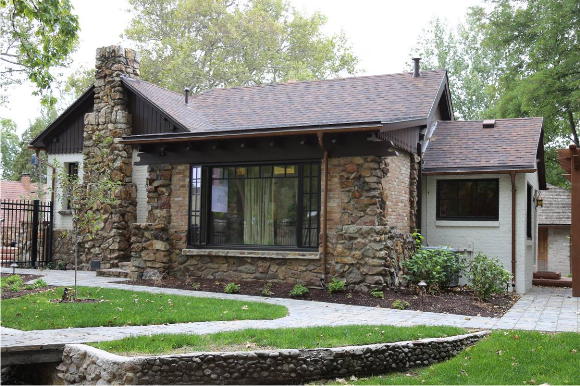
5 of 20. Northeast façade. Camera facing southwest.
