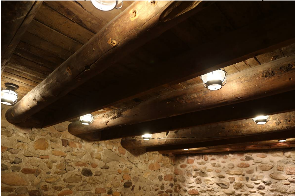
12 of 20. Basement floor joist and cobblestone wall construction. Camera facing northwest.
