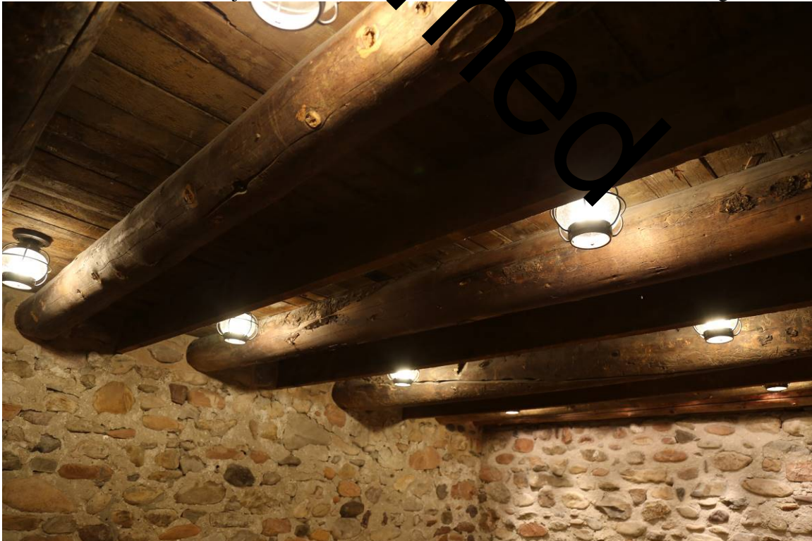
12 of 16. Basement floor joist and cobblestone wall construction. Camera facing northwest.
