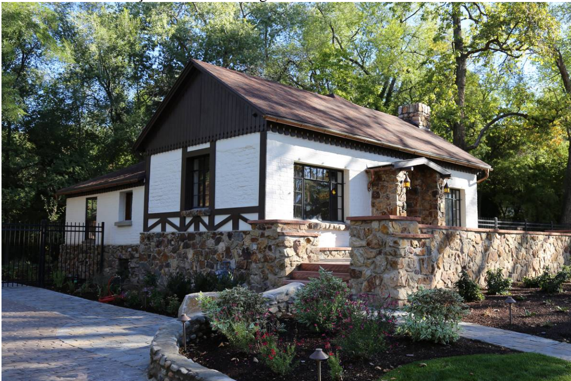
2 of 20. Southwest façade. Camera facing northeast.
