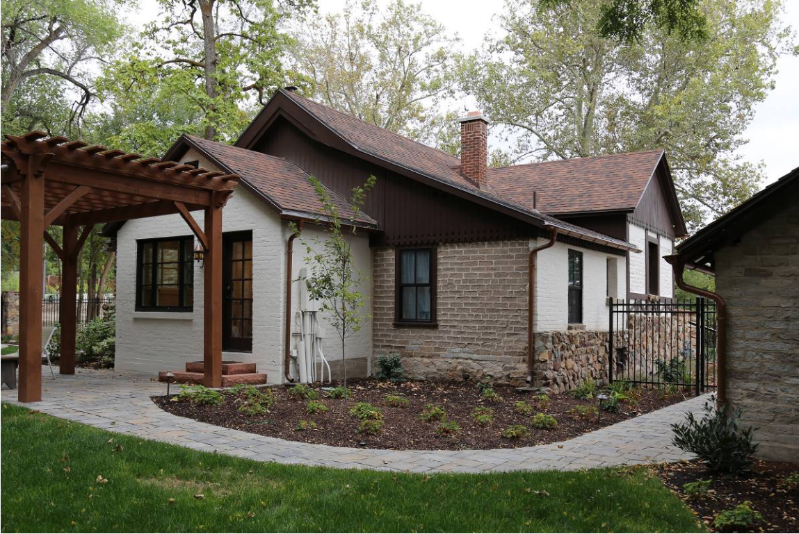
7 of 20. Northwest façade with garage. Camera facing southeast.
