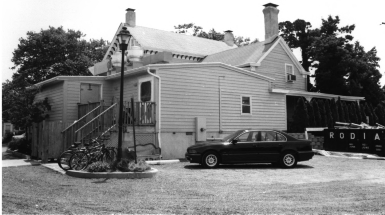
Whilldin-Miller House Cape May Co., NJ # 3
