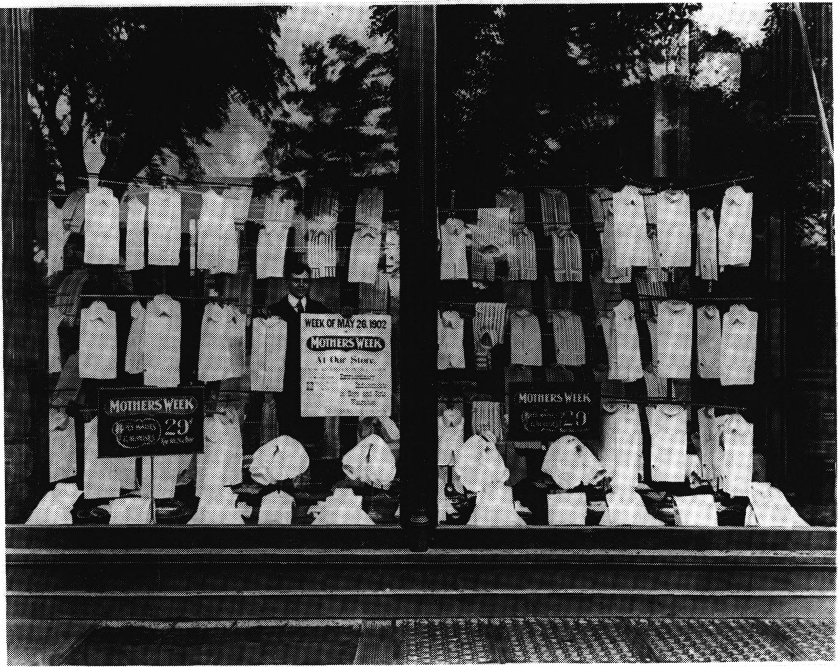
Plate 4 of 9: Display window, probably Halsey Street elevation, Mother's Week Sale, May 1902. View looking east.
