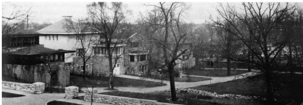
Fig 23: Houses on State Street, viewed from the south, before the construction of the second floor addition above the Rule House veranda, and of the MacNider House. Date Unknown, probably late 1910s, taken before the second floor addition above the Rule veranda. Historic Postcard, Paul Kruty collection.
