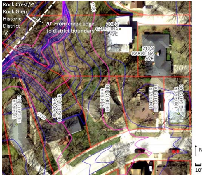
Fig. 13: Aerial view of 78 and 86 River Heights Drive, and 204 South Carolina, clarifying partial property boundary line. Willow Creek is to the northwest (upper left). Base map City of Mason City, generated by LIDAR, formatted 2015.
