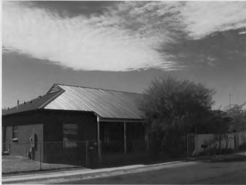
Photograph 13. 545-547 W. Shibell St.; view south.
