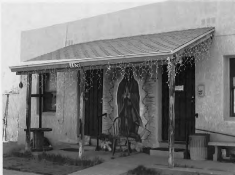
Photograph 15. 632 N. Anita Ave.; view north-northeast.
