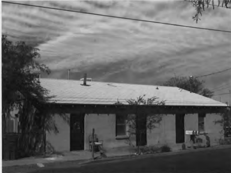
Photograph 23. 709-713 N. Anita Ave.; view west-northwest.
