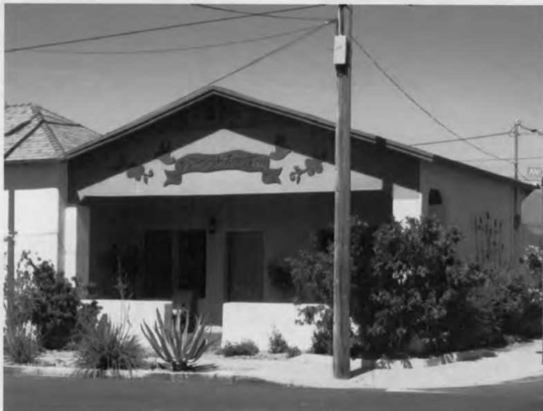
Photograph 5. 654 N. Anita Ave.; view northeast.
