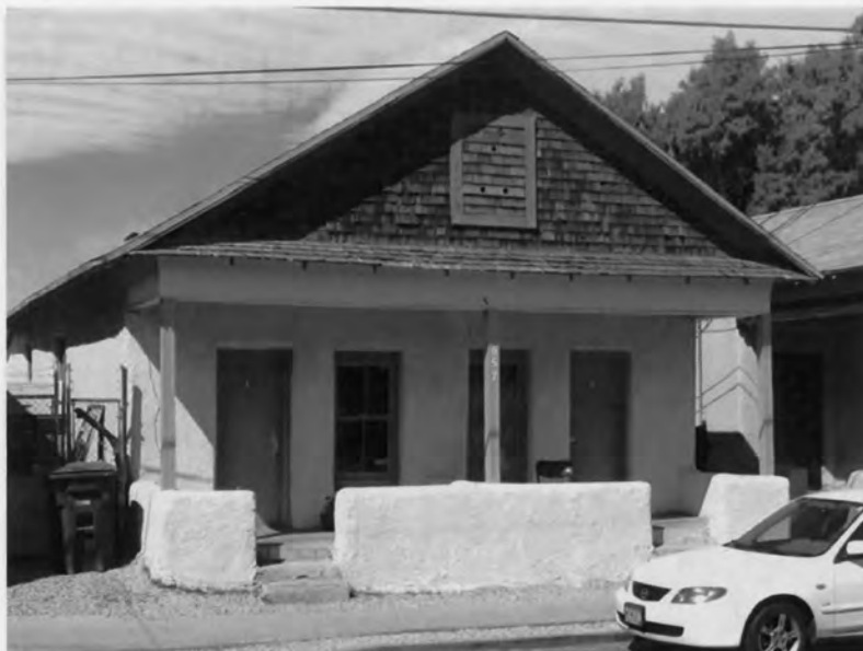
Photograph 4. 657 N. Anita; view west.
