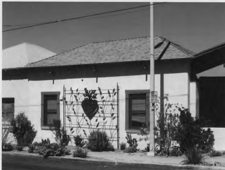
Photograph 21. 656 N. Anita Ave., view northeast.
