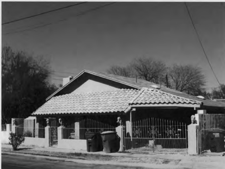
Photograph 14. 940 N. Anita Ave.; view northeast.
