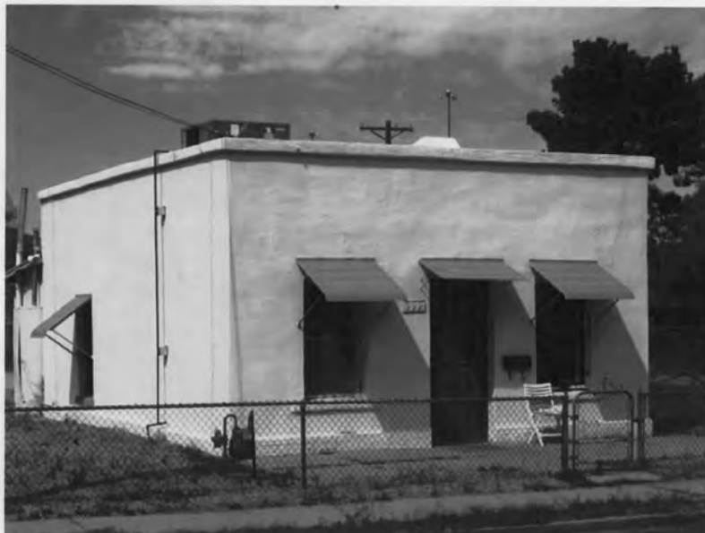
Photograph 17. 999 N. Anita Ave.; view west-northwest.
