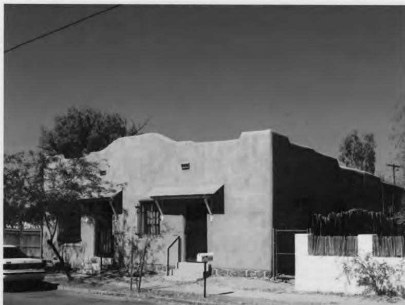
Photograph 22. 1000 N. Anita Ave.; view north-northeast.
