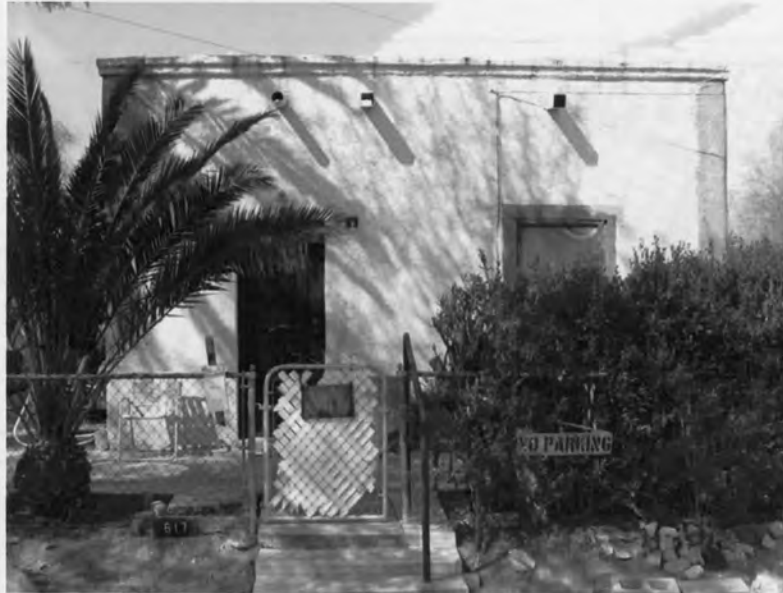
Photograph 1. 617 N. Brady Ave.; view west-southwest.
