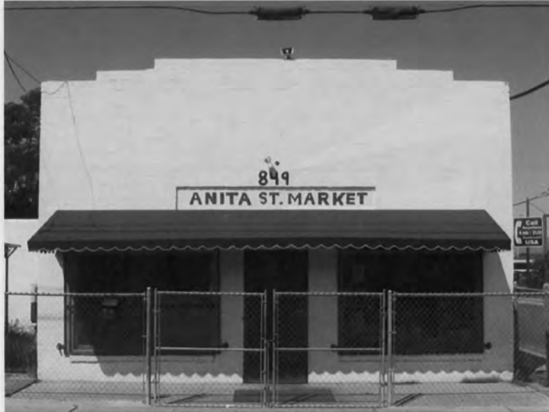
Photograph 7. Anita St. Market, 849 N. Anita Ave.; view west-southwest.
