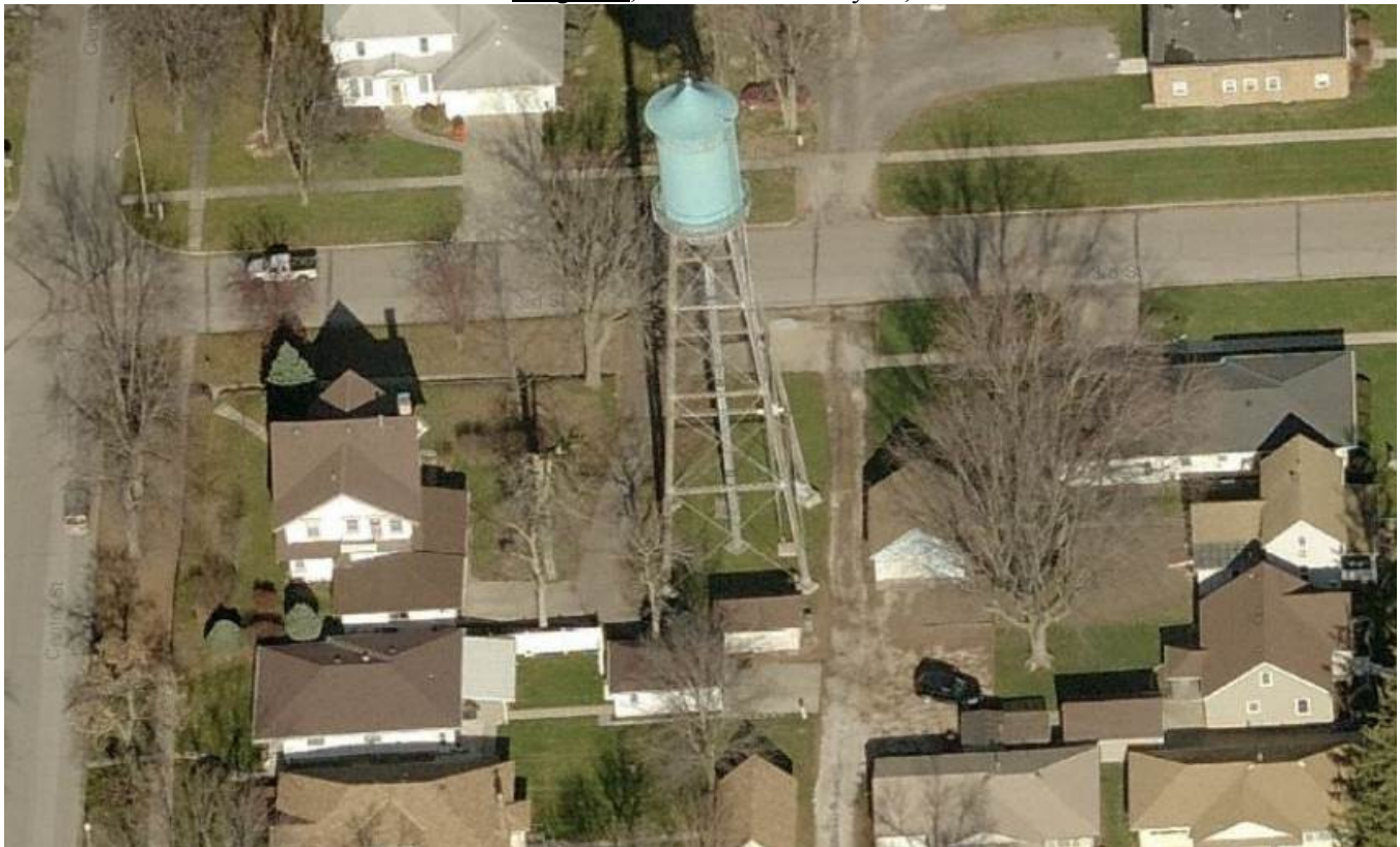
Bird's-Eye Aerial Photograph of the Manning Water Tower looking to the North. Source: Bing.com , accessed February 10, 2012.
