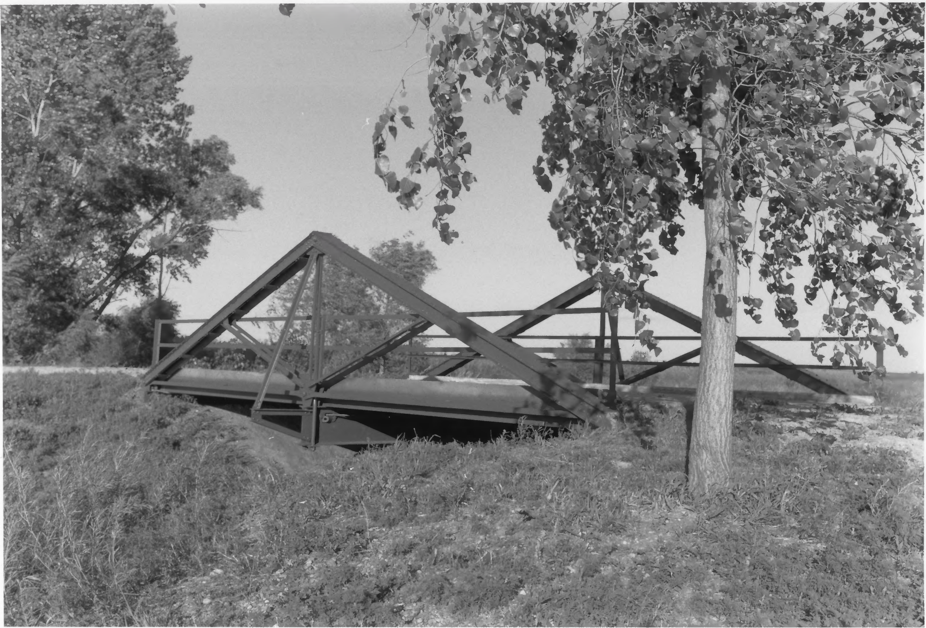
BRIDGE 1482 LIVERNE TOWNSHIP, ROCK COUNTY, MINNESOTA #011015-19
