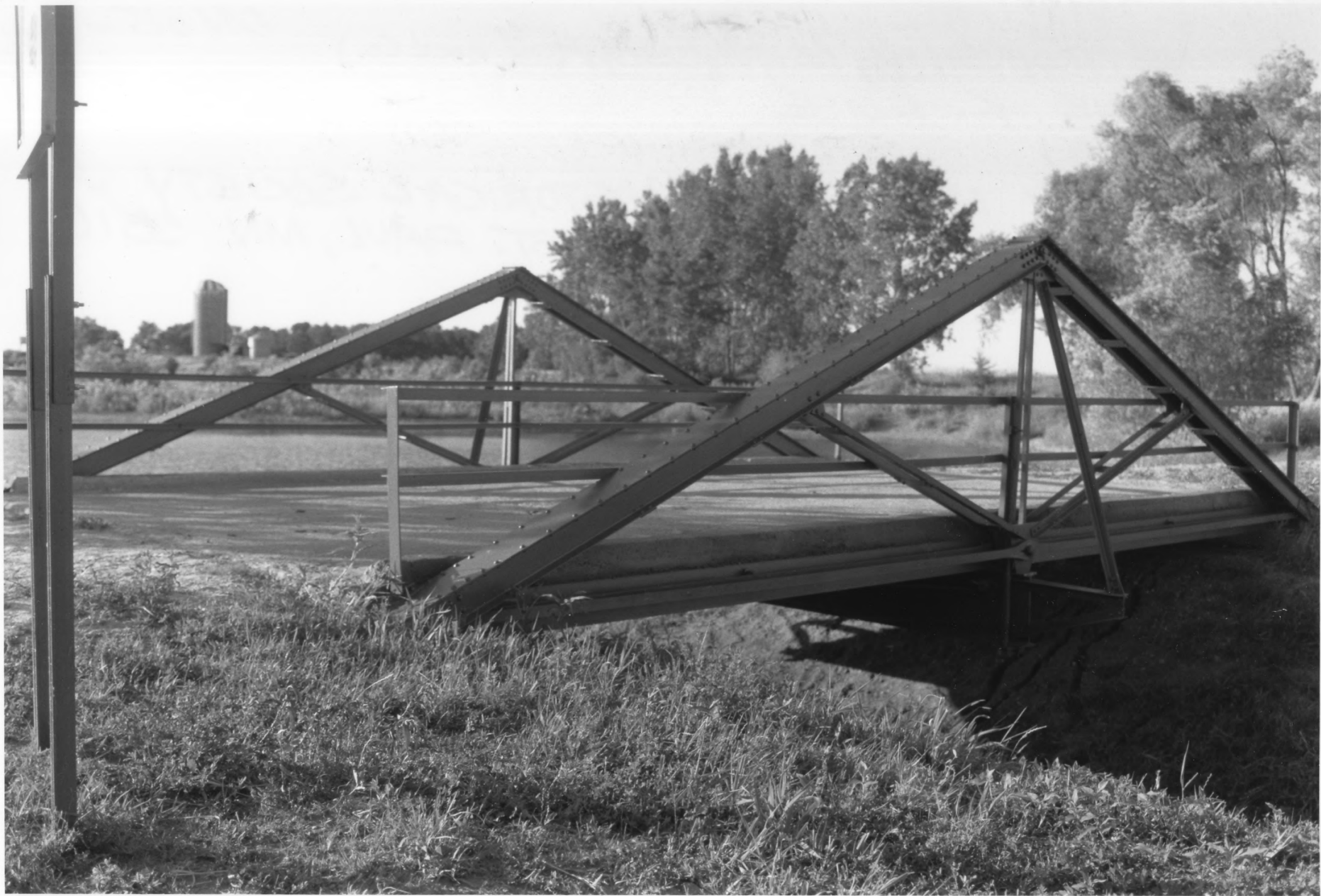
BRIDGE 1482 LUVERVE TOWNSHIP, ROCK COUNTY, MINNESOTA # 011015-20
