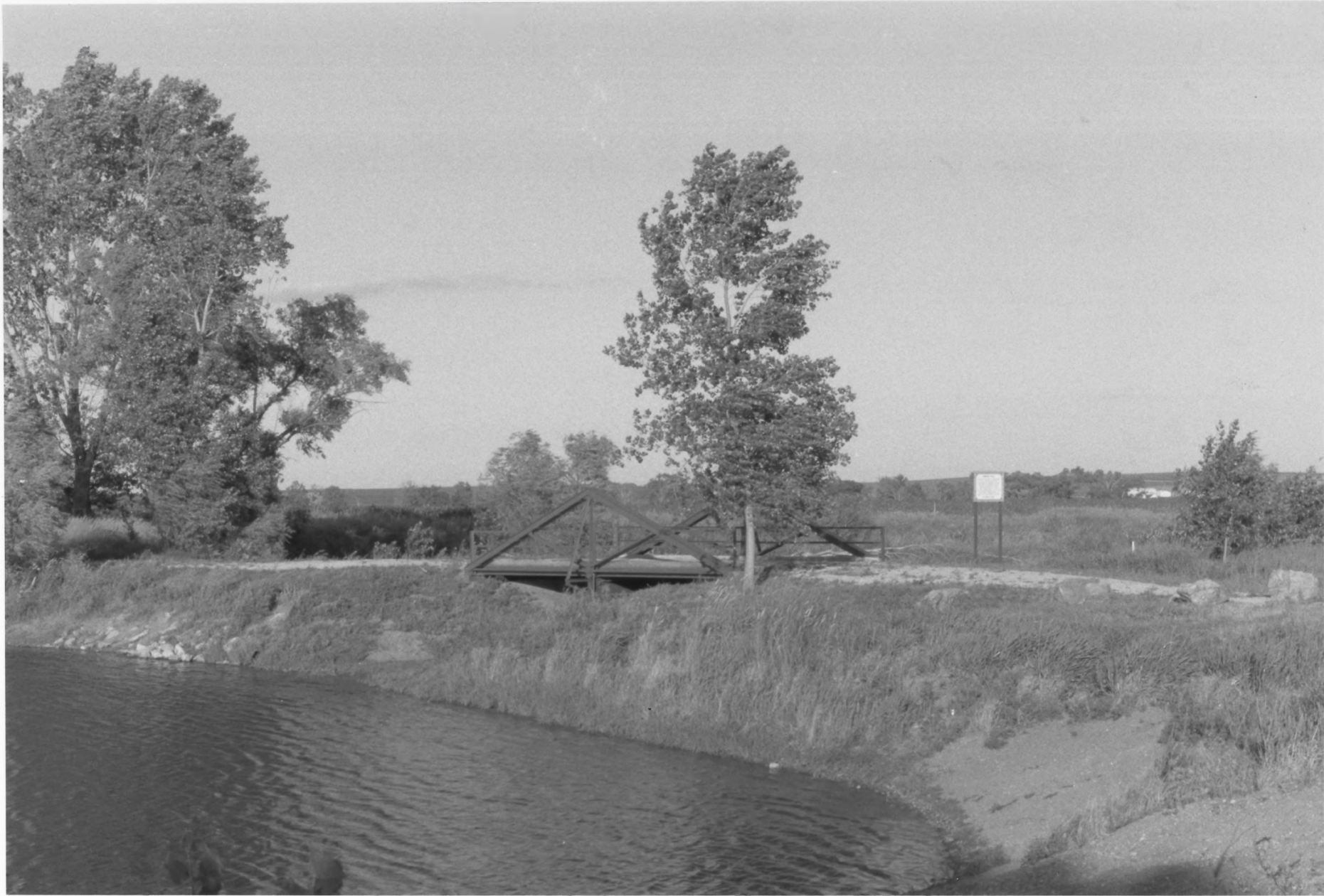
BRIDGE 1482 LVERNE TOWNSHIP, ROCK COUNTY, MINNESOTA #011015-23
