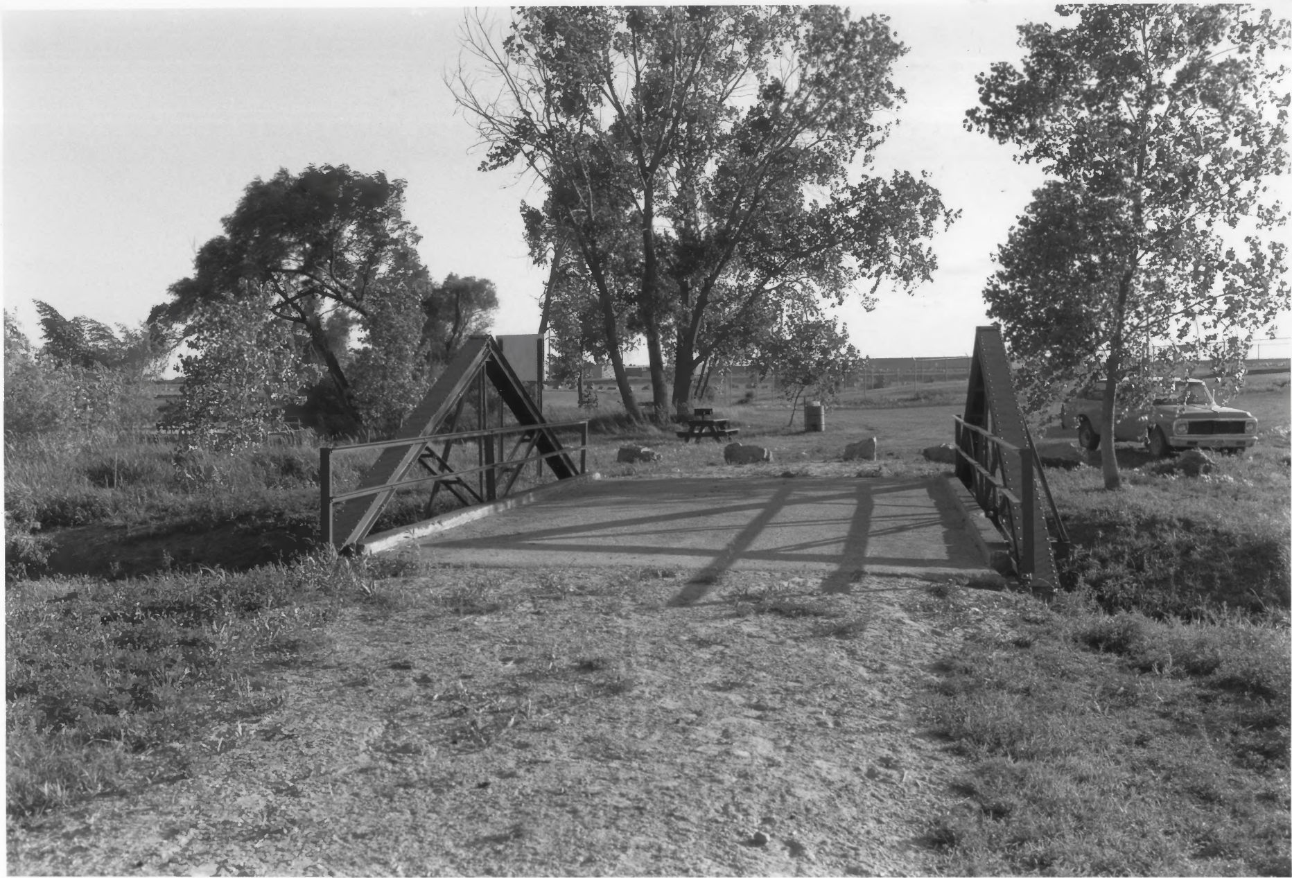
BRIDGE 1482 LIVERNE TOWNSHIP, ROCK COUNTY, MINNESOTA #011015-16
