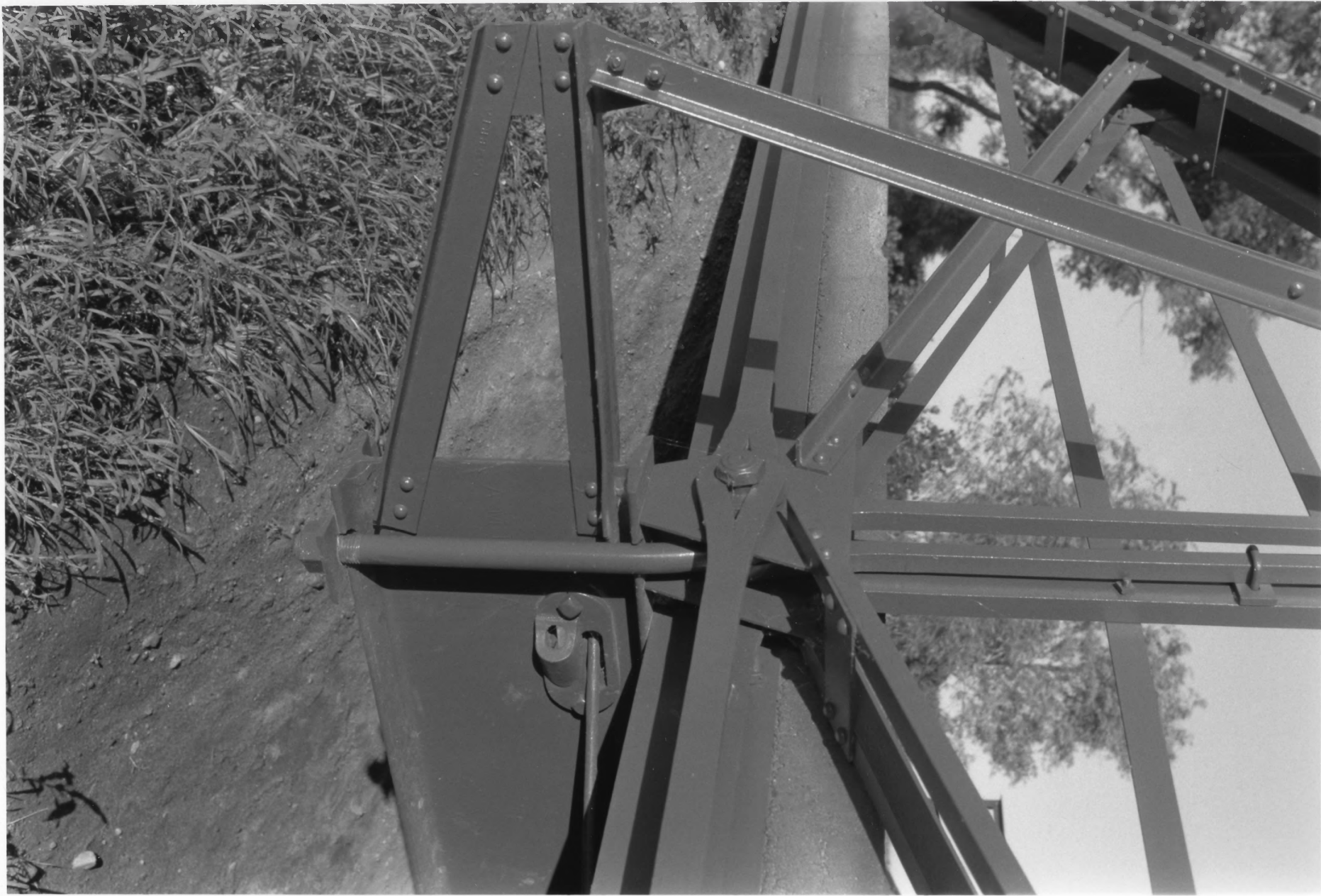
BRIDGE 1482 LIVERNE TOWNSHIP, ROCK COUNTY, MINNESOTA #011015-18
