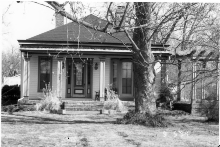
Oakland-Freepport Historic District Warren Co. Ky ⑧
