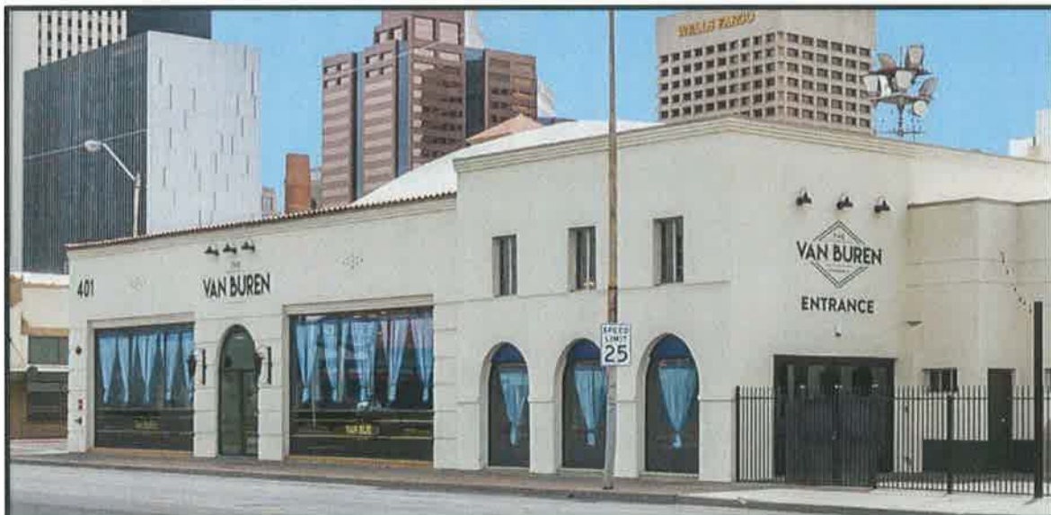
Figure 15. Facing southeast. Photograph by Elena Leon-Seefeld.
