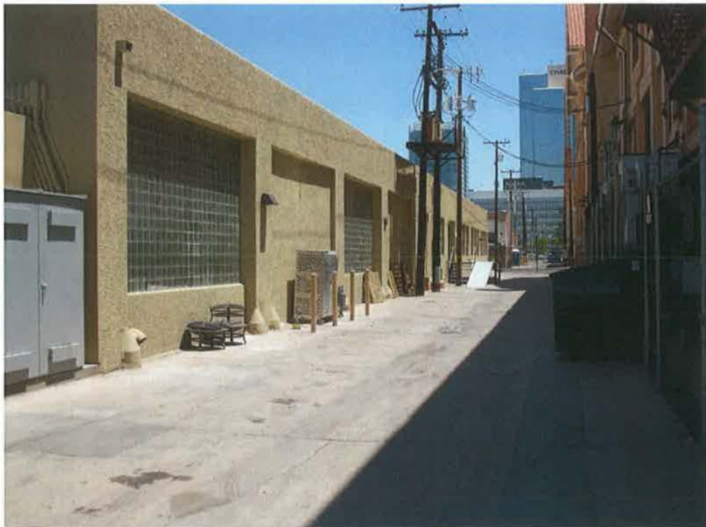
Photograph 1. Alley and rear façade. Facing east.
