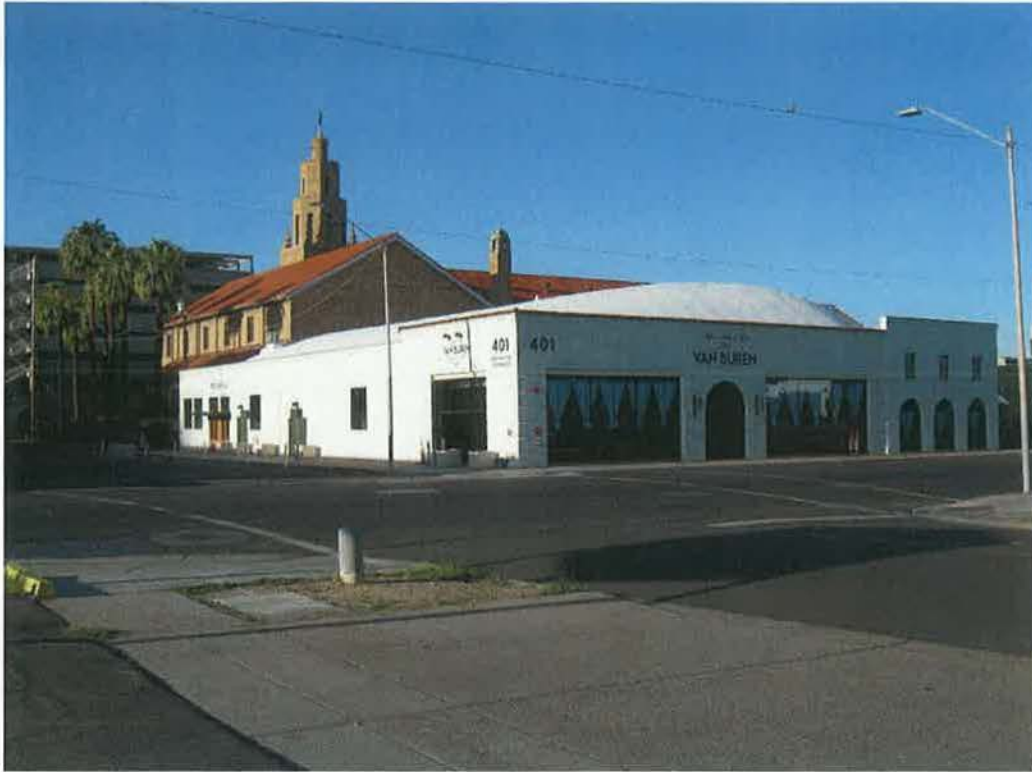
Photograph 5. Front façade. Facing south.
