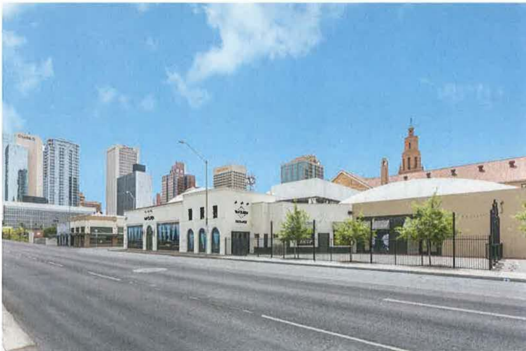
Photograph 4. Front façade and inside lot. Facing southeast.
