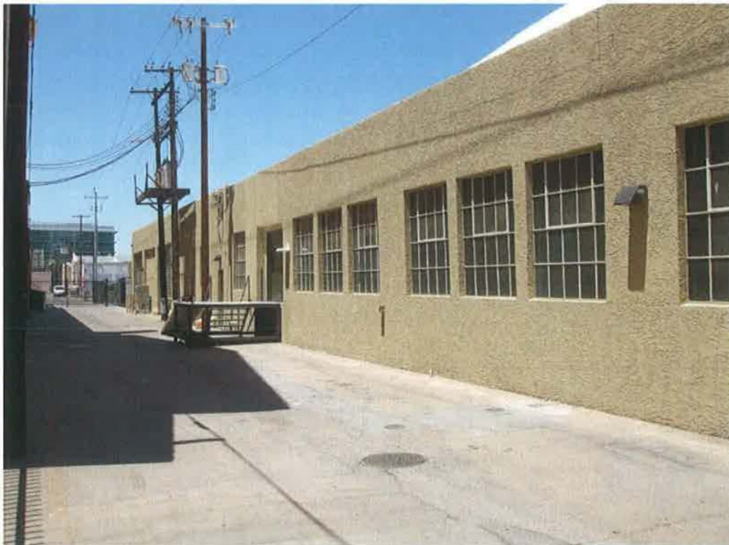
Photograph 8. Alley and rear façade. Facing west.
