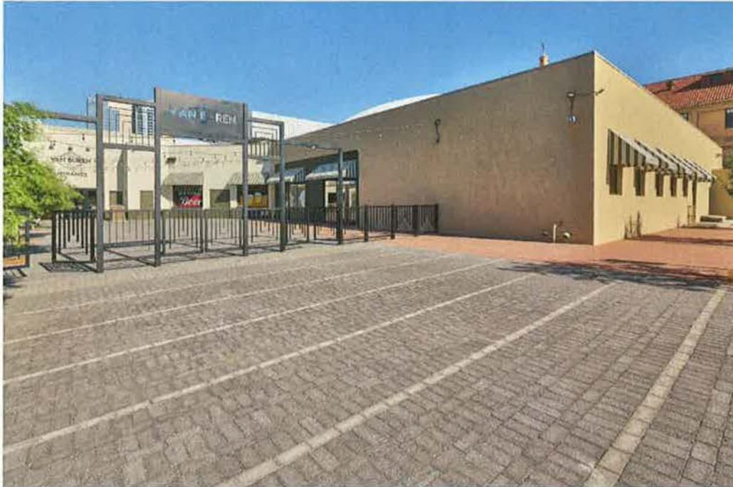
Photograph 3. Addition front façade and inside lot. Facing southeast.
