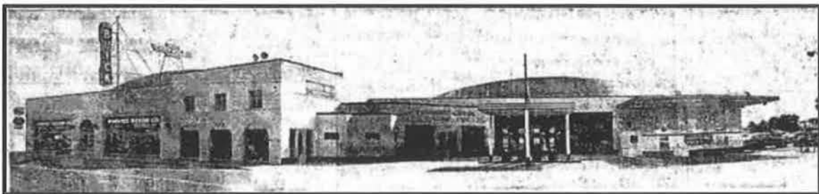
Figure 17. A panoramic rendition of the new home of Phoenix Motor Company. Arizona Republic , 16 December 1939.
