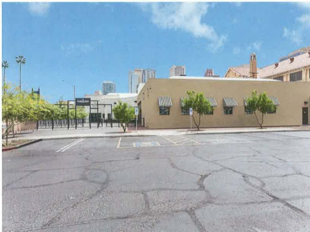
Photograph 2. East façade of addition and inside lot. Facing east.
