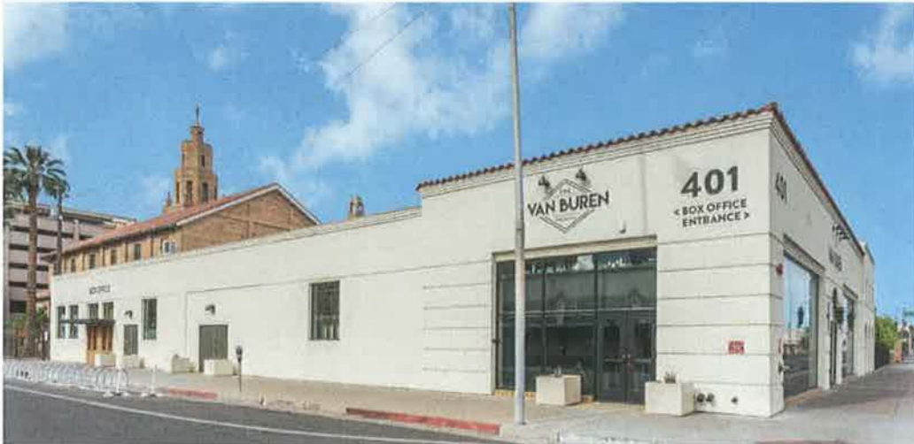
Photograph 6. East façade. Facing west.
