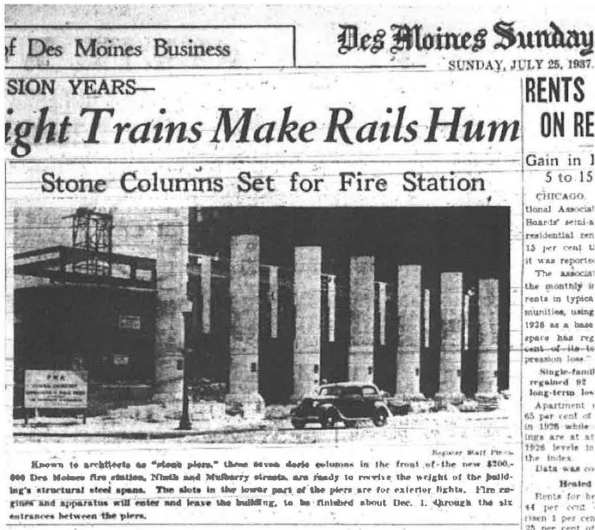
Figure 15. HISTORIC IMAGE – Fire station, July 1937
