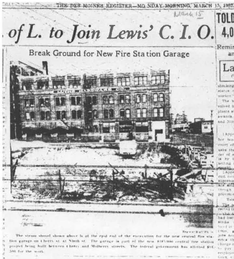
Figure 12. HISTORIC IMAGE – Shop Building excavation, March 1937
