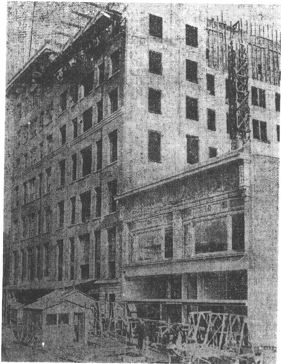
PERKINS BUILDING, 1101 A STREET, TACOMA, WA. Historic Photo, 1910, Progress photo of Perkins Annex. Tacoma Public Library, Northwest Room Collection
