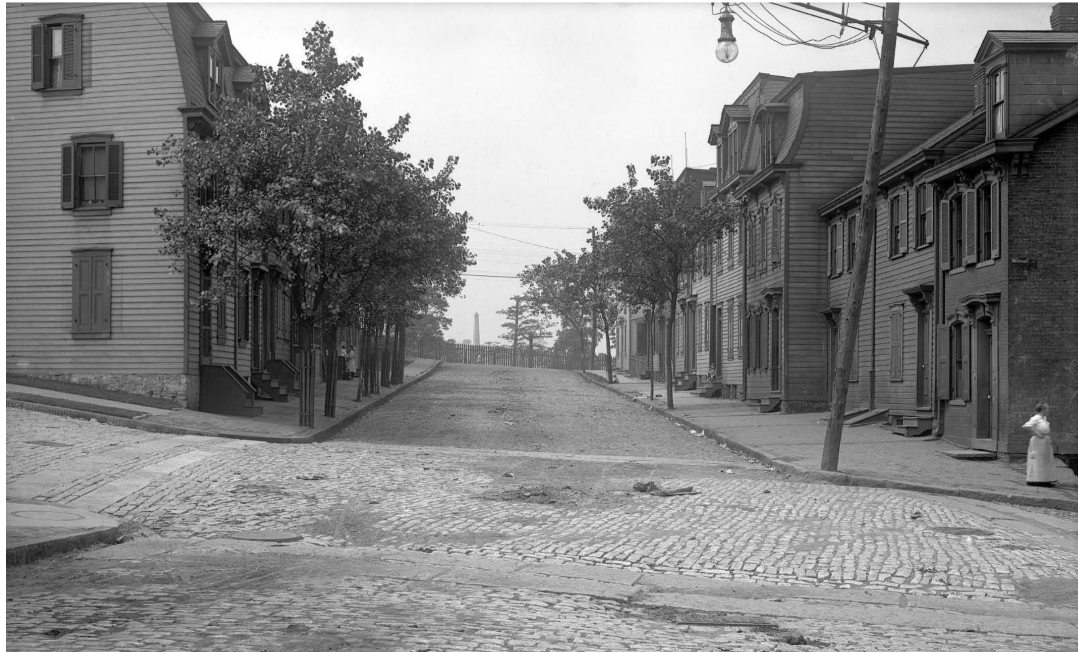
Figure 18: Duncan Street between 52 nd Street and Stanton Avenue, in what had been part of the Mowry property, in 1910. Allegheny Cemetery is across Stanton Avenue, just past the wood fence. City Photographer's Collection, University of Pittsburgh.
