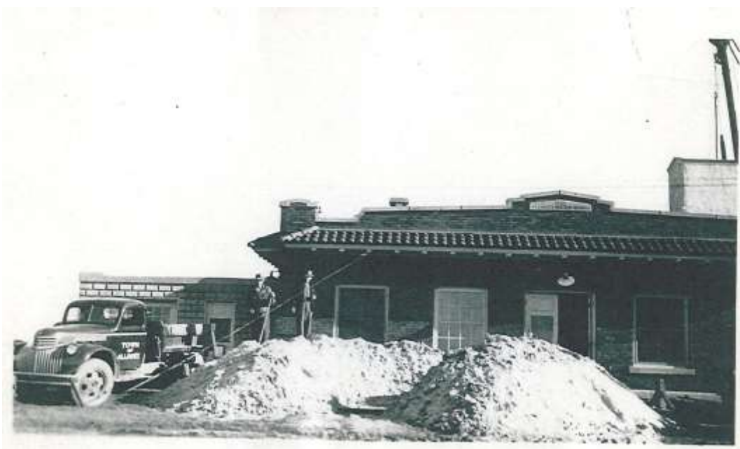
Allouez Pump House, c. 1950. Photograph courtesy of the Village of Allouez records.
