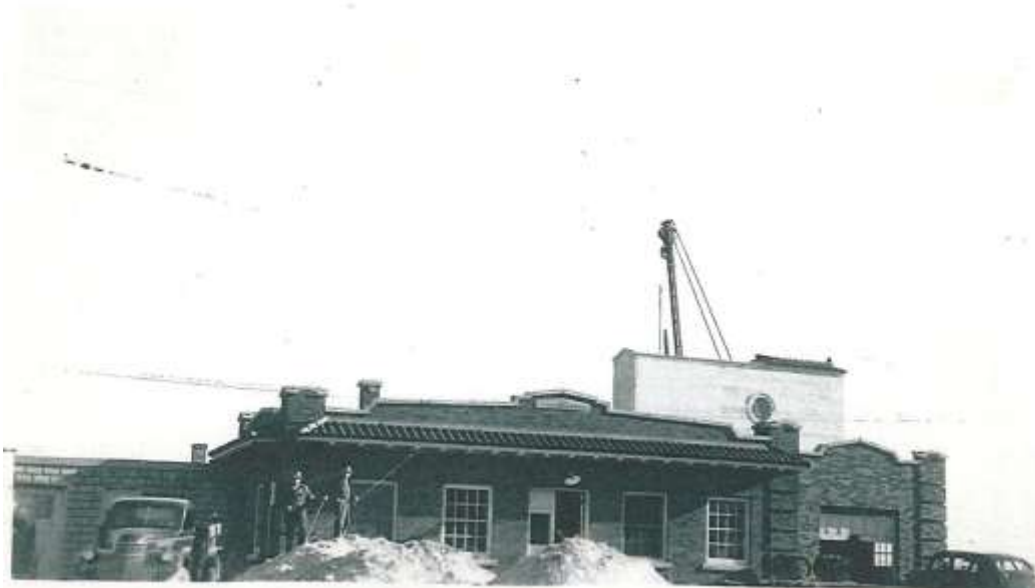
Allouez Pump House, c. 1950. Photograph courtesy of the Village of Allouez records.
