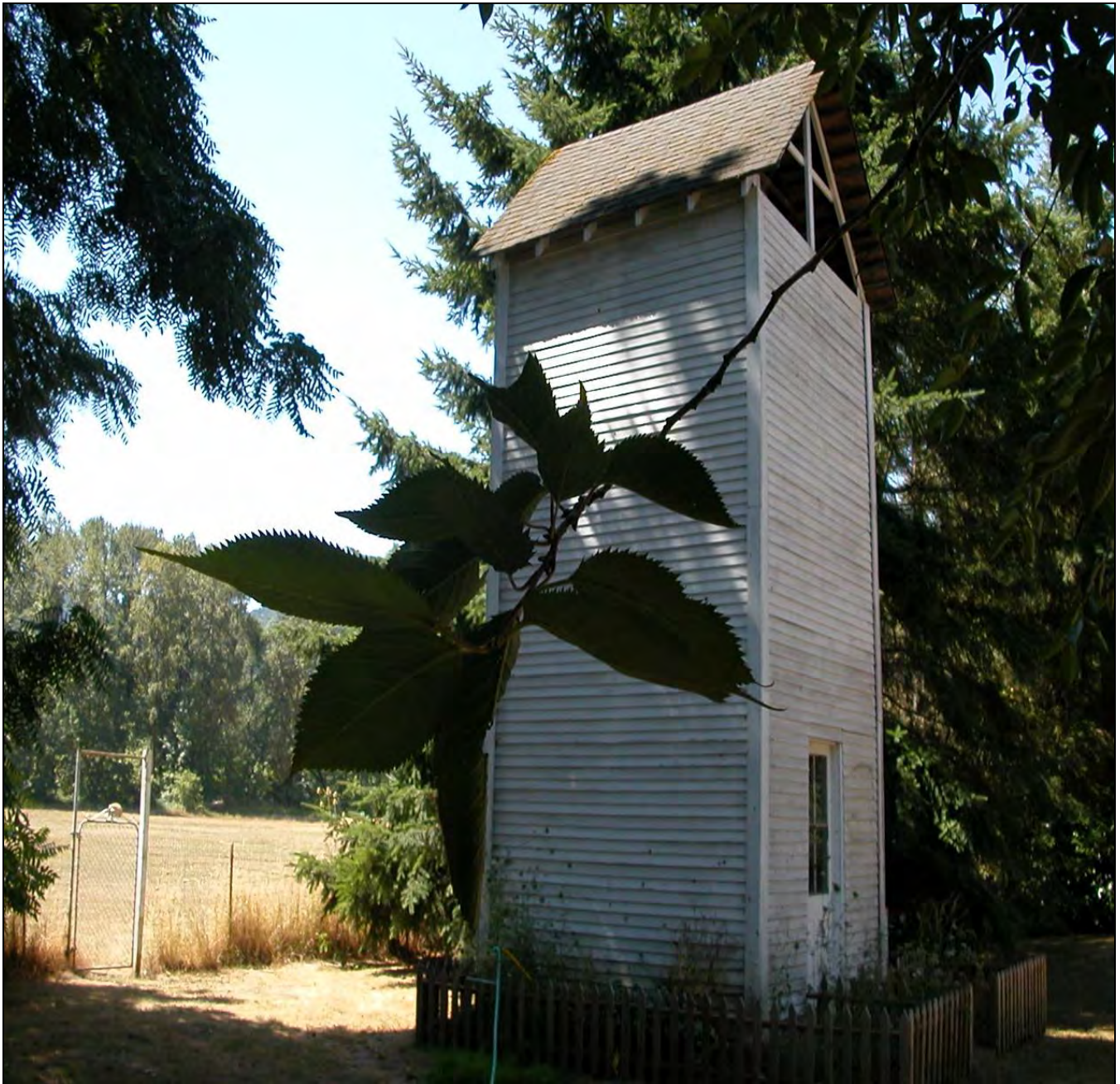
Photo 19 of 20: Site, camera facing west, east façade of water tower
