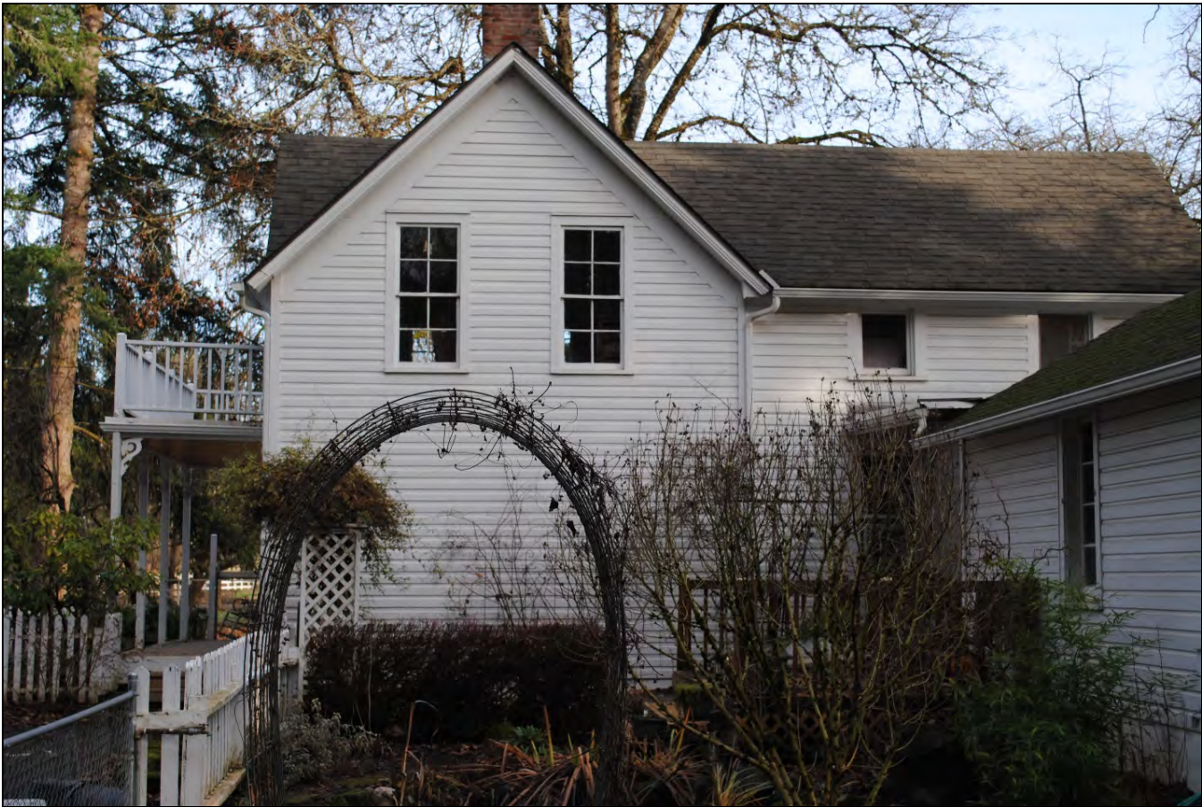
Photo 4 of 20: Farmhouse west façade, camera facing east
