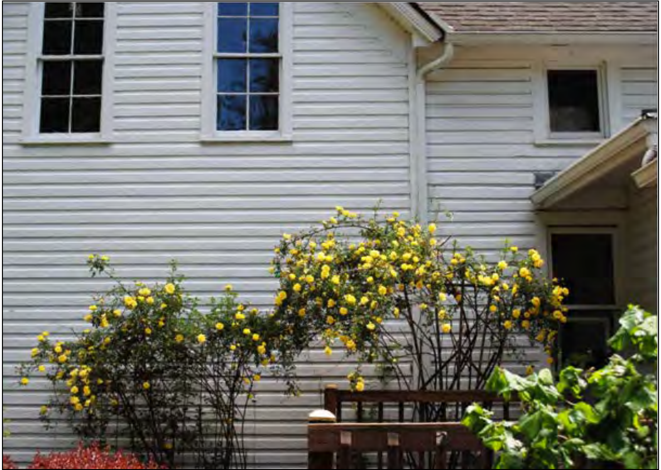
Photo 5 of 20: Farmhouse west façade, camera facing east
