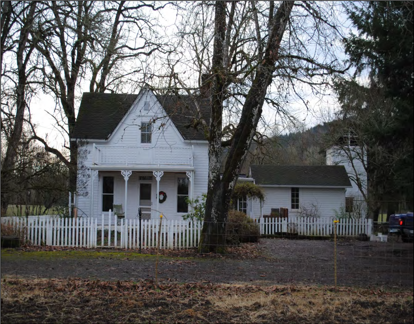
Photo 1 of 20: Farmhouse north façade, camera facing south
