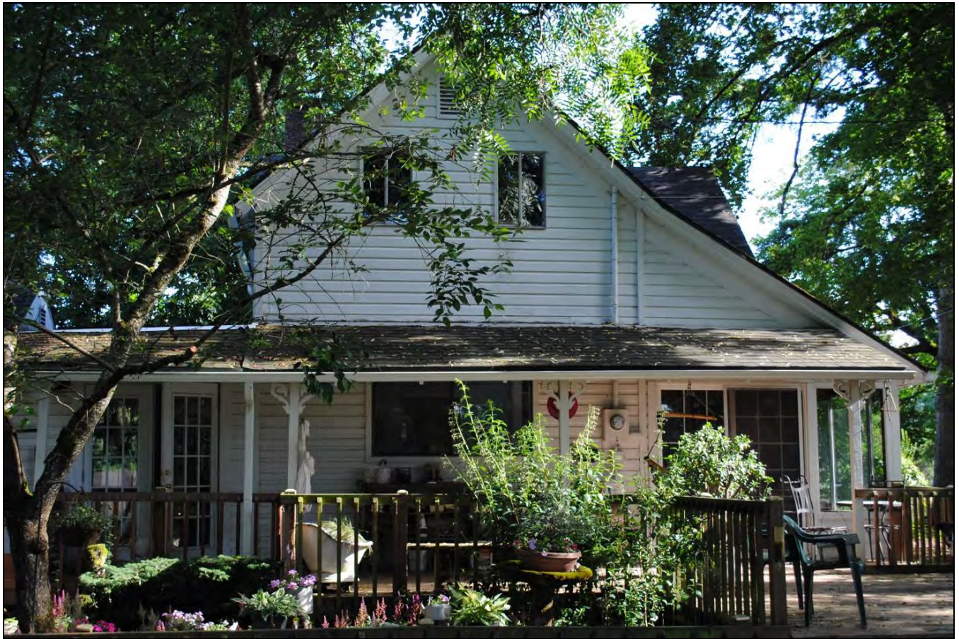
Photo 18 of 20: Farmhouse south façade, camera facing north
