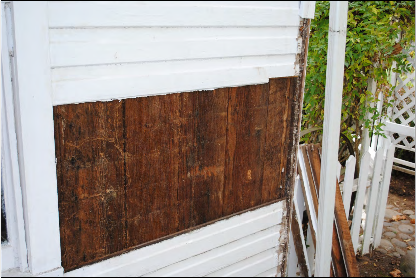
Photo 17 of 20: Farmhouse north exterior wall, exposed construction, camera facing south
