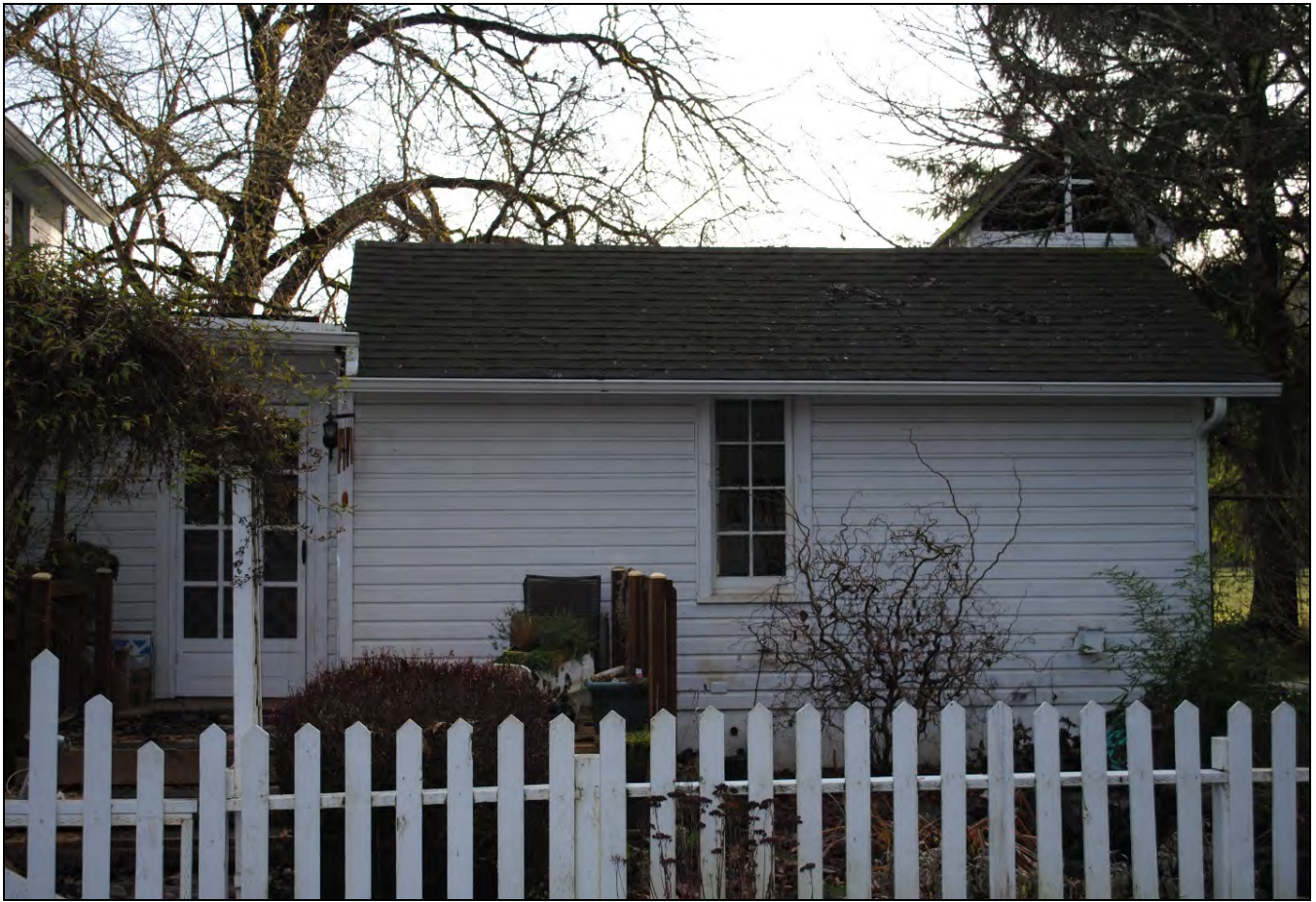
Photo 2 of 20: Farmhouse north façade, east end, camera facing south
