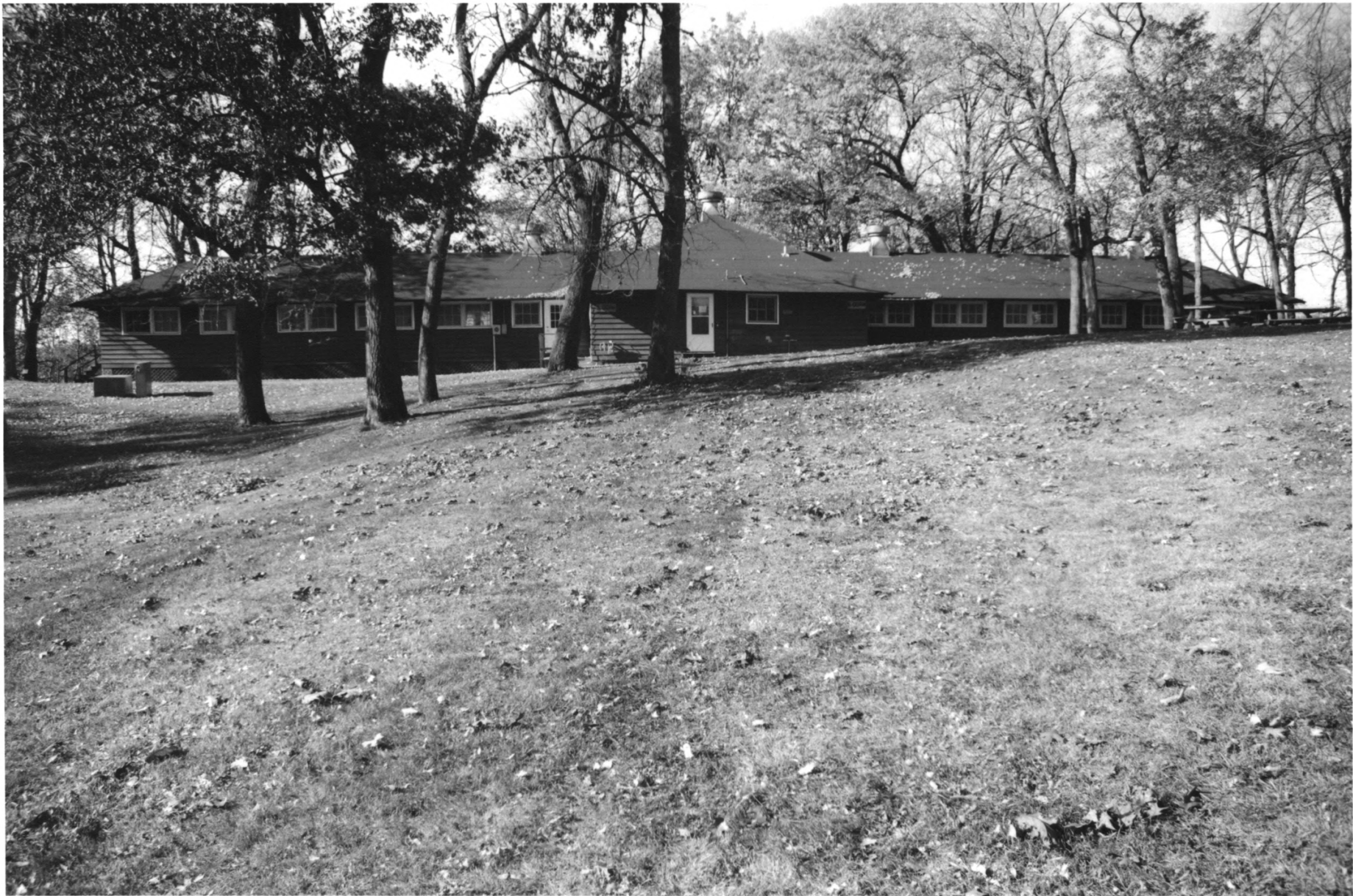
GLEN LAKE CHILDREN'S CAMP (DORMITORY)
