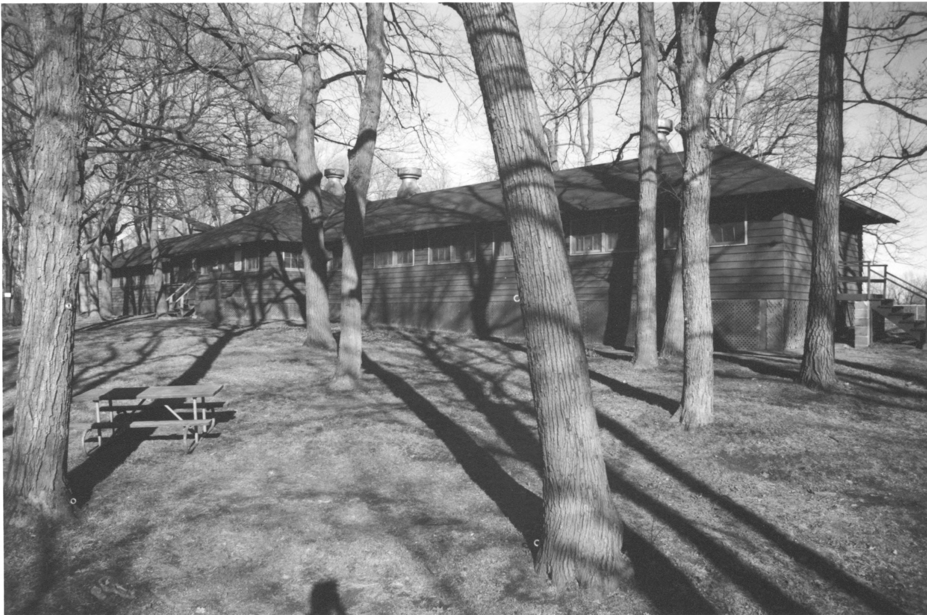
GLEN LAKE CHILDREN'S CAMP (DORMITORY)
