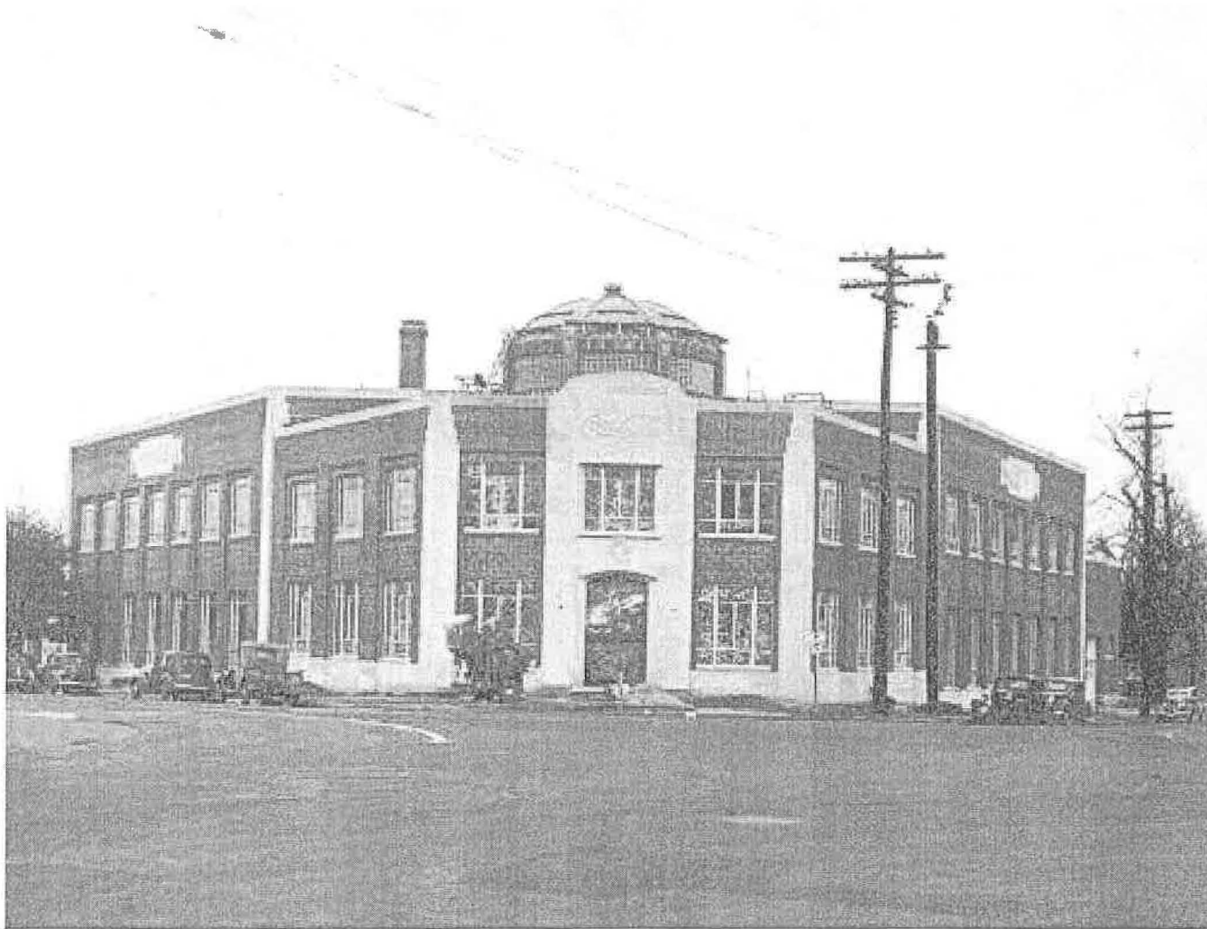
Figure 9- 3121 Broadway- Under Construction
