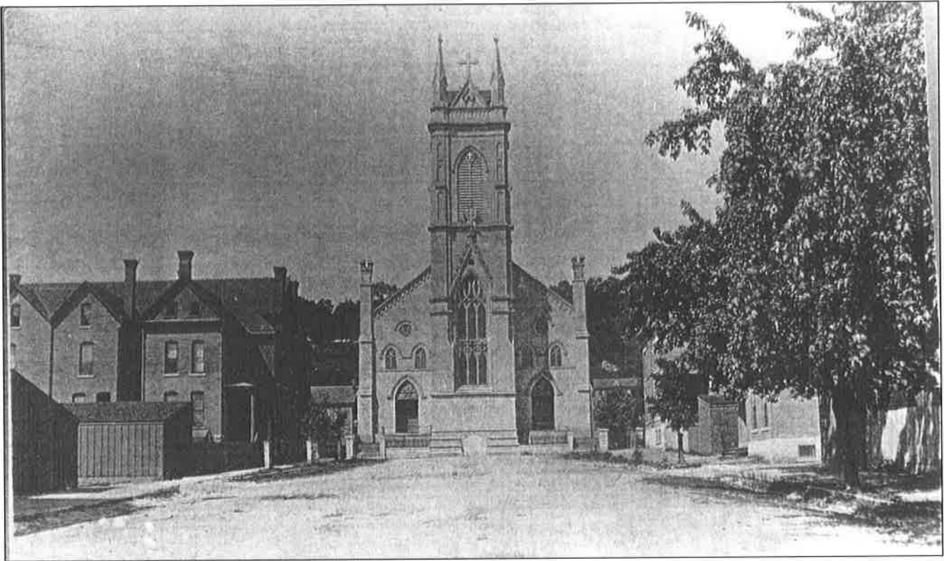
Figure 16. West Second Street terminus and St. Raphael Cathedral, c.1886 (Photo 1139, Center For Dubuque History, Loras College)
