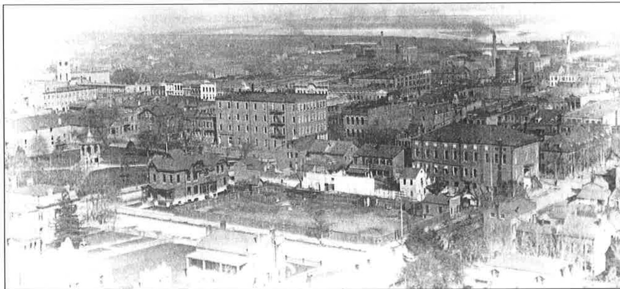
Figure 13. 400s-500s block of Bluff Street, c.1884-85 (Photo KRE 124, Center For Dubuque History, Loras College)
