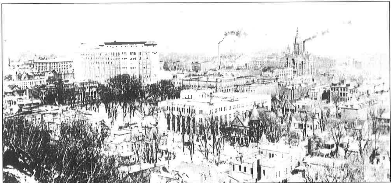
Figure 35. 400s-500s blocks of Bluff, view northeast, c.1940 (John Vachon?) (Photo LS 670, Center For Dubuque History, Loras College)
