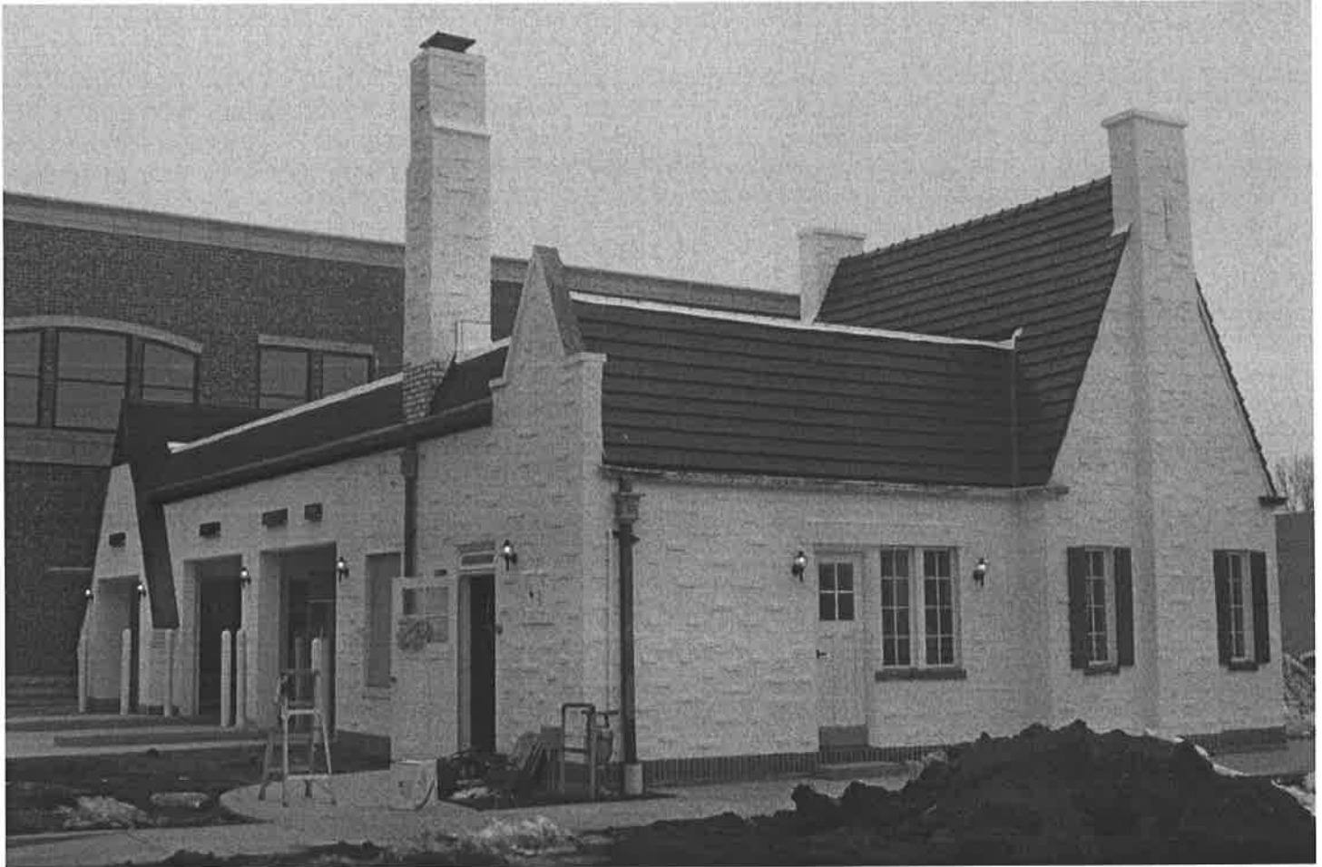
Pure Oil Station, with non historic addition removed. 502 W. State Street, Geneva, Illinois Kane County
